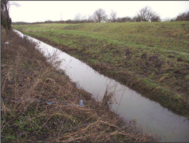
Plate 1: General shot of the Car Dyke, showing the end of the drainage trench marked out in blue, looking northwest
