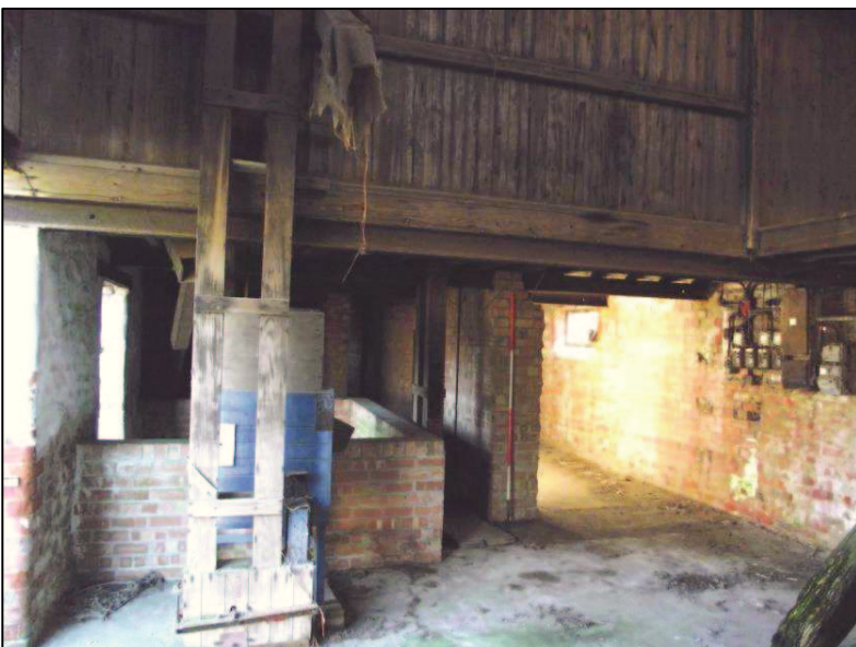
Plate 27 (Shot 29): Interior view of B4, looking southeast. Scale is 2m
