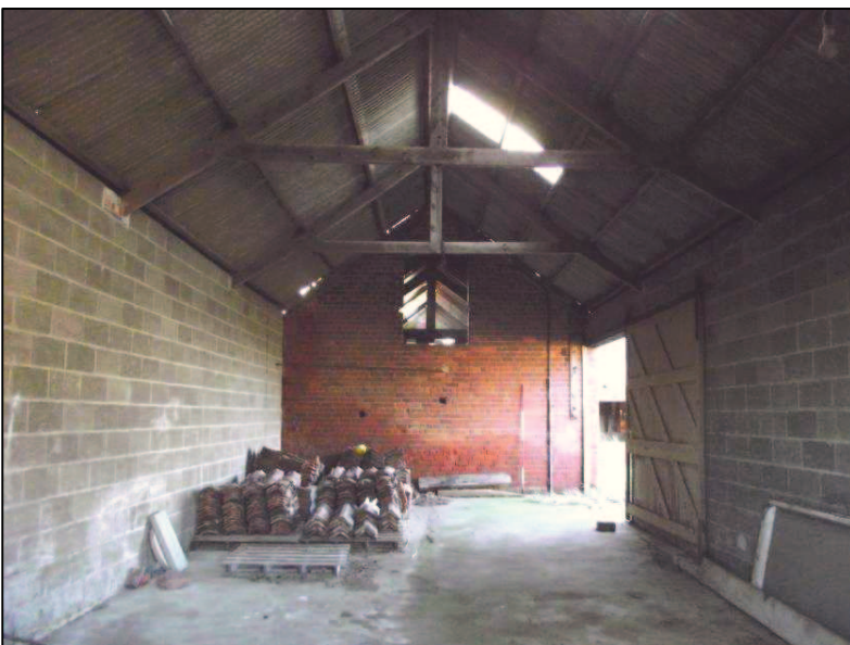
Plate 33 (Shot 39): Interior view of B5.2, looking south-southwest. Scale is 2m
