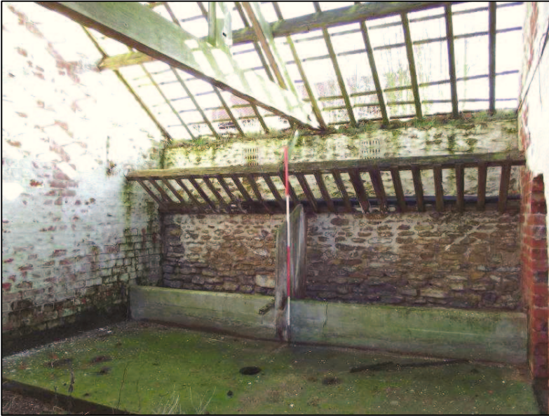
Plate 10 (Shot 12): Interior view of B1.6, looking east. Scale is 2m
