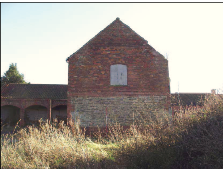
Plate 24 (Shot 27): Northwest elevation of B4, looking northeast. Scale is 2m
