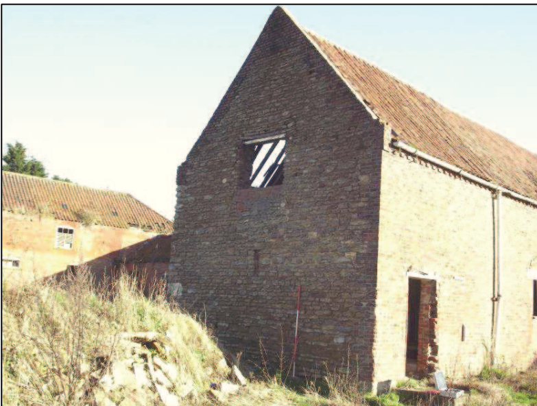
Plate 12 (Shot 17): Northwest elevation of B2, looking northeast. Scale is 2m.
