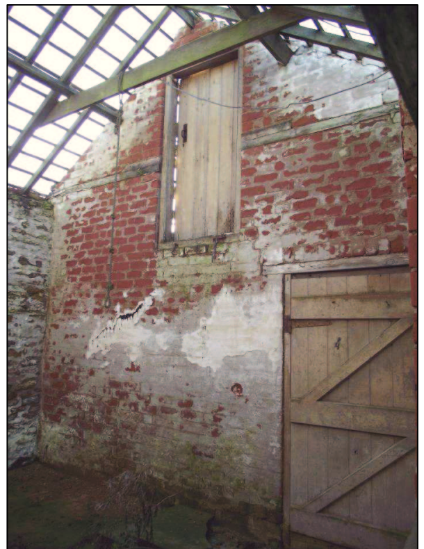
Plate 6 (Shot 6): Northeast elevation of Barn 1.2, looking southeast
