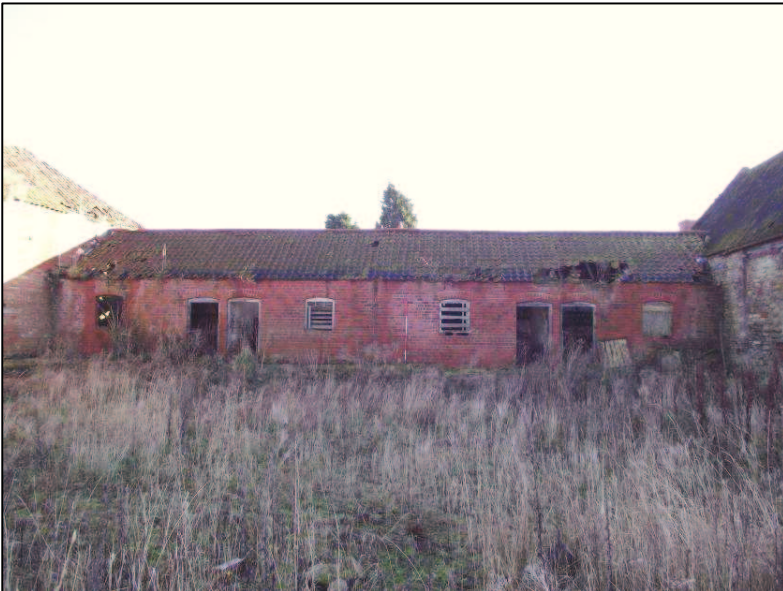
Plate 17 (Shot 20): Northwest elevation of B3, looking east-southeast. Scale is 2m
