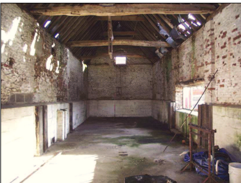
Plate 15 (Shot 14): Interior view of B2, looking east-southeast. Scale is 2m
