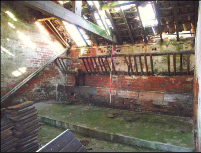
Plate 22 (Shot 25): Interior view of B3.4, looking east. Scale is 2m
