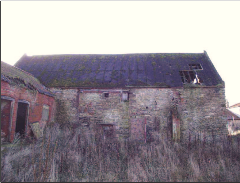
Plate 13 (Shot 19): Northeast elevation of B2, looking southwest. Scale is 2m
