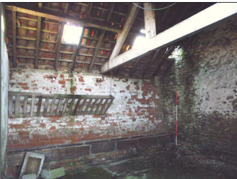
Plate 18 (Shot 21): Interior view of B3.1, looking southeast. Scale is 2m
