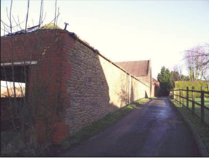
Plate 1 (Shot 2): Southeast elevation of B1, looking north. Scale is 2m
