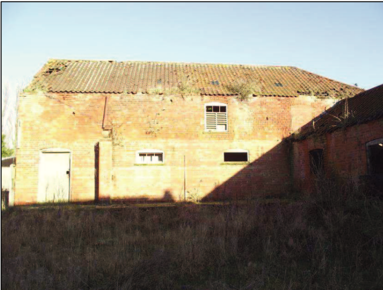
Plate 23 (Shot 26): Southwest elevation of B4, looking north-northeast. Scale is 2m
