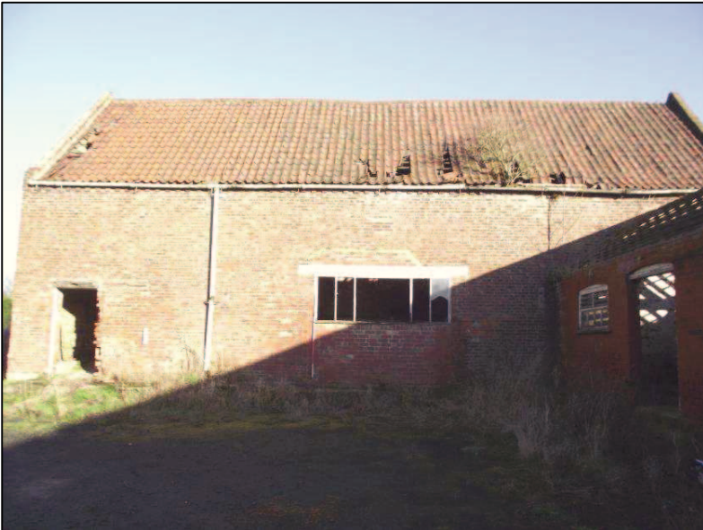
Plate 11 (Shot 13): Southwest elevation of B2, looking north-northeast. Scale is 2m
