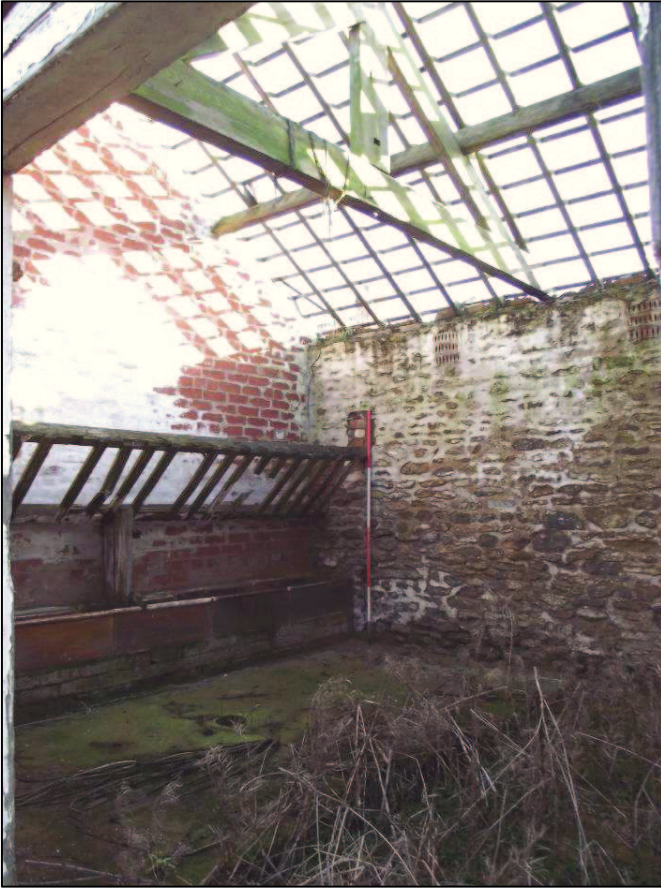
Plate 7 (Shot 9): Interior view of B1.3, looking northeast. Scale is 2m
