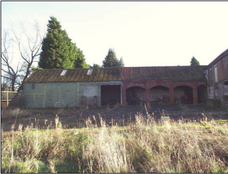
Plate 28 (Shot 34): Northwest elevation of B5, looking southeast. Scale is 2m
