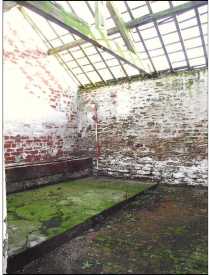
Plate 8 (Shot 10): Interior view of B1.4, looking northeast. Scale is 2m
