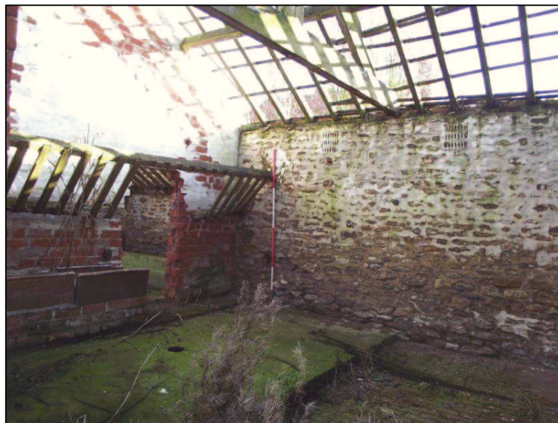
Plate 9 (Shot 11): Interior view of B1.5, looking northeast. Scale is 2m
