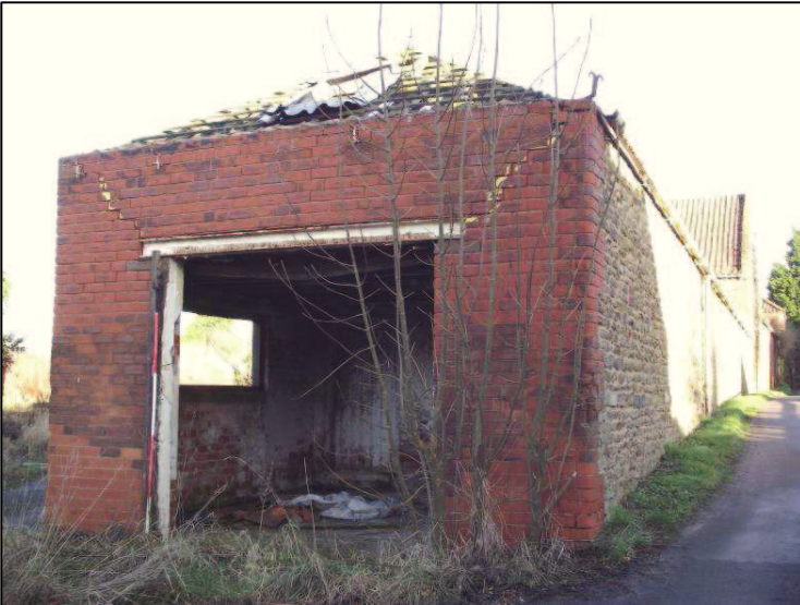
Plate 2 (Shot 3): Southwest elevation of B1, looking north. Scale is 2m
