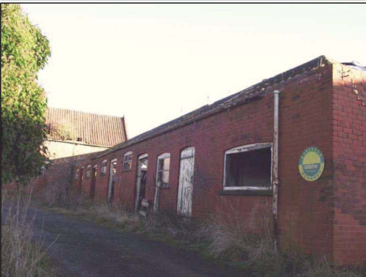
Plate 3 (Shot 4): Northwest elevation of B1, looking north-northeast. Scale is 2m
