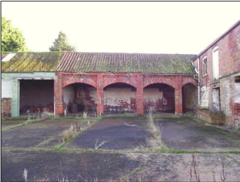
Plate 29 (Shot 35): Northwest elevation of B5.1, looking southeast. Scale is 2m
