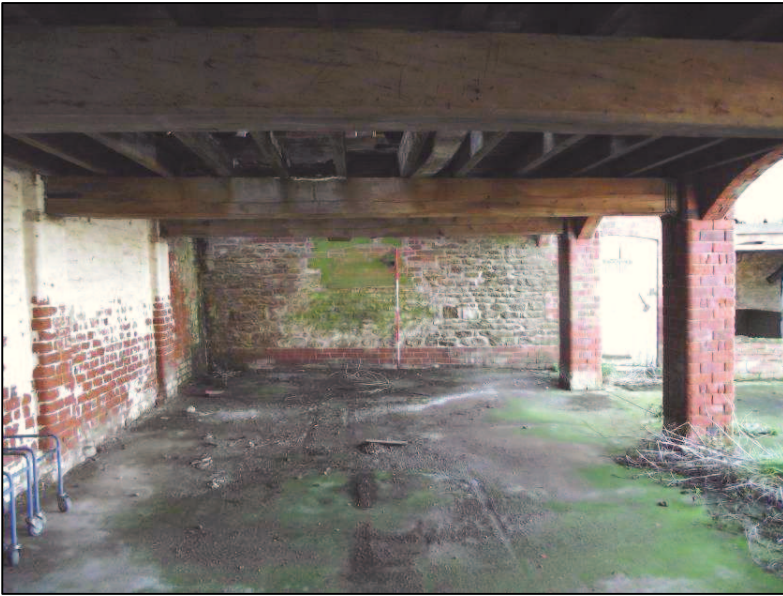
Plate 31 (Shot 36): Interior view of B5.1, looking south-southwest. Scale is 2m
