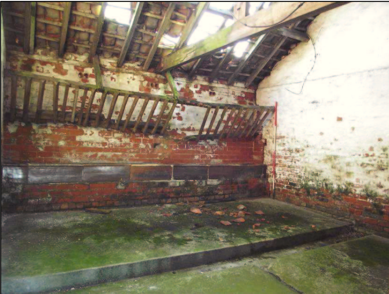
Plate 20 (Shot 23): Interior view of B3.3, looking southeast. Scale is 2m
