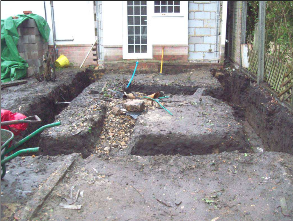
Plate 1: General view of the groundworks, looking northwest
