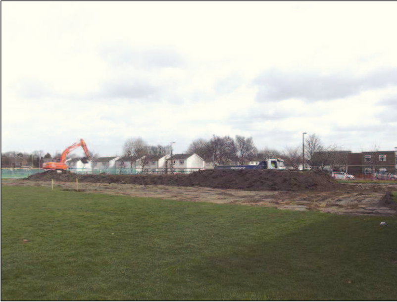
Plate 1: General view of site, looking northeast
