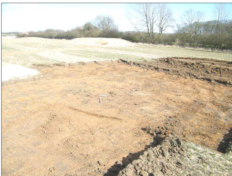
Plate 3: Stripped area of crane hardstanding, looking north-northwest. Scales are 1m
