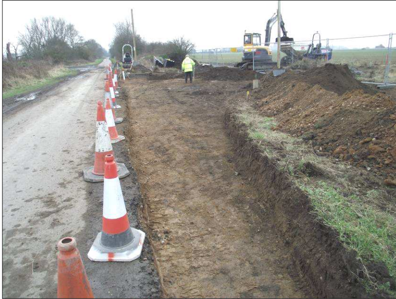
Plate 1: General view of groundworks at site entrance, looking southwest
