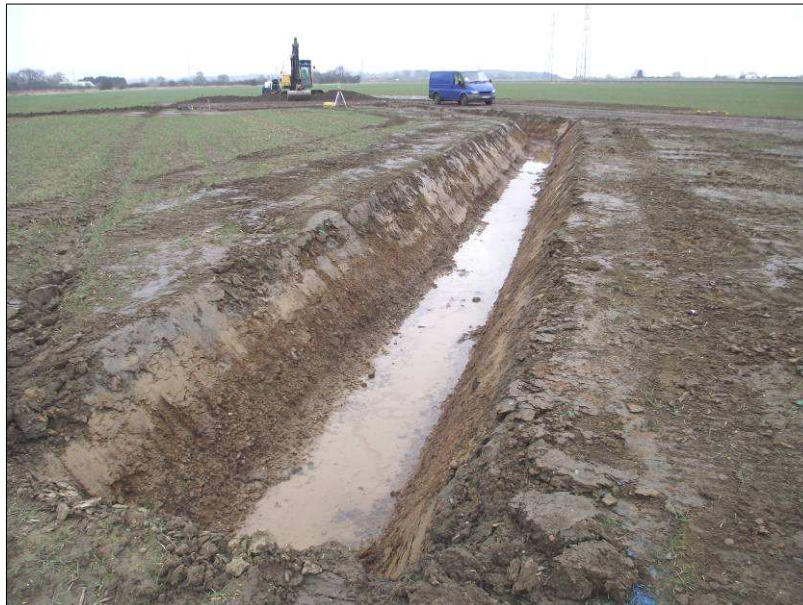
Plate 2: General view of excavated swales, looking northwest
