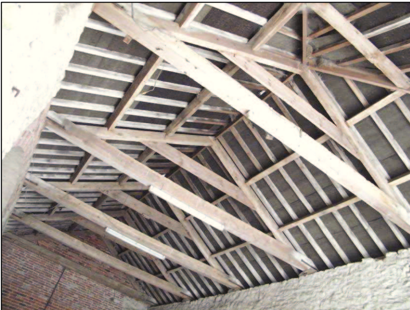
Plate 11 (Shot 20): Roof structure in the threshing barn, looking north
