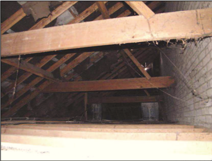
Plate 40 (Shot 72): Roof structure of Building D, looking north
