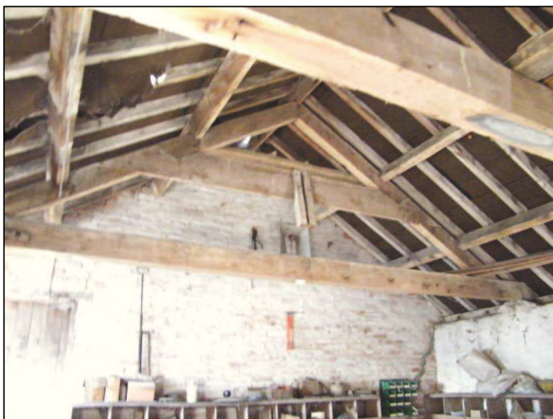
Plate 15 (Shot 26): Roof structure above the loft, looking east-southeast.
