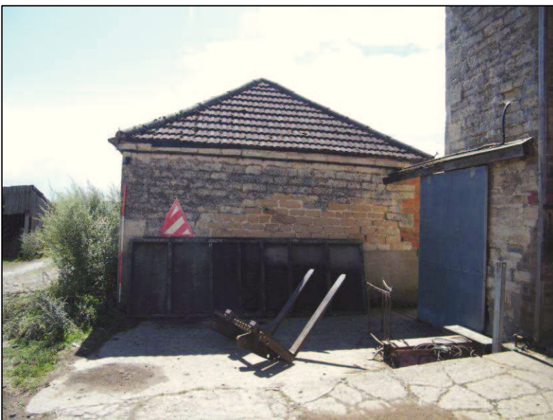
Plate 18 (Shot 35): North elevation of Building B, looking south-southwest. Scale is 2m
