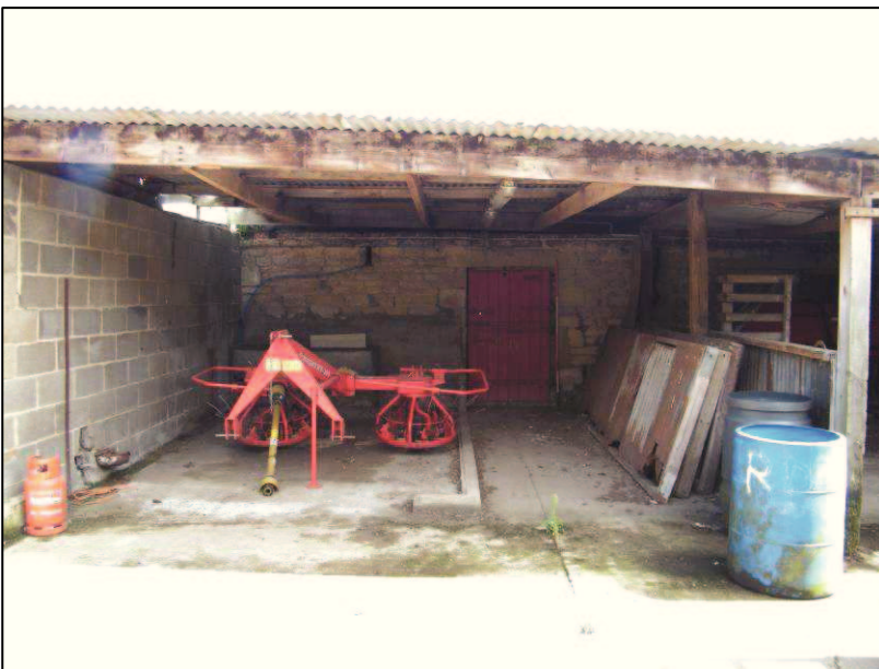
Plate 23 (Shot 43): Southern lean-to of Building B, looking east-southeast. Scale is 2m
