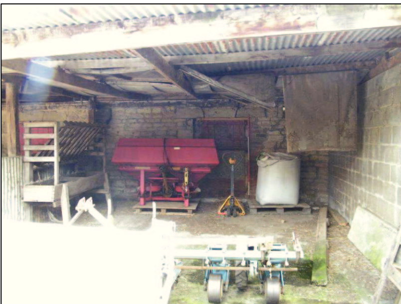
Plate 24 (Shot 45): Southern lean-to of Building B, looking east-southeast. Scale is 2m
