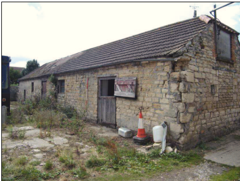
Plate 26 (Shot 48): West elevation of Building C, looking southwest. Scale is 2m
