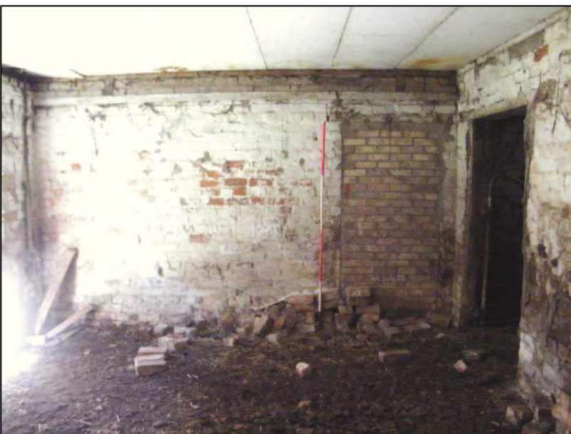
Plate 42 (Shot 75): Bricked up door in the north elevation of Building D, looking north-northeast. Scale is 2m
