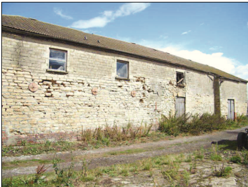
Plate 7 (Shot 11): South elevation of Building A, looking northeast. Scale is 2m
