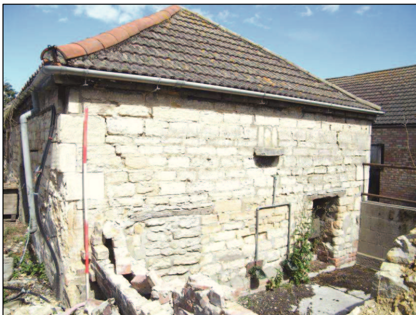
Plate 32 (Shot 60): South elevation of Building C, looking east-northeast. Scale is 2m
