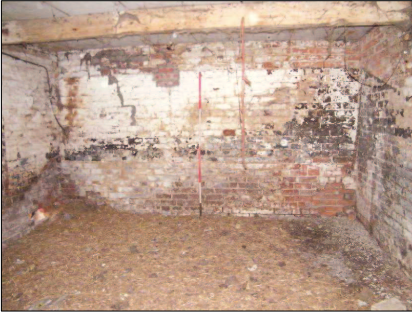
Plate 43 (Shot 78): Eastern half of northern block of Building D, looking south. Scale is 2m
