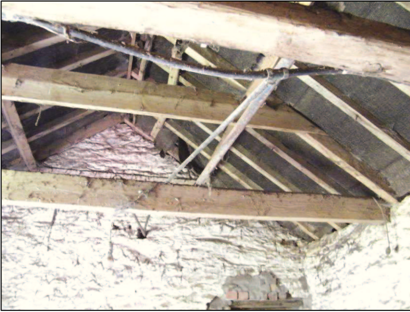
Plate 34 (Shot 63): Roof structure of southern block of Building C, looking north
