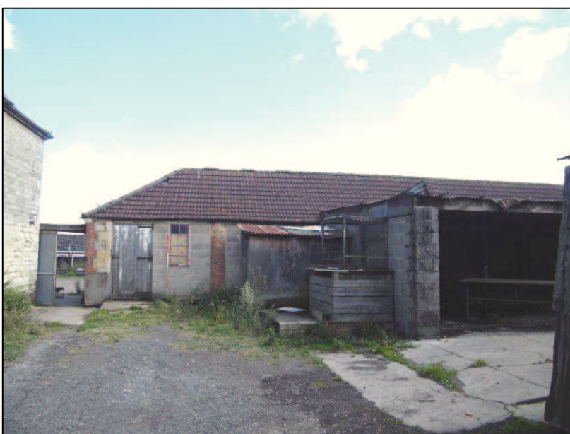
Plate 21 (Shot 40): West elevation, north end of Building B, looking east-southeast. Scale is 2m
