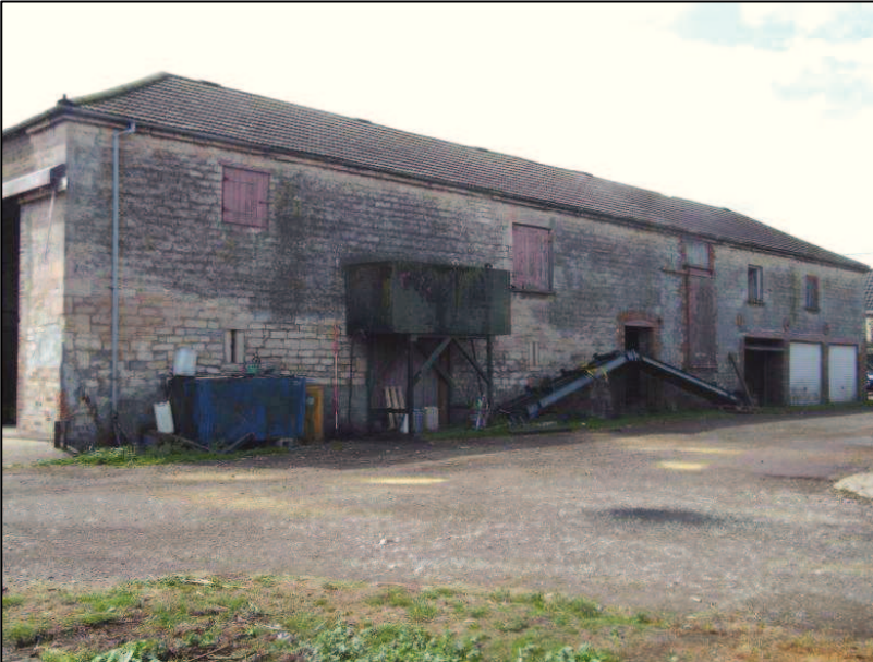
Plate 2 (Shot 2): North elevation of Building A, looking southwest. Scale is 2m
