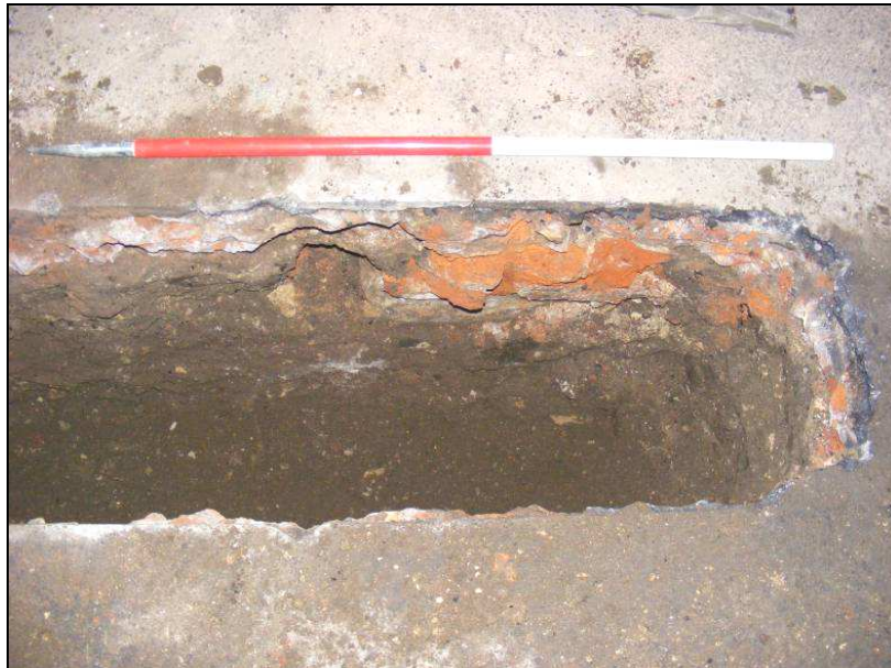
Plate 2: Wall 202 and foundation 203 at west end of Trench 2. Looking south, 1m scale
