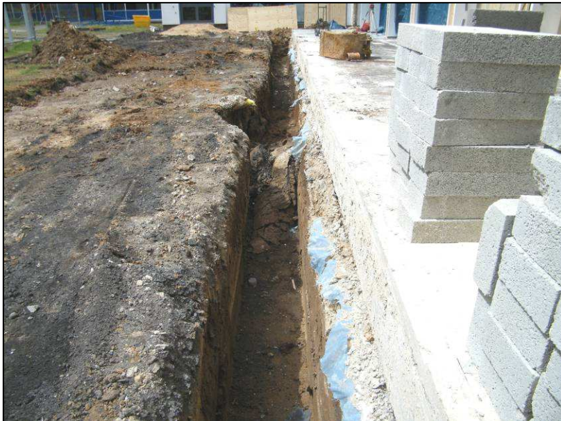
Plate 2: General shot of Area 2, looking west
