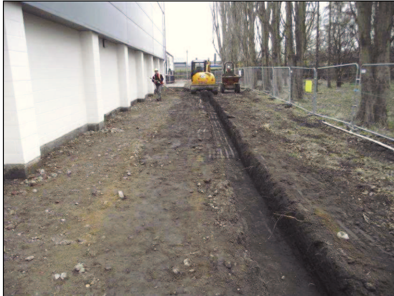
Plate 1: General view of the foundation footings, looking east-southeast
