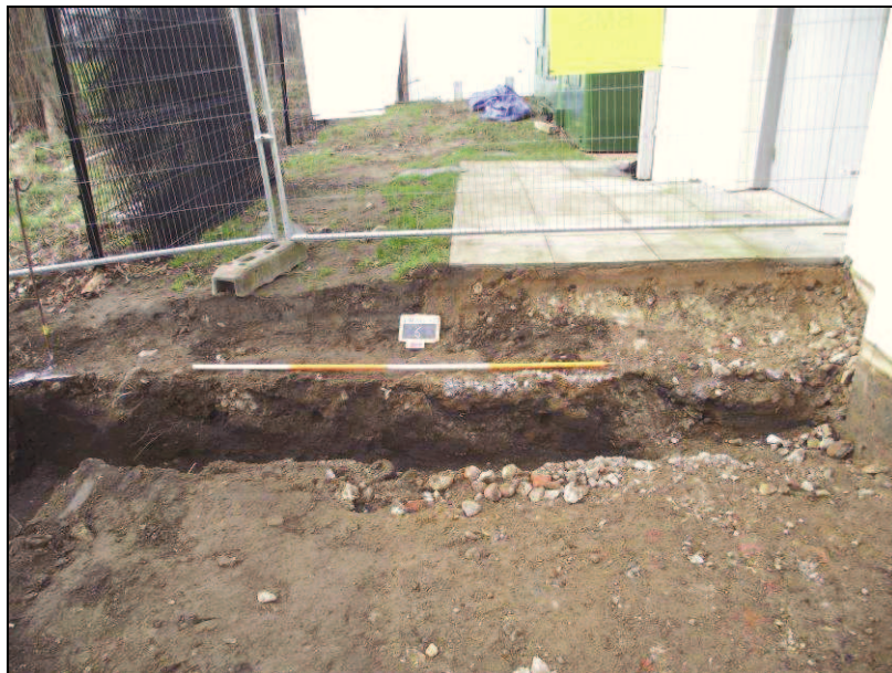
Plate 2: East facing section of foundation footings, scale is 2m
