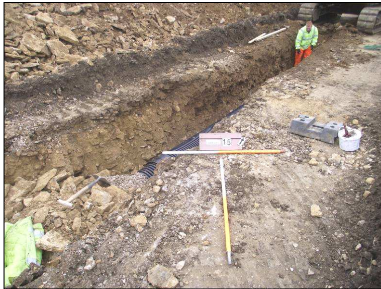
Plate 1: Northwest facing section of trench showing feature [015]. 1m and 2m scales
