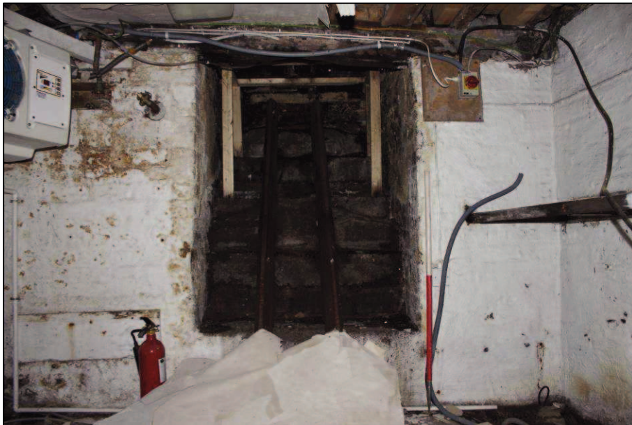
Plate 11 (Shot 46): Cellar access to Andover Road, looking east-southeast, 1m scale
