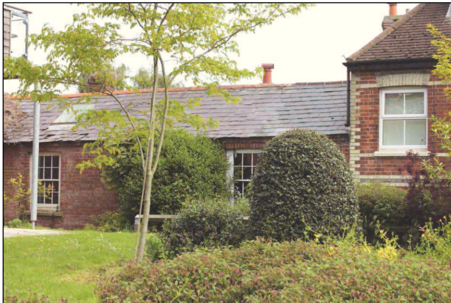
Plate 26 (Shot 121): Southwest elevation of the function room
