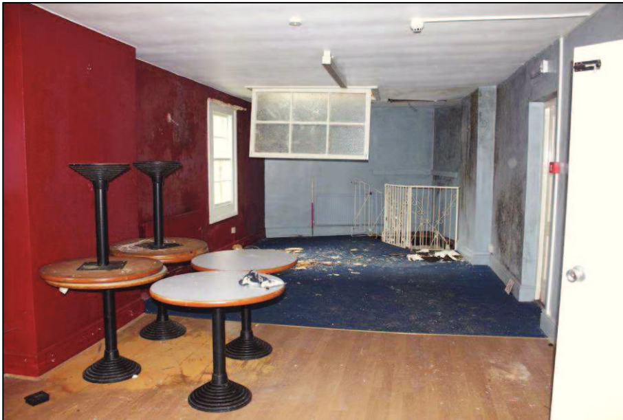
Plate 29 (Shot 60): General view of the function room, looking northwest, 1m scale
