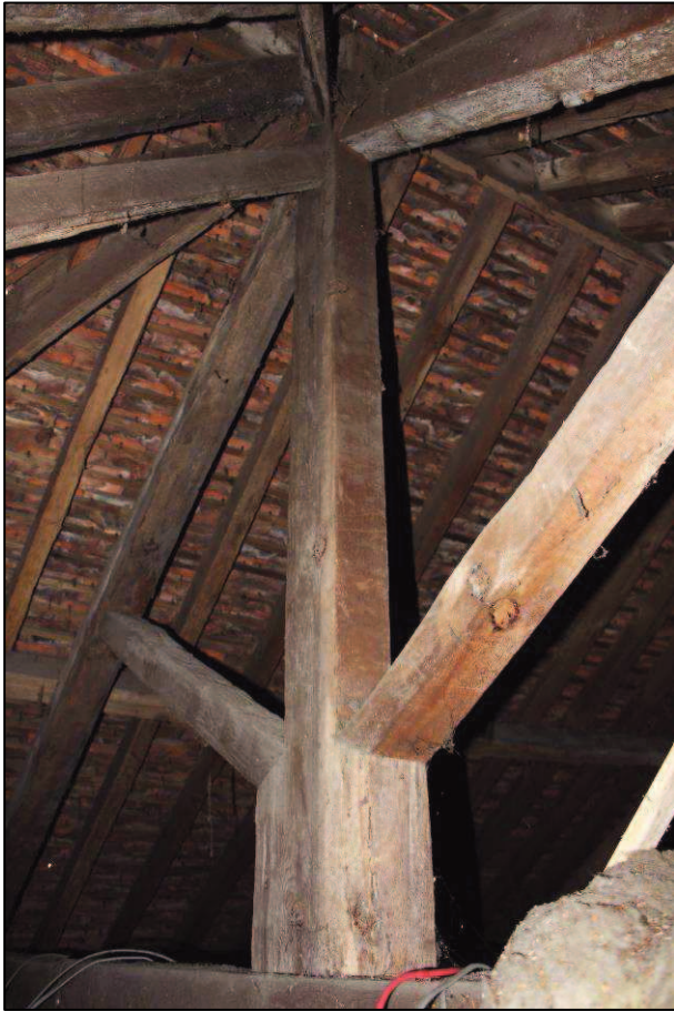
Plate 20 (Shot 39): Kingpost roof truss above the main pub, looking southeast
