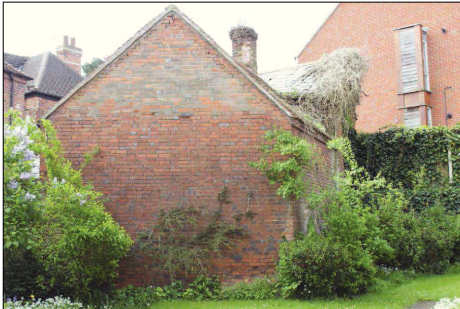
Plate 35 (Shot 127): Northeast and northwest elevations of the store, looking south
