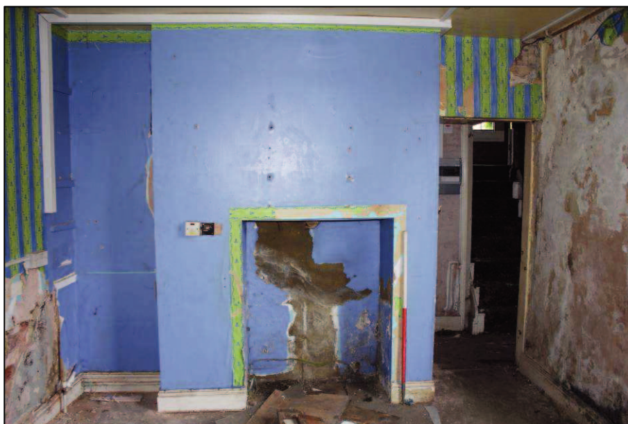
Plate 24 (Shot 17): Disused fireplace in the back room, looking southwest, 1m scale
