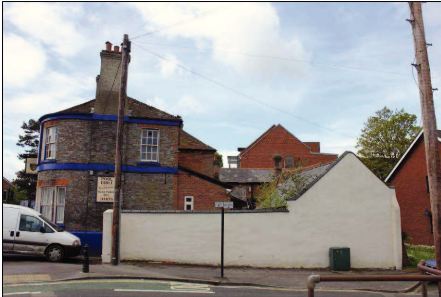
Plate 40 (Shot 117): Northeast elevation and boundary wall, looking southwest
