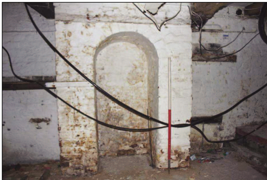
Plate 12 (Shot 47): Vaulted chimney base, looking southwest, 1m scale
