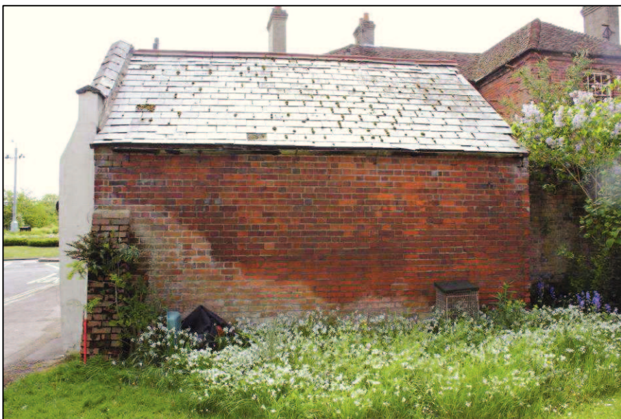
Plate 42 (Shot 124): Northwest elevation of garage, looking southeast, 1m scale
