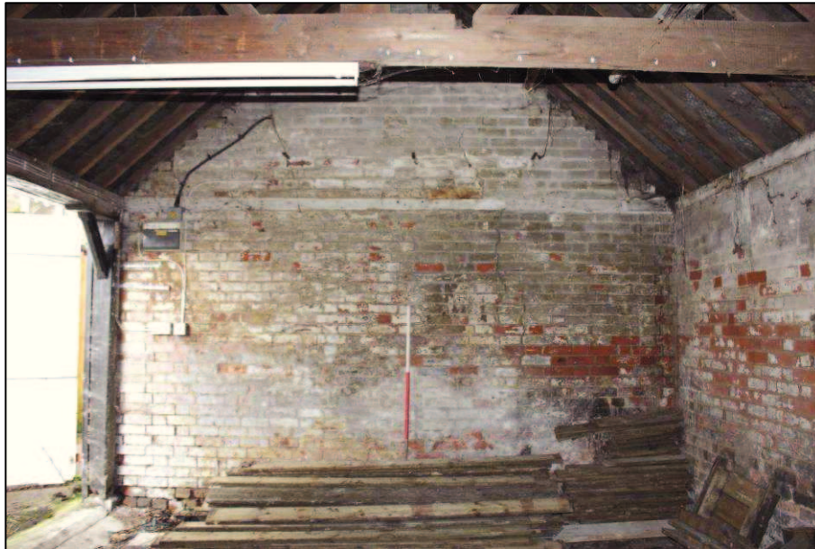
Plate 43 (Shot 82): Southwest internal elevation of the garage, looking southwest, 1m scale
