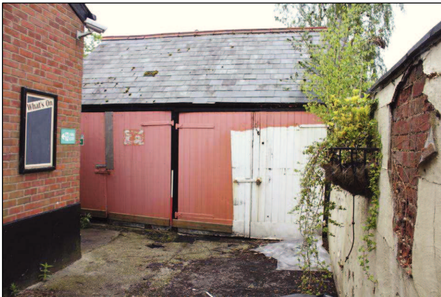
Plate 41 (Shot 90): Southeast elevation of the garage, looking west, 1m scale
