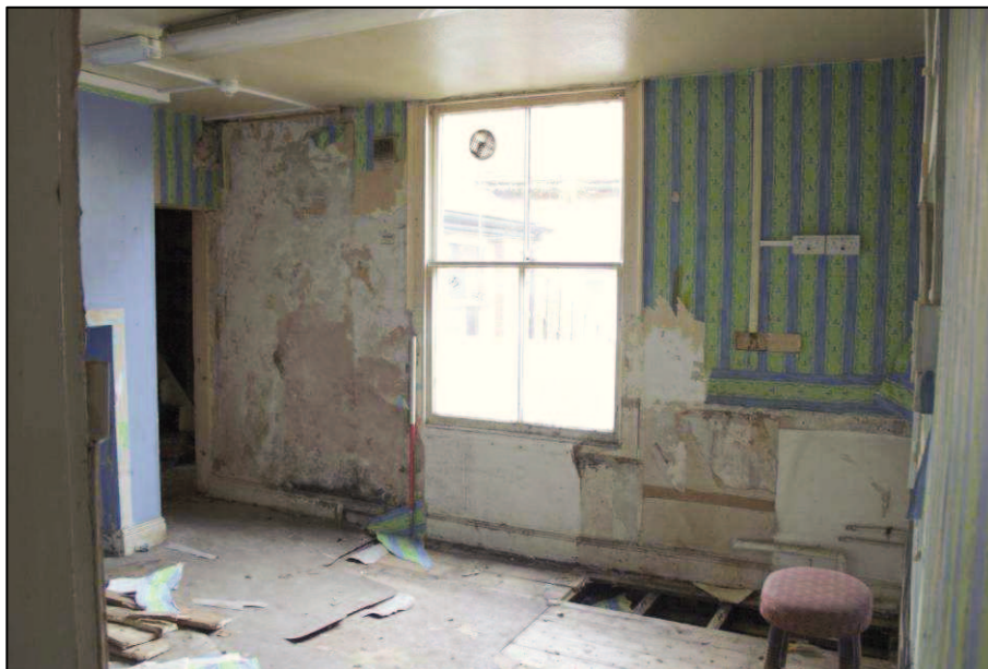
Plate 23 (Shot 16): Back room in the extension, looking west, 1m scale
