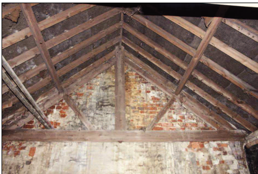
Plate 45 (Shot 84): Kingpost roof structure looking northeast
