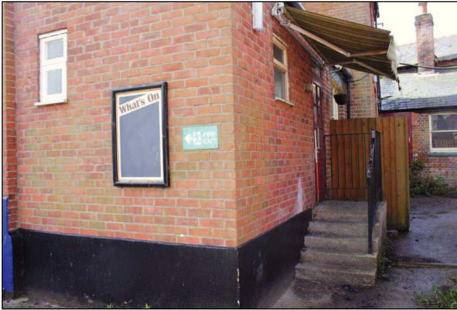
Plate 49 (Shot 111): Northeast elevation of toilet block, looking southeast, 1m scale
