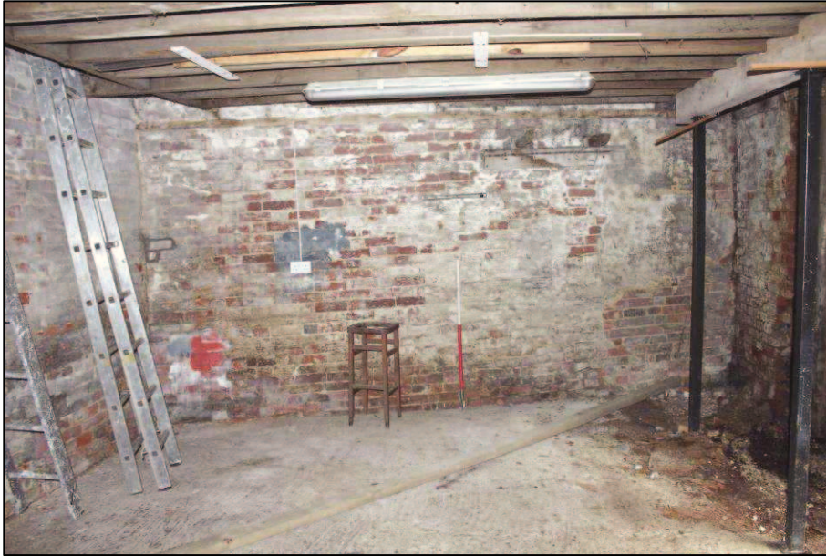
Plate 37 (Shot 68): Northeast elevation of the store, 1m scale
