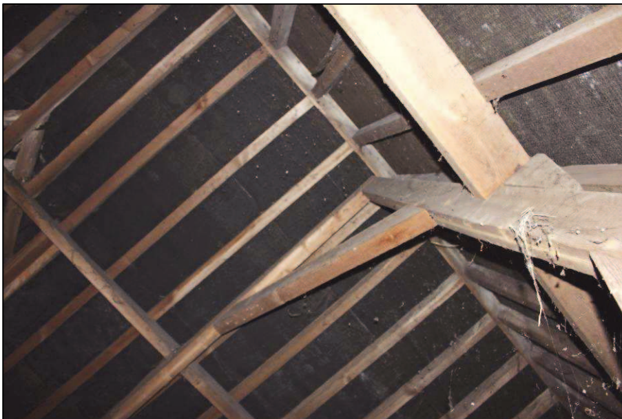
Plate 39 (Shot 73): Roof structure, looking south
