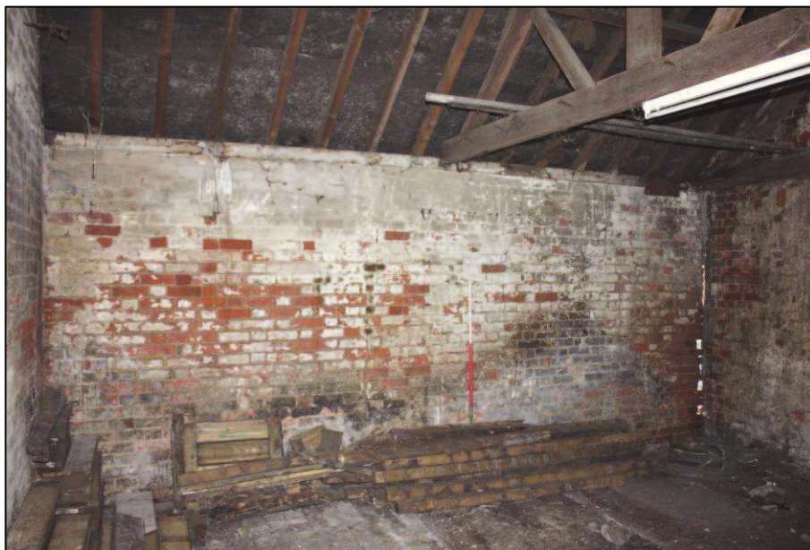
Plate 44 (Shot 88): General view of the garage interior, looking northwest, 1m scale
