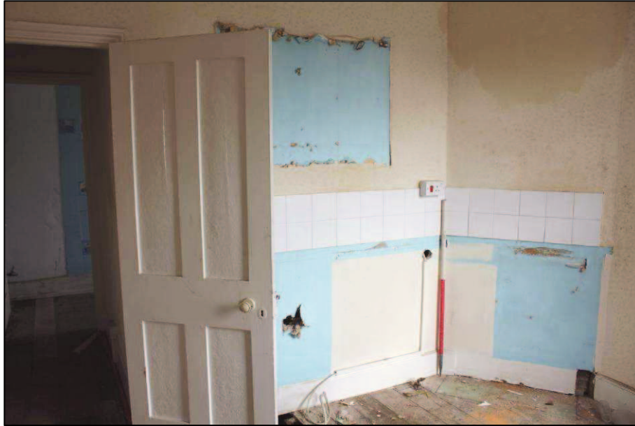
Plate 19 (Shot 34): General view of the kitchen, looking northwest, 1m scale
