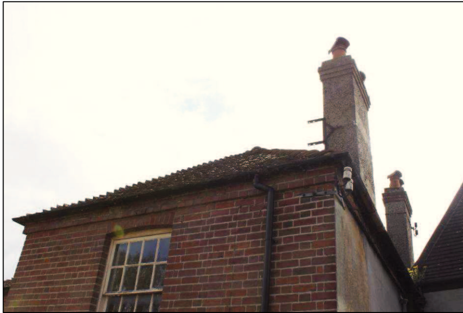
Plate 22 (Shot 106): Roof of pub extension, looking east
