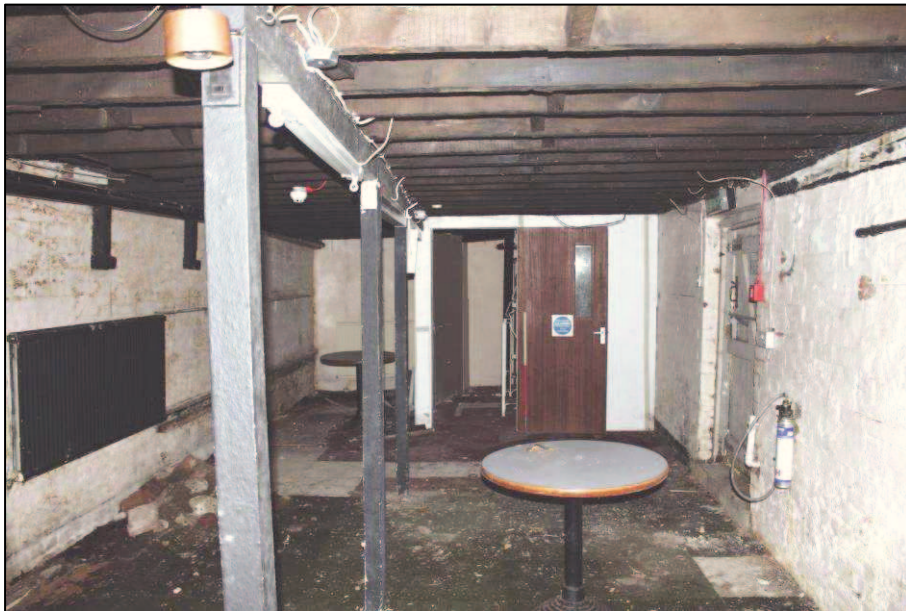
Plate 32 (Shot 64): Ground floor showing supporting columns, looking northwest, 1m scale
