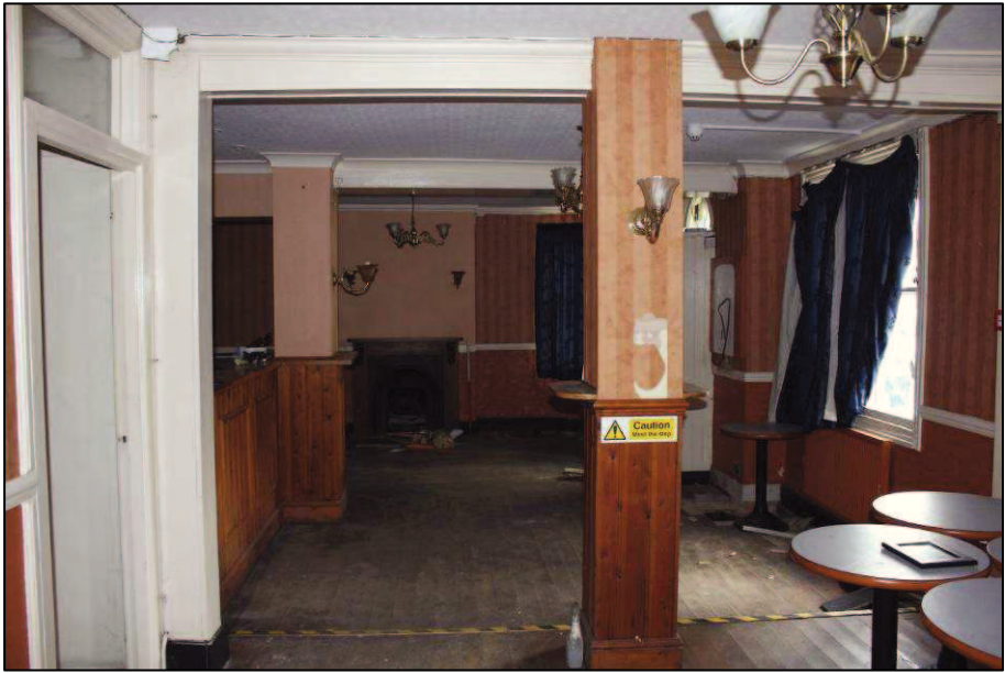
Plate 9 (Shot 12): Pub area on ground floor, looking northeast, 1m scale
