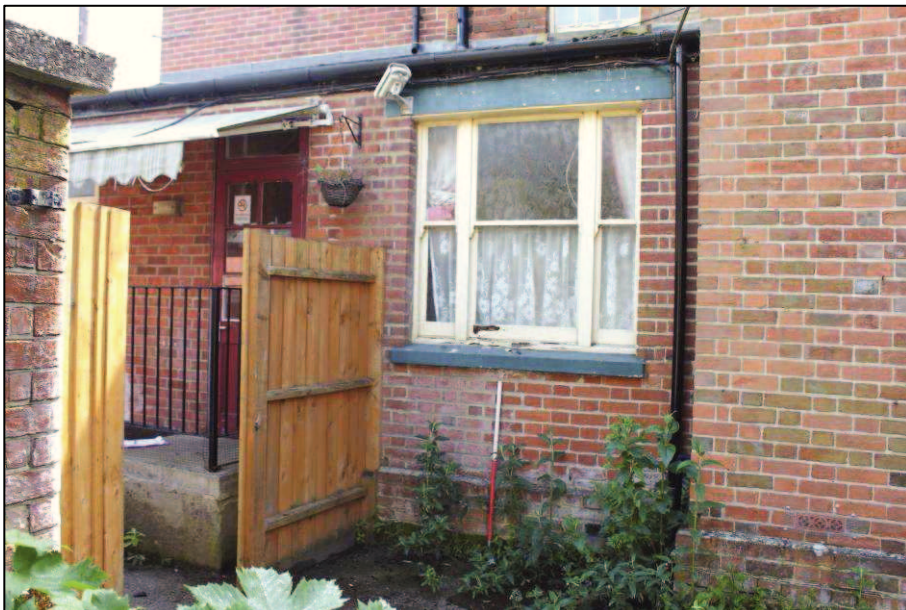
Plate 48 (Shot 110): Northwest elevation of toilet block, looking east, 1m scale
