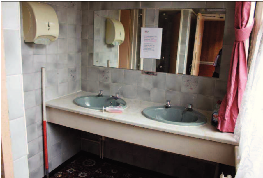
Plate 50 (Shot 06). Ladies toilet, looking south, 1m scale
