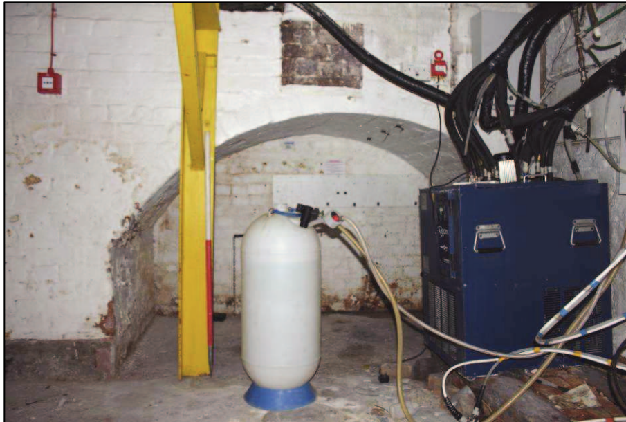
Plate 13 (Shot 49): Vaulted storage cell on the northwest elevation, 1m scale
