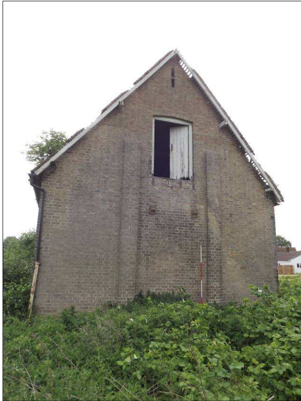
Plate 1 (Shot 9): Western gable of Building A, looking east-northeast. 2m scale
