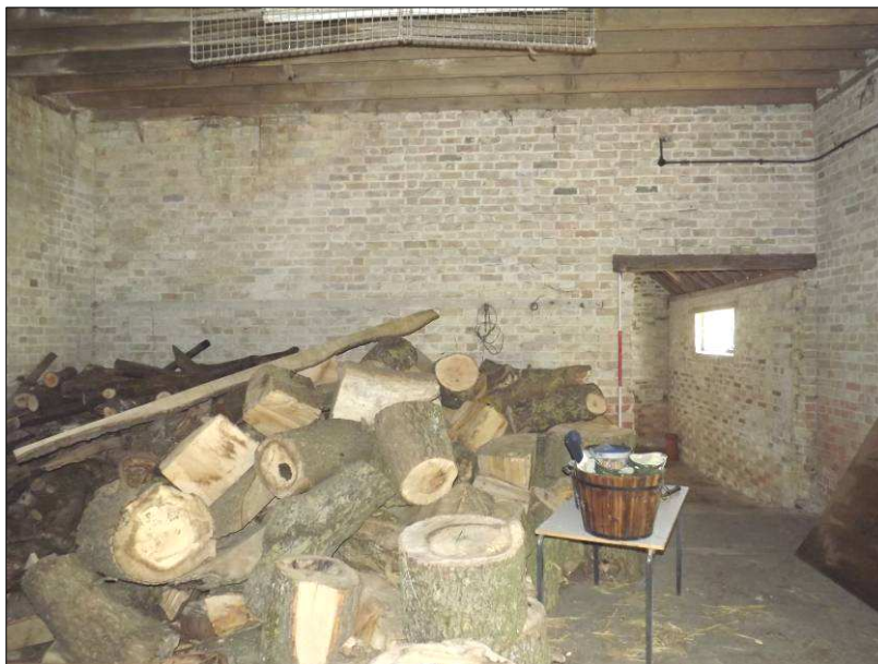
Plate 4 (Shot 57): Building A interior, looking east-northeast. 2m scale
