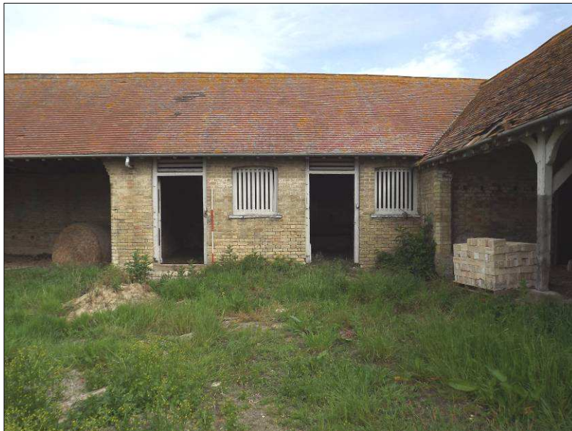
Plate 12 (Shot 6): South elevation of B5 and B6, looking north-northwest. 2m scale
