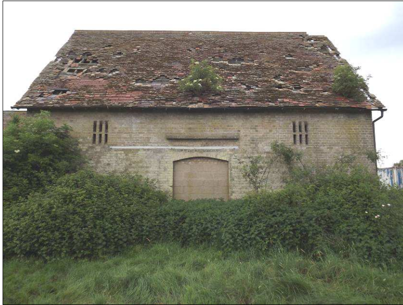
Plate 3 (Shot 10): North elevation of Building A, looking south-southeast
