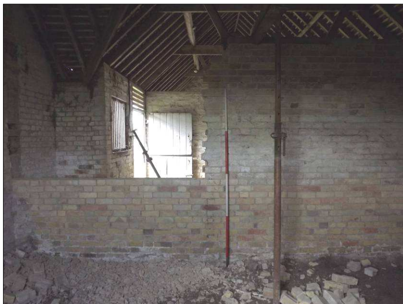
Plate 15 (Shot 33): Partition between B6 and B7, looking west-southwest. 2m scale
