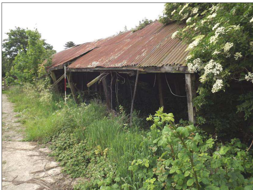
Plate 21 (Shot 15): Building D, east elevation, looking south. 2m scale
