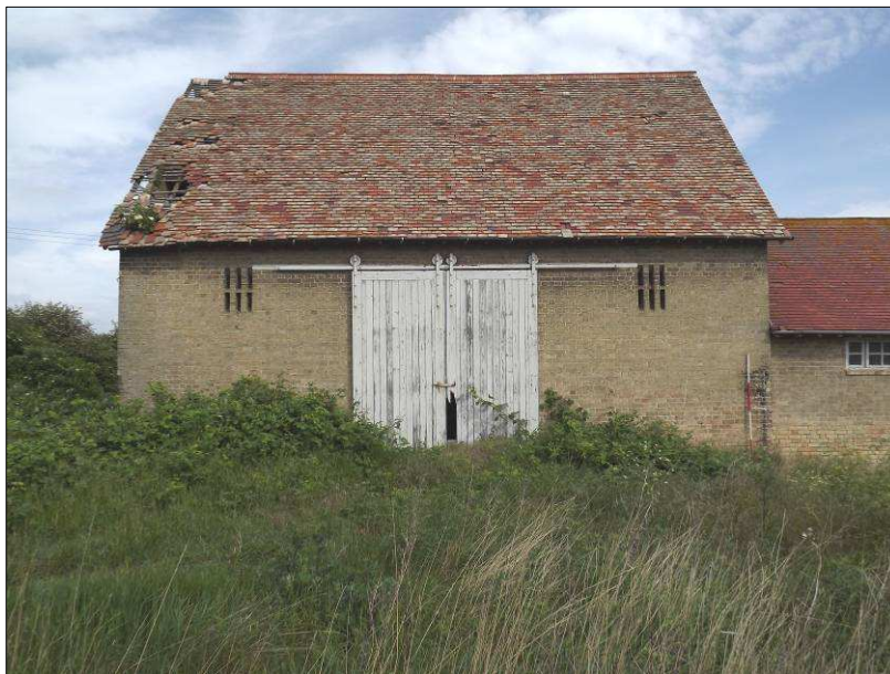
Plate 2 (Shot 2): South elevation of Building A, looking north-northwest. 2m scale
