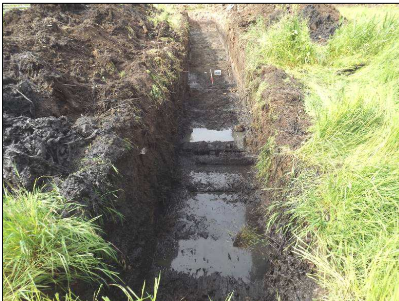
Plate 26: Trench 3 looking southwest. 1m scale
