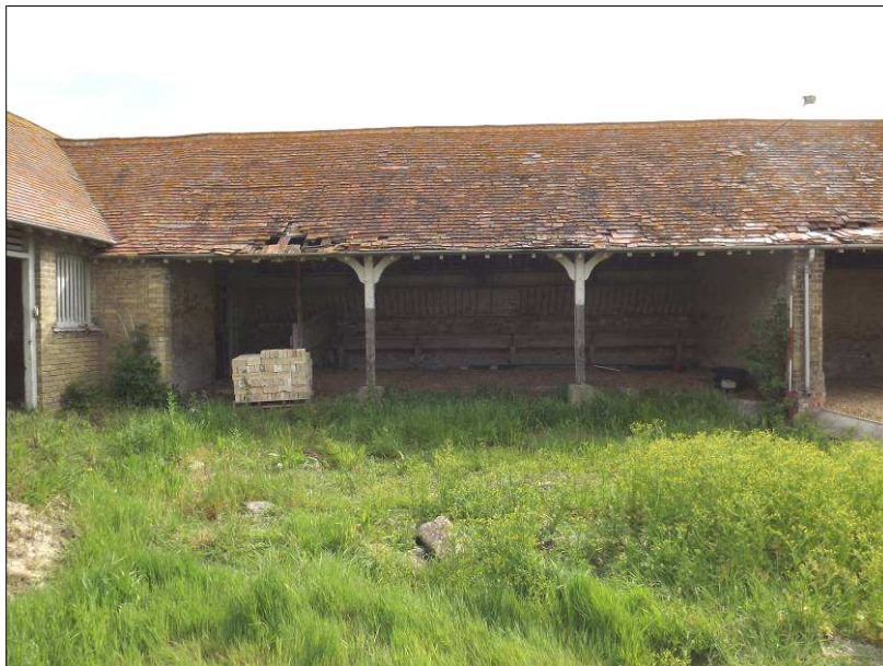
Plate 17 (Shot 7): West elevation of C1, looking east-northeast. 2m scale
