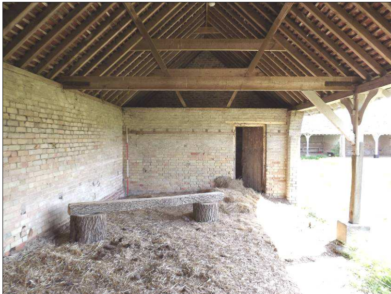
Plate 7 (Shot 47): B2 interior and roof structure, looking east-northeast. 2m scale
