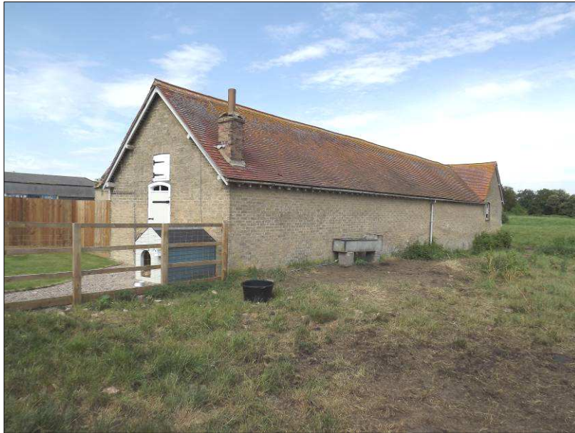
Plate 16 (Shot 75): Building C, south and east elevations, looking northwest. 2m scale
