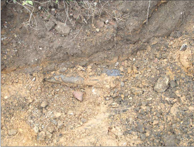
Plate 2: Exposure of large cable/service pipe in Trench 2.
