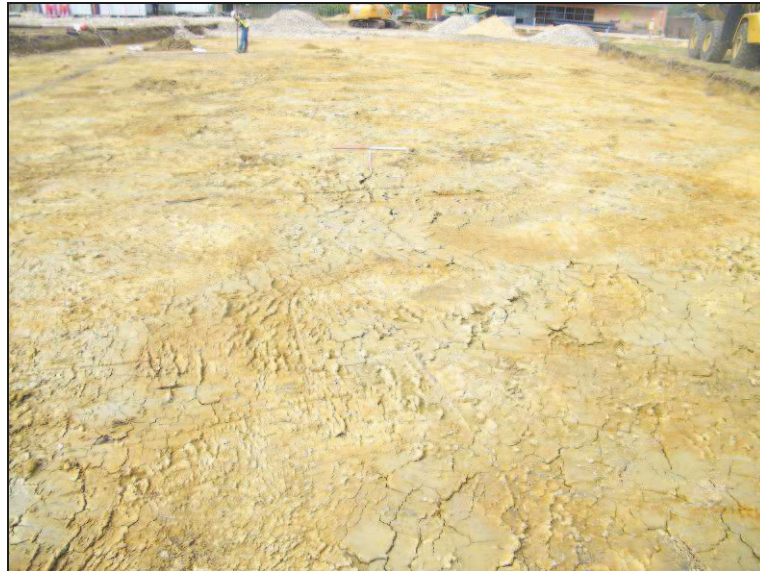
Plate 1: General shot of site, looking west with two 1m scales
