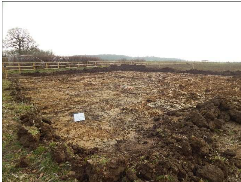
Plate 1: General view of site after machine stripping, looking southwest
