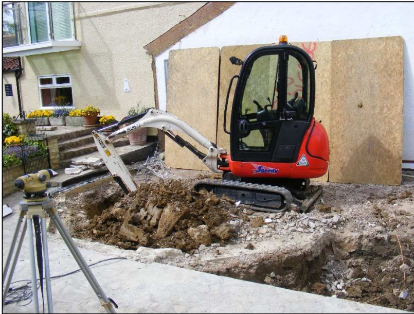
Plate 1: Northwest view of the development area during excavation
