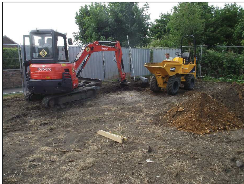
Plate 1: Machine excavation being undertaken during groundworks, looking southeast
