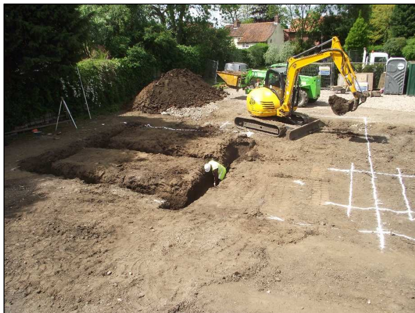
Plate 1: View of the development area during excavation, looking south.
