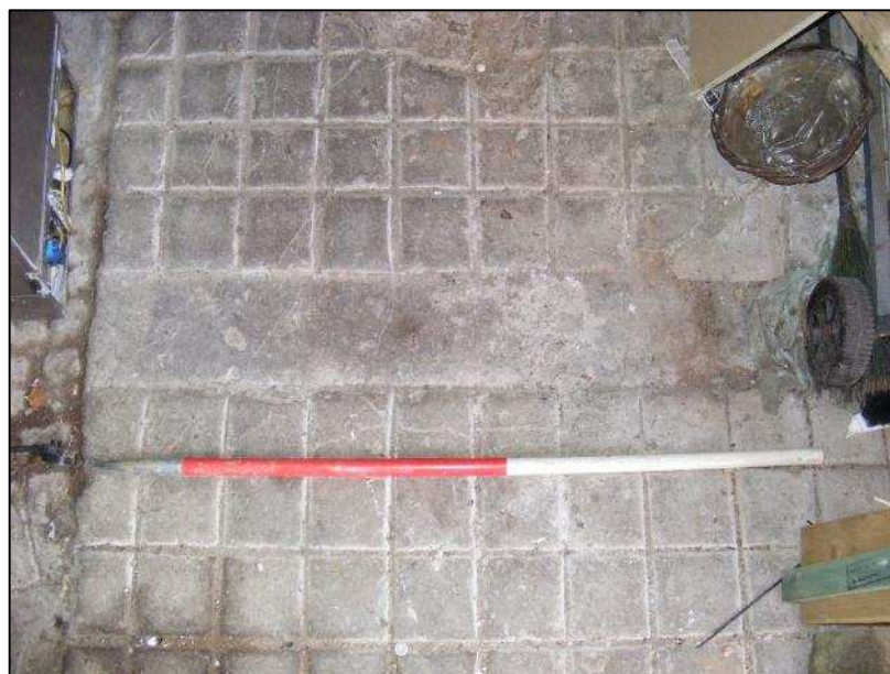
Plate 15 (shot 15): Interior of north-south aligned range, detail of flooring and drainage channel. 1m scale.
