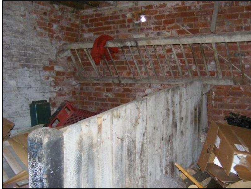
Plate 16 (shot 14): Interior of north-south aligned range, detail of stall division and manger
