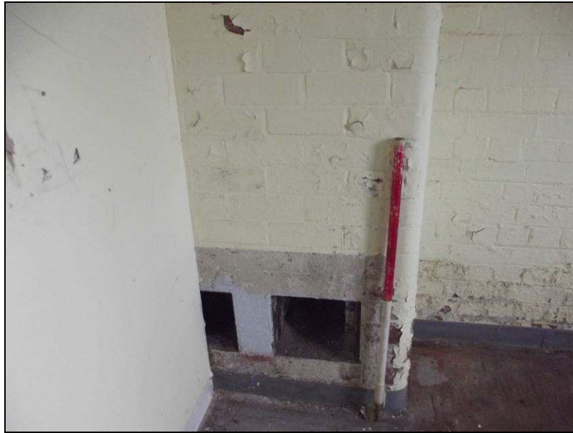
Plate 57 (shot 23): Partition abutting fireplace in D1, looking south
