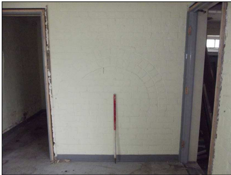
Plate 60 (shot 8): Bricked up semi-circular archway in the first southern extension of Dragonby Building. Looking east
