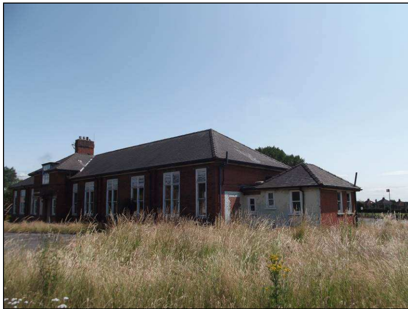
Plate 68 (shot 318): View of the north-western facing elevation of Epworth House. The simple layout is indicative of its modernist design, looking northeast
