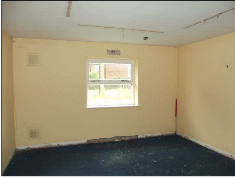
Plate 49 (shot 256): Room in C4, looking southeast
