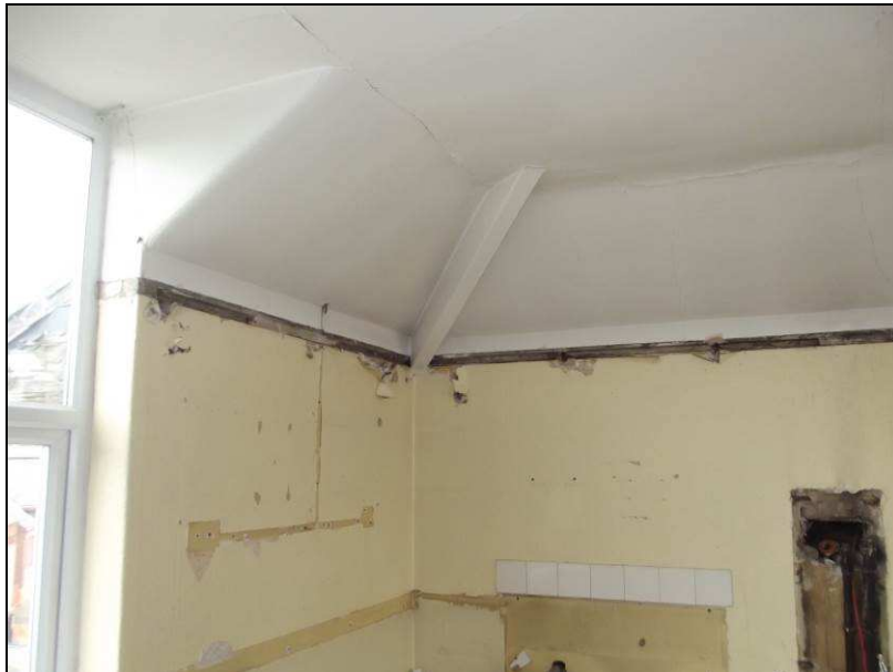
Plate 74 (shot 75): First floor of Epworth House, looking northwest
