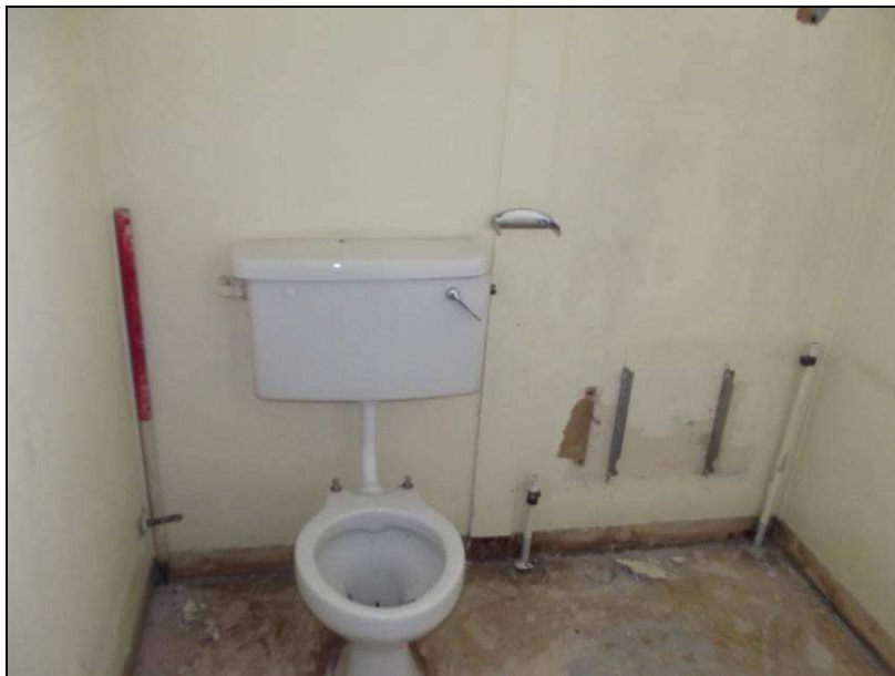
Plate 4 (shot 365): One of the lavatories in Ashby House, looking west
