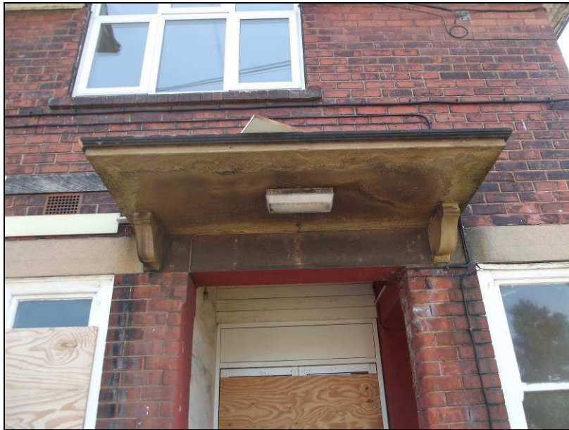
Plate 70 (shot 304): Awning on the main entrance of Epworth House, looking southeast
