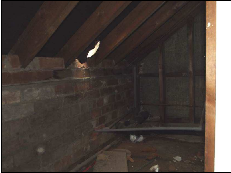
Plate 35 (shot 208): Timber framed roof visible through crawl space, looking southwest
