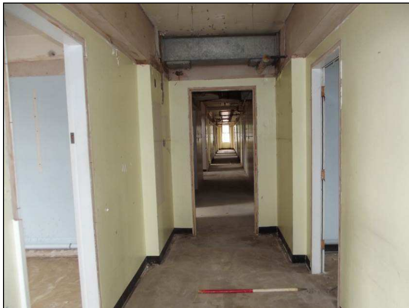
Plate 26 (shot 195): Corridor on the first floor of Barton House, looking west
