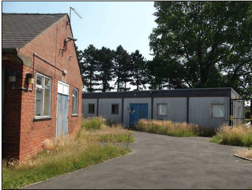
Plate 41 (shot 278): Prefabricated extension to the rear of Crosby House, looking east
