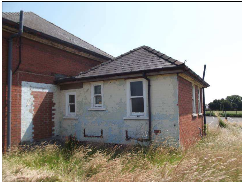
Plate 66 (shot 316): An extension has been removed from the southern end of Epworth House, looking east
