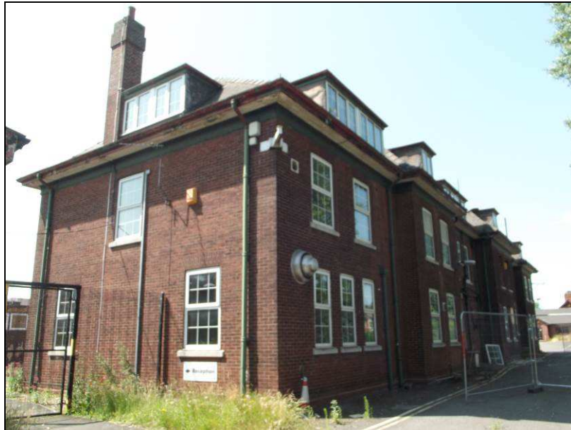
Plate 7 (shot 298): View of Barton House taken from the northeast looking southwest
