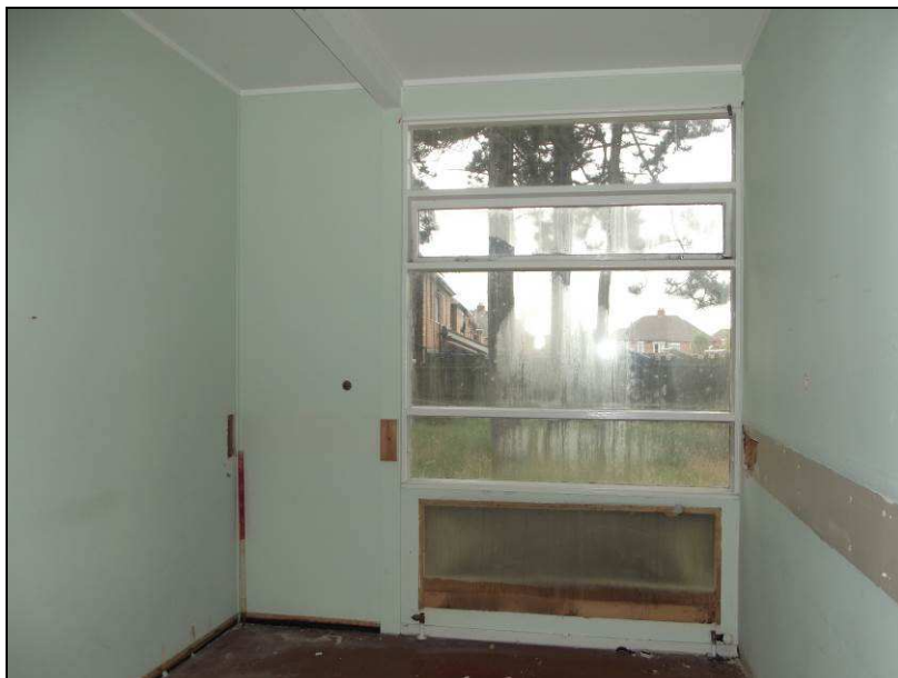
Plate 2 (shot 341): One of the office rooms in Ashby House, looking east
