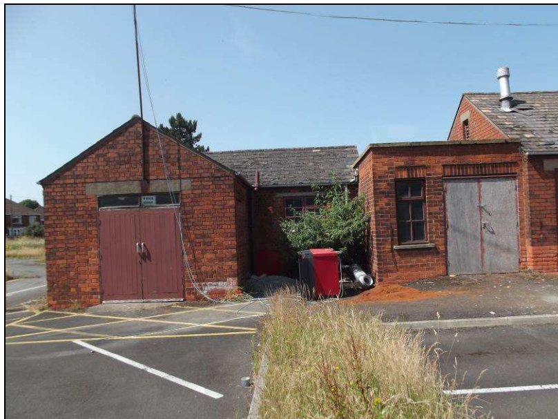
Plate 52 (shot 327): View of both southern extensions to Dragonby House, looking west
