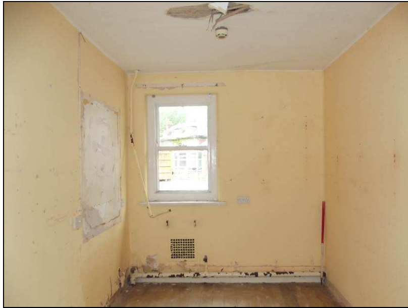
Plate 47 (shot 246): One of the small office spaces in C3, looking northwest
