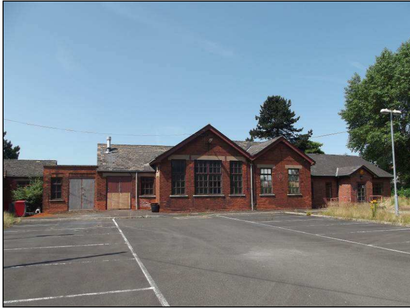
Plate 50 (shot 325): Exterior of Dragonby building, looking west
