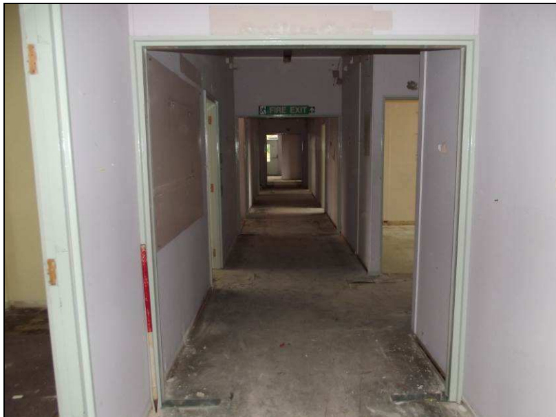
Plate 6 (shot 354): Eastern corridor of Ashby House, looking south
