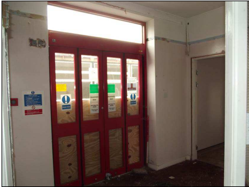
Plate 13 (shot 96): Eastern extension to Barton House, entrance, looking southwest
