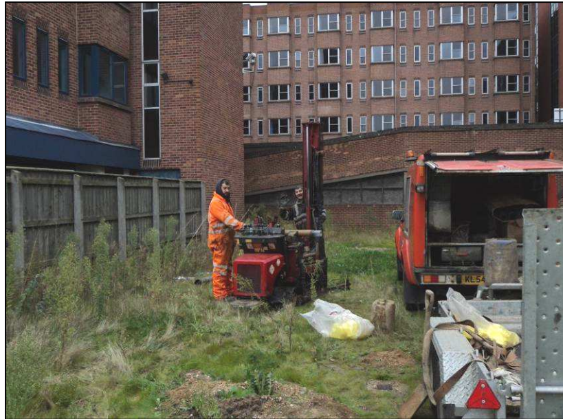
Plate 1: Dando Terrier rig set up over BH2 at Mill House, Lincoln
