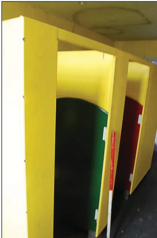
Plate 42 (shot 80): Toilet cubicles, looking west, scale 1m
