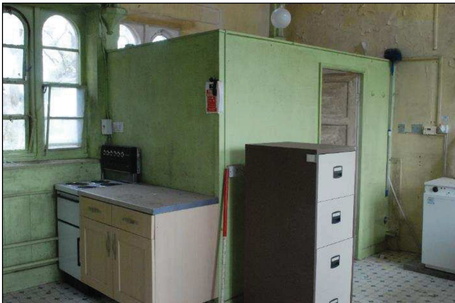
Plate 36 (shot 63): Partitions inserted into the kitchen to create a storage room, looking north, scale 1m
