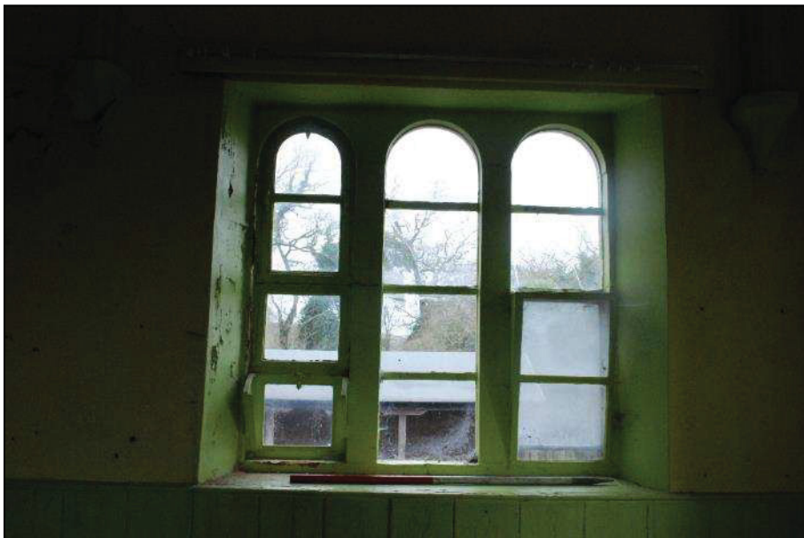
Plate 20 (shot 5): Triple window in the southern bay, looking northeast, scale 1m
