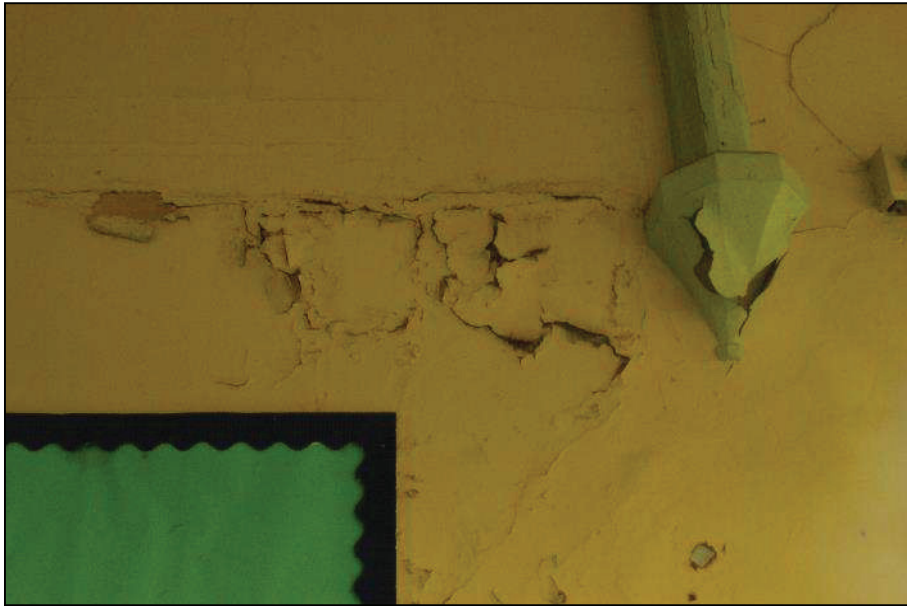
Plate 21 (shot 26): A blocked up window can be made out by the remaining lintel which has been painted over, looking northeast
