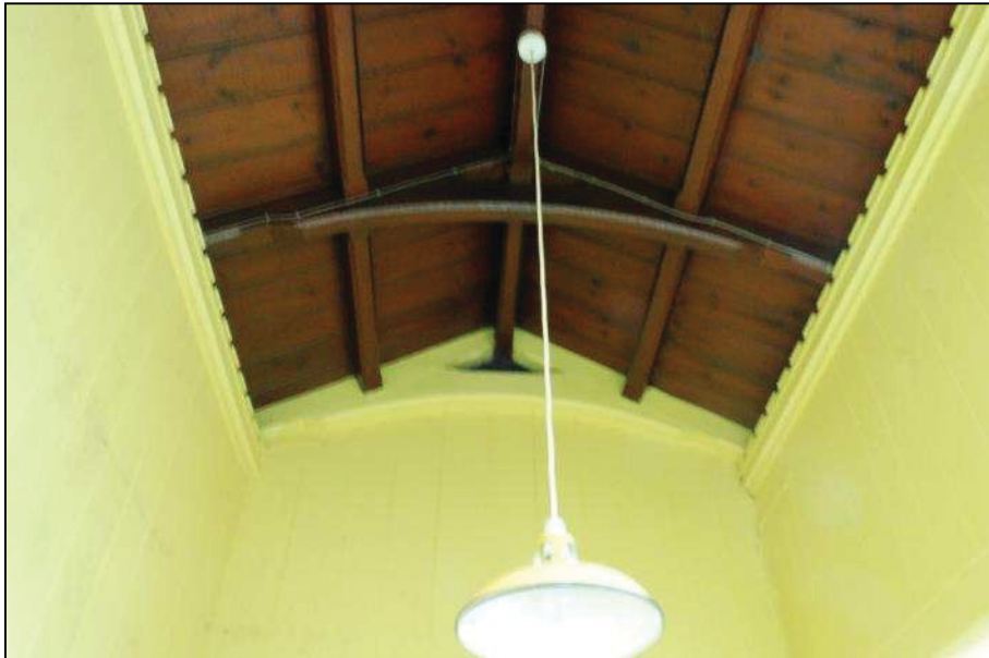
Plate 16 (shot 98): View of the timber roof in the entranceway, looking southwest
