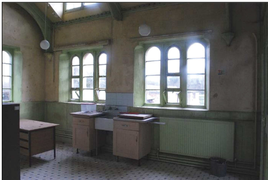
Plate 34 (shot 50): General interior view of the kitchen, looking east, scale 1m
