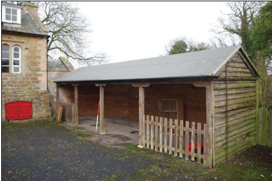
Plate 14 (shot 136): Timber framed shelter in the playground, looking north (1m scale)
