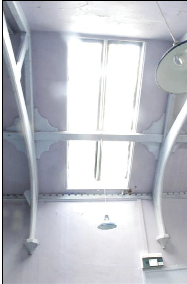
Plate 27 (shot 47): Skylight in the northwest elevation, looking northwest
