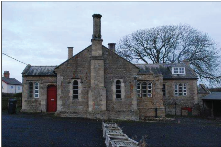
Plate 1 (shot 110): Southeast elevation of the school building: the gable end at the centre of the building is the second classroom; the porch can be seen to the left of the image; the 1930s main entrance can be seen to the right and behind this the original building can be seen. Looking northwest, scale 1m
