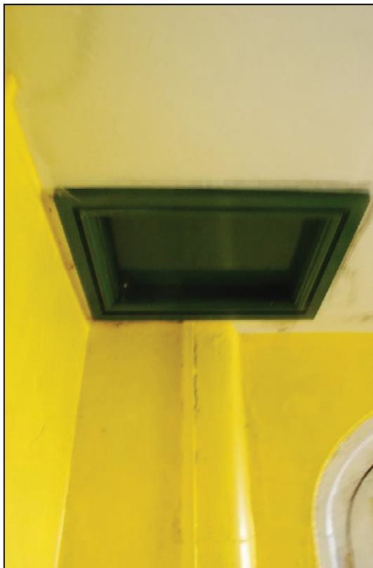
Plate 40 (shot 87): Entrance to the roof from the toilet block, looking northeast
