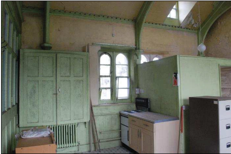
Plate 35 (shot 64): Windows in the northwest elevation, looking north, scale 1m
