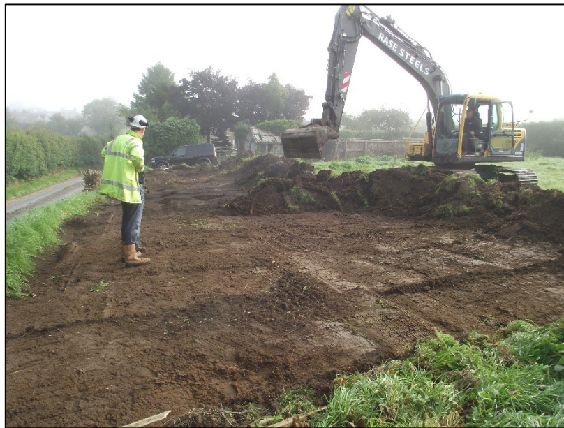
Plate 1: General view of the site during topsoil stripping, looking northeast
