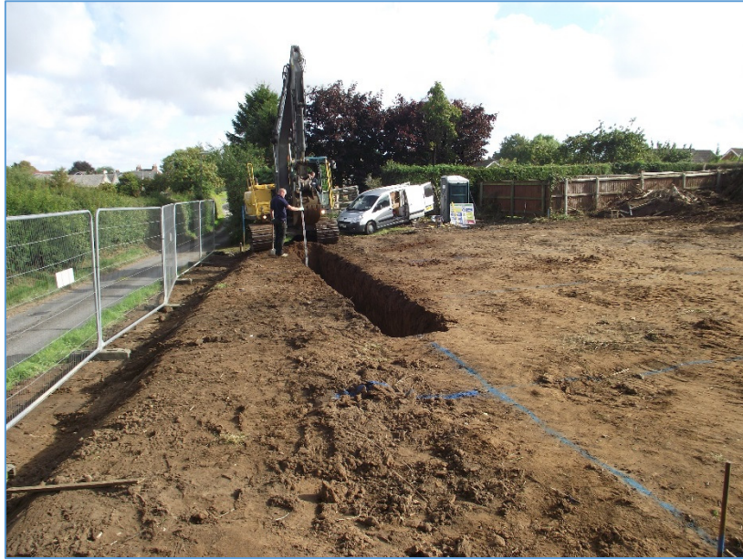
Plate 2: General view of the footings during excavation, looking west
