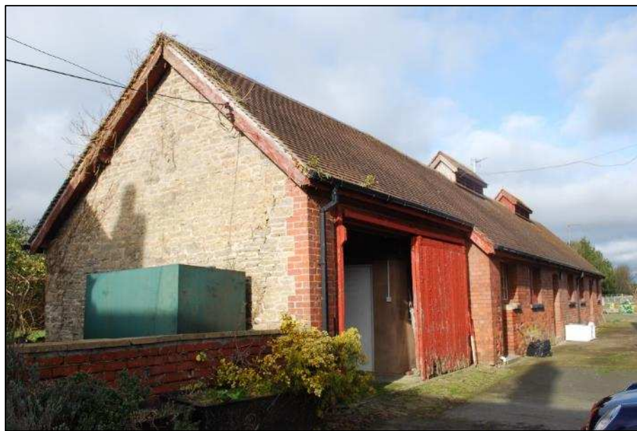
Plate 21 (Shot 117): Southern extent of Building D, the interplay between the red brick and stone rubble is clear, looking northwest
