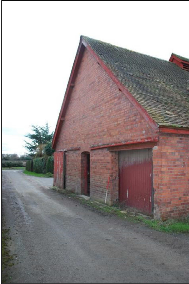
Plate 9 (Shot 18): East facing elevation pierced by a stable door and two larger sliding doors, looking southwest
