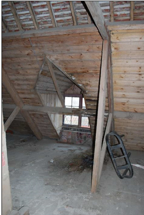
Plate 16 (Shot 3): North facing dormer window at the eastern end of building C. The central window differs from this as the lower purlin, which currently blocks the window has been raised to allow access to the door, looking north
