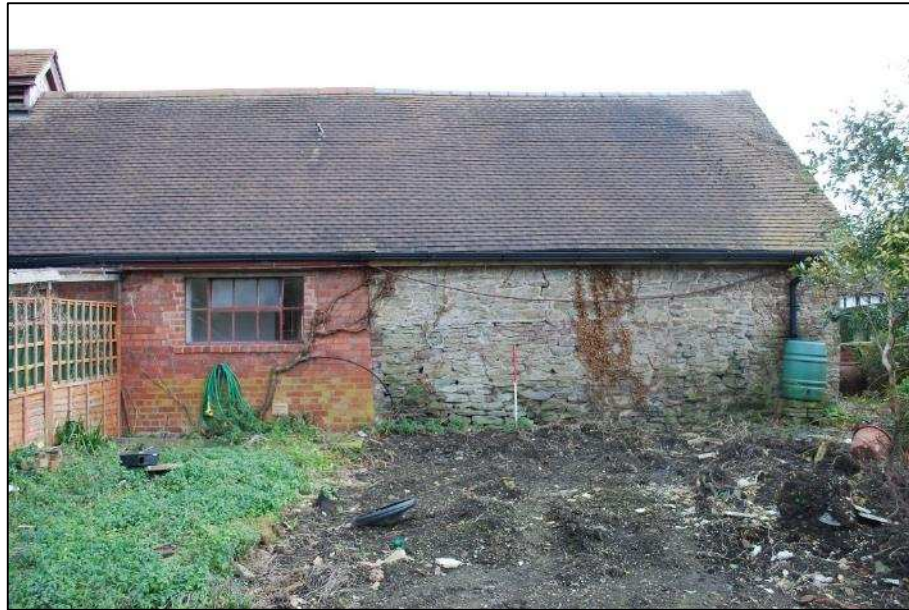
Plate 20 (Shot 103): Southern extent of Building D, the change in building material shows that the building has been extended, looking east
