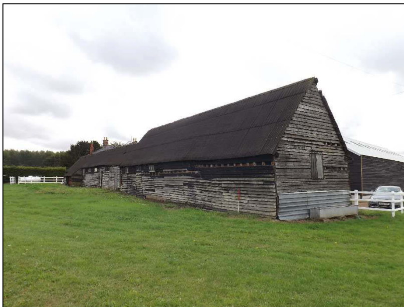
Plate 3 (shot 52): Northeast facing elevation, looking southeast
