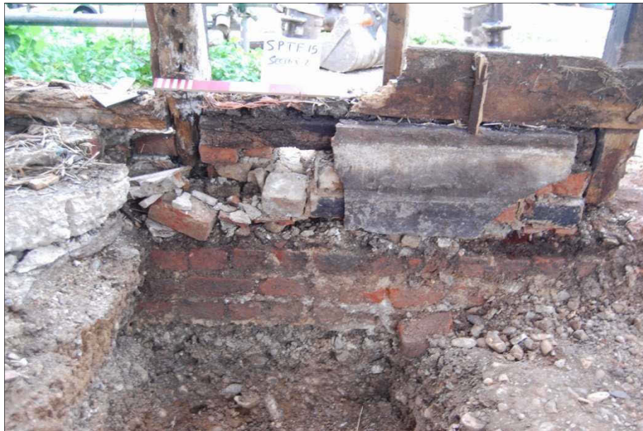
Plate 14: Northeast facing section of walls 03 and 08, scale 0.5m
