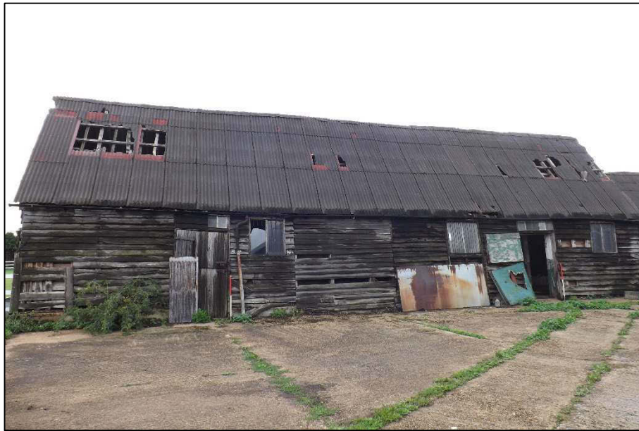
Plate 1 (shot 3): Southwest-facing elevation, looking northeast
