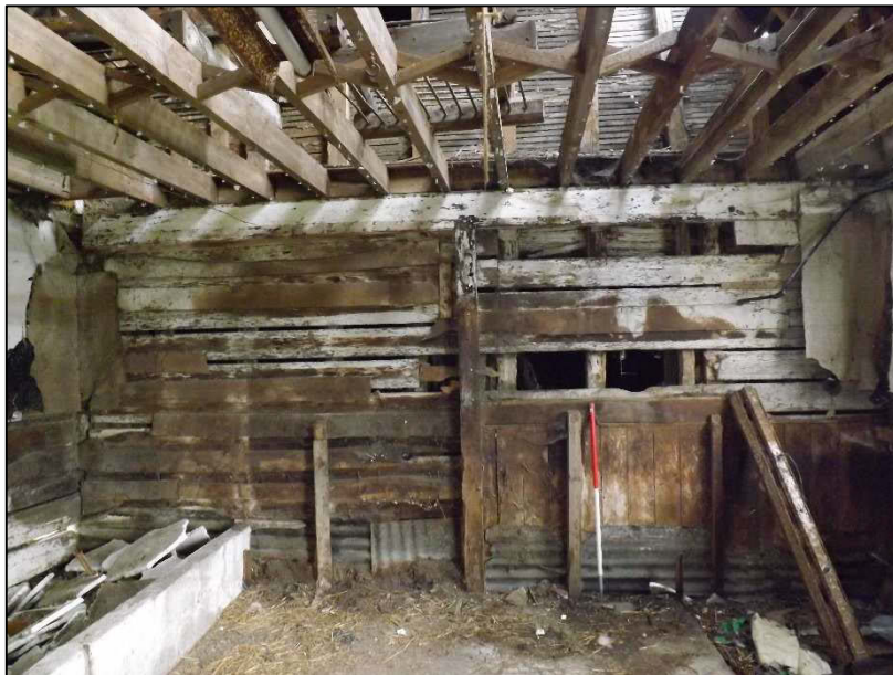
Plate 5 (shot 21): Northwest-facing internal elevation, looking southeast
