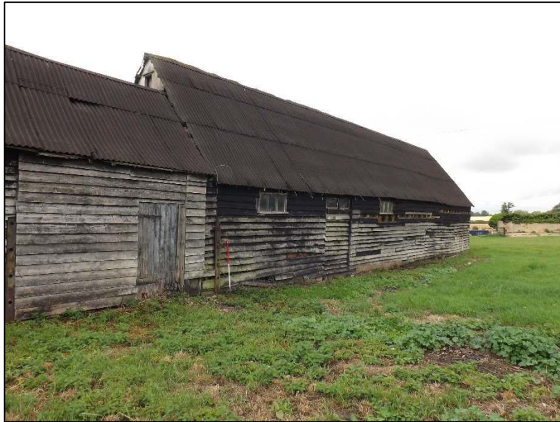
Plate 2 (shot 55): View of the northeast facing elevation, looking west
