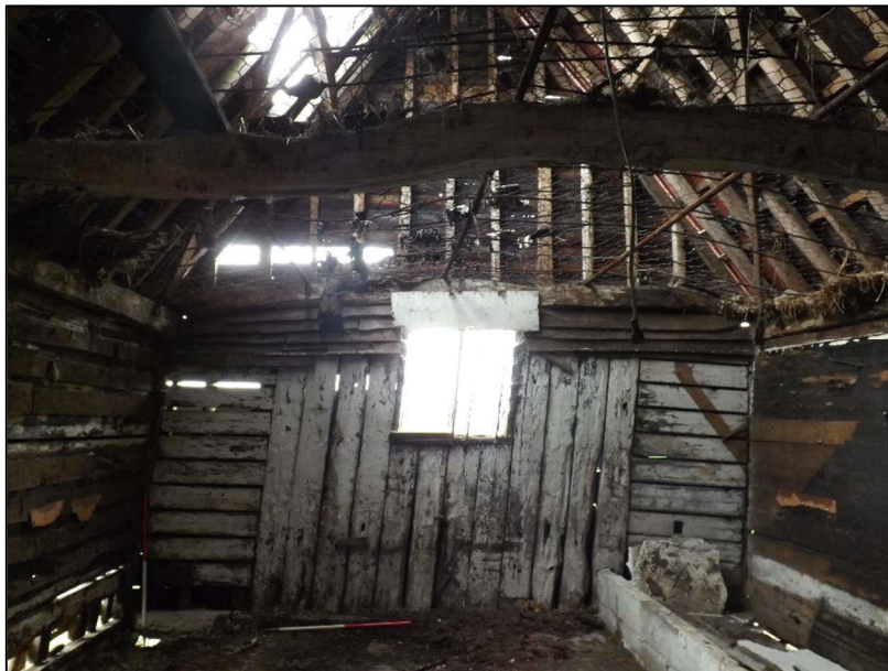
Plate 7 (shot 39): Southeast facing elevation, looking northwest
