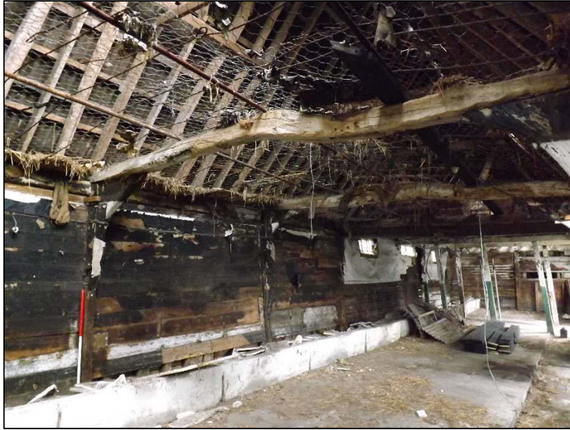
Plate 8 (shot 45): Southwest-facing elevation, looking east
