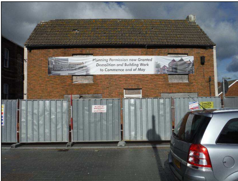
Plate 1 (Shot 1): East elevation of 6 Market Place, looking west (2m scale)
