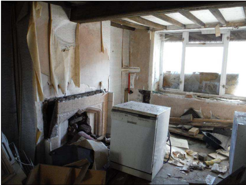
Plate 9 (Shot 60): Room 1 of the ground floor, looking northeast (1m scale)
