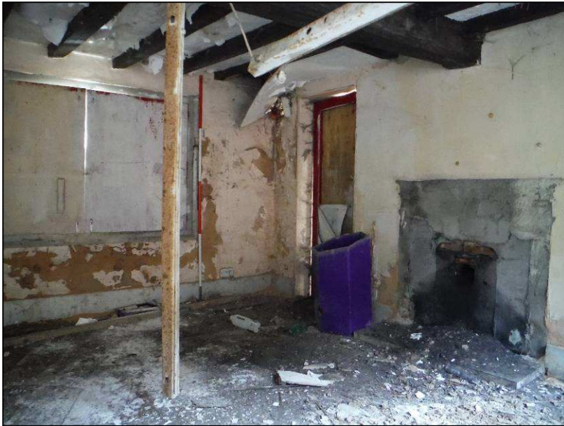
Plate 23 (Shot 36): Room 6 showing entrance, fireplace and window, looking southeast (2m scale)
