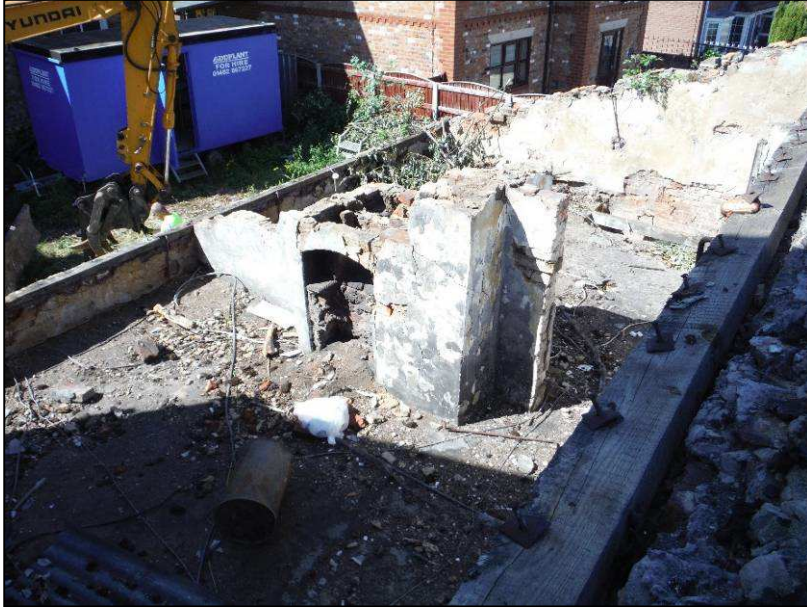
Plate 19 (Shot 91): Chimney stacks visible between Rooms 3 and 4, looking southwest
