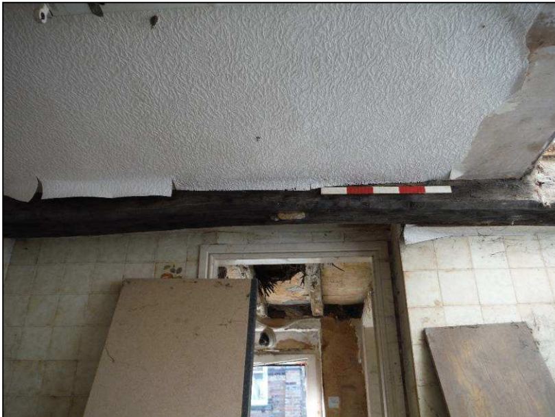
Plate 14 (Shot 49): Suspended ceiling in Room 4, looking south (40cm scale)
