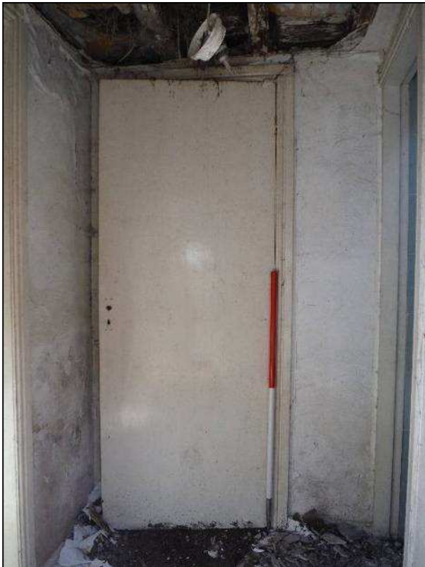
Plate 16 (Shot 40): Subdivided area in Room 3, looking north (1m scale)
