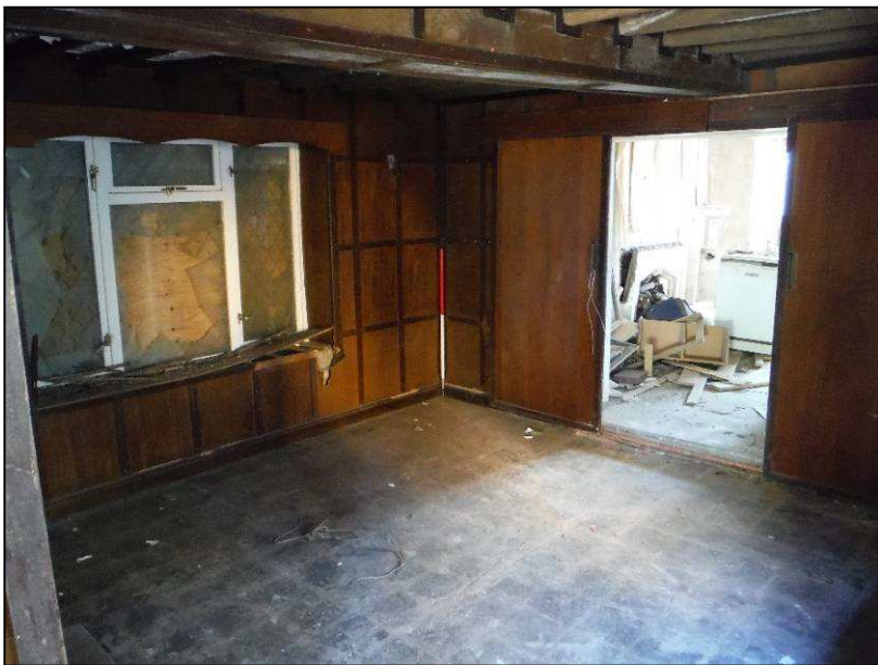
Plate 10 (Shot 54): Room 2 of the ground floor, looking northeast (1m scale)
