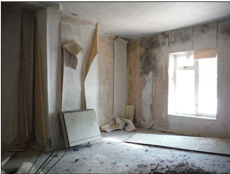
Plate 26 (Shot 67): Room 8 showing modern window and chimneystack on eastern elevation, looking northeast
