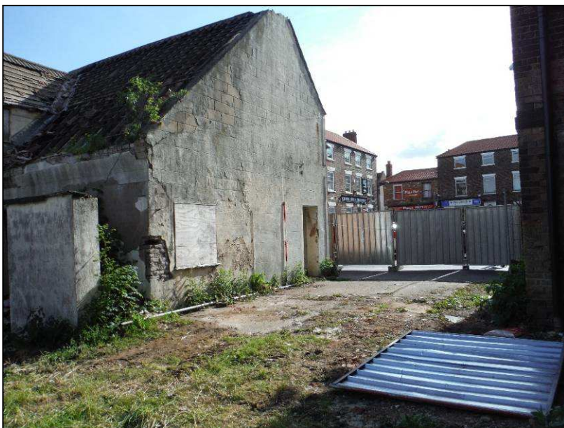
Plate 2 (Shot 5): Oblique image of the south elevation, looking northeast (2m scale)
