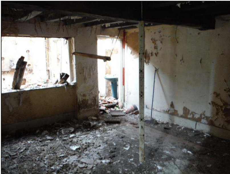
Plate 24 (Shot 34): Room 6 looking into Room 5, looking northwest (2m scale)
