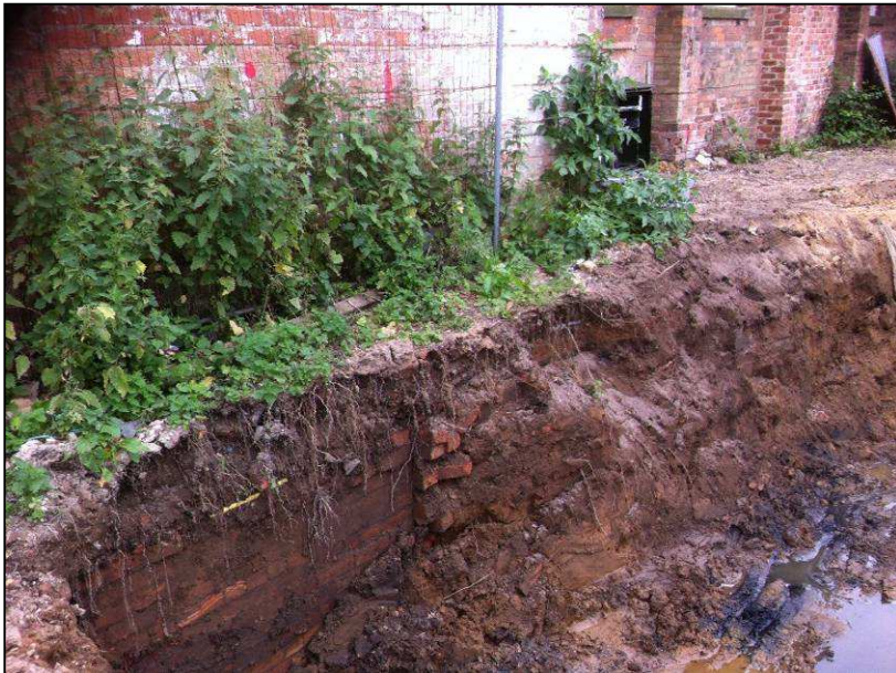
Plate 32 (Provided by client): Brick-lined cellars used to house the fuel tanks, looking southwest
