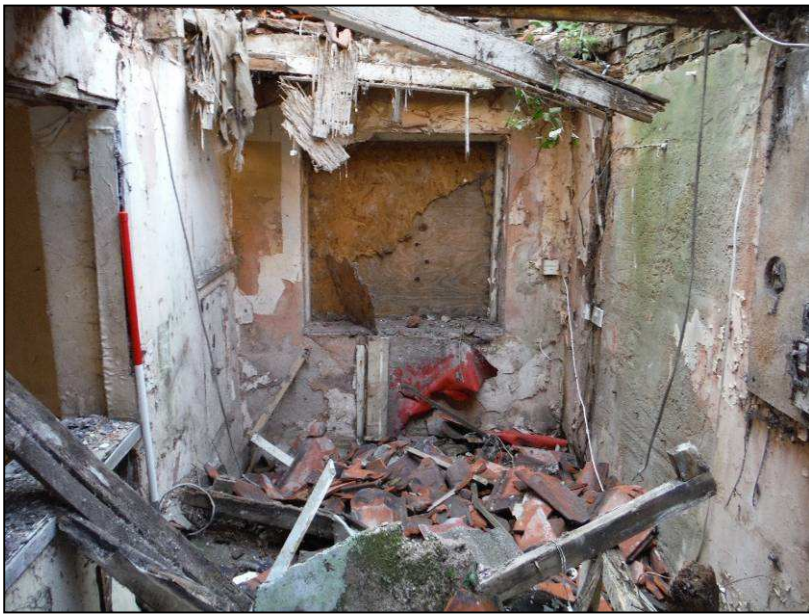
Plate 22 (Shot 76): Room 5 looking south (1m scale)
