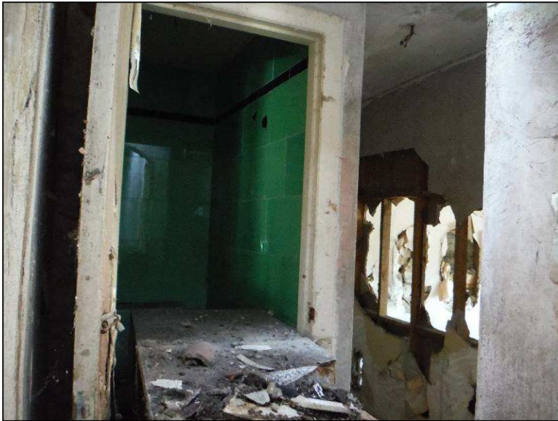
Plate 27 (Shot 72): Bathroom and dividing wall on the first floor, looking northwest
