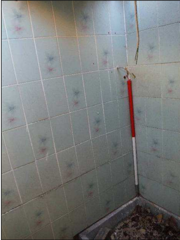
Plate 15 (Shot 42): Shower room in Room 3, looking southeast (1m scale)
