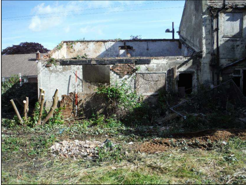
Plate 7 (Shot 10): Single storey elevation, looking north (2m scale)
