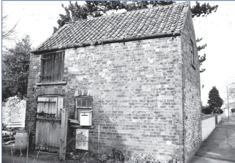
Plate 4: East elevation, looking west
