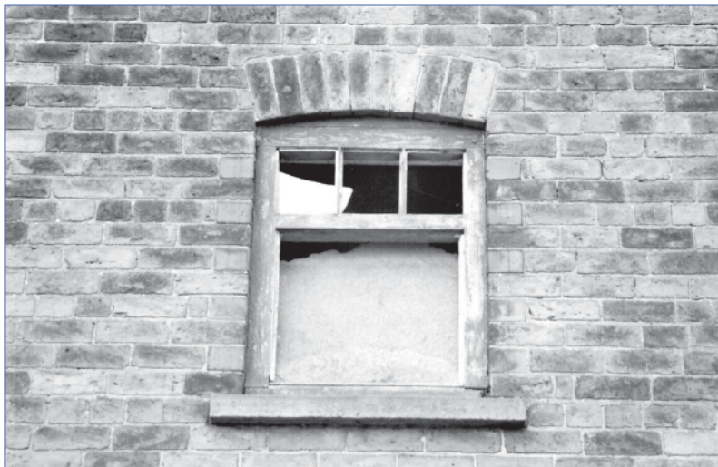
Plate 6: Window in upper storey of north elevation, looking south-south-west
