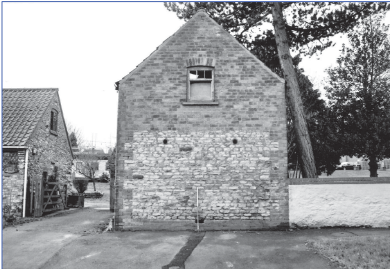
Plate 2: North elevation, looking south-south-west
