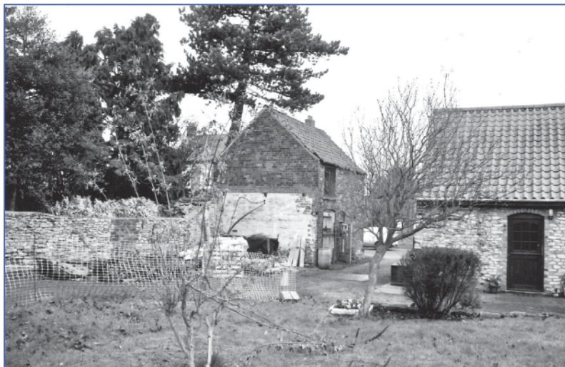
Plate 12: General view of the barn, looking north.
