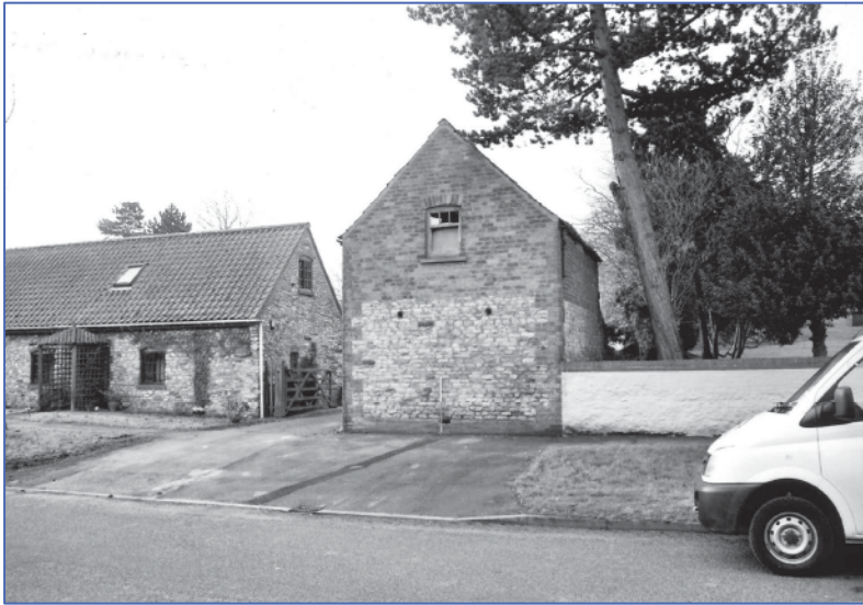
Plate 1: General shot of the barn looking south, showing the adjacent cottage.
