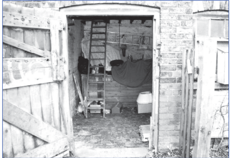
Plate 8: Interior view of the lower storey of the barn, looking west-north-west through the door towards the staircase to the upper storey.
