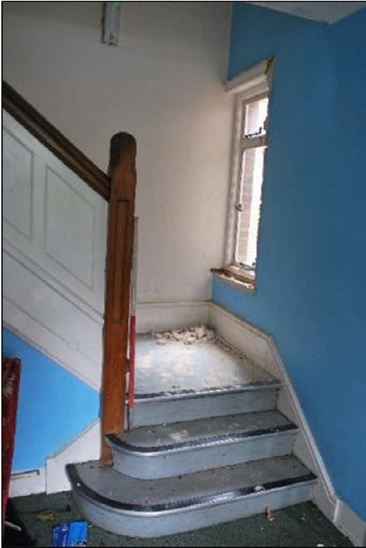
Plate 29 (Shot 210): Staircase in the entrance lobby, looking east, 1m scale
