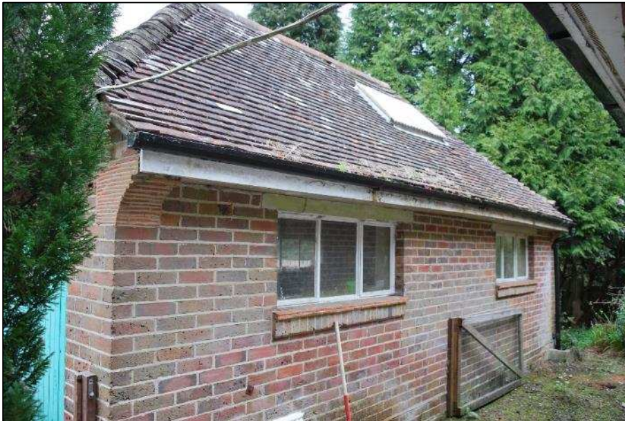
Plate 36 (Shot 337): Southeast facing elevation of the garage, looking north, 1m scale
