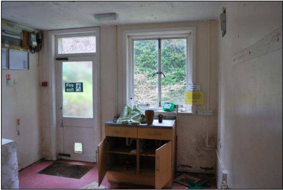
Plate 25 (Shot 179): Laundry room, looking southeast, 1m scale
