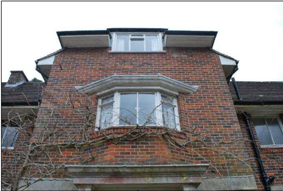
Plate 5 (Shot 81): Dormer window at second floor level which is placed through the roofline, looking northeast
