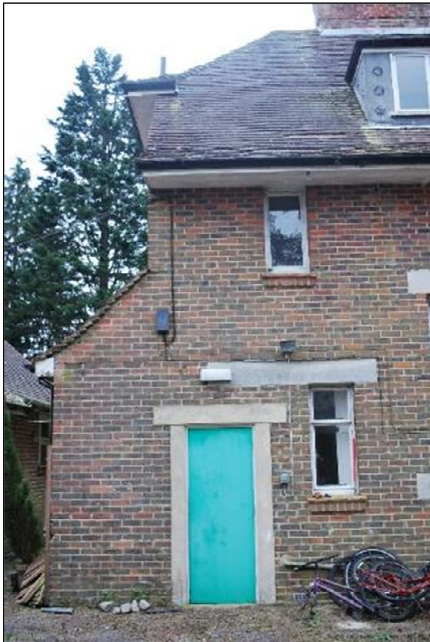
Plate 10 (Shot 28): Northern extent of Elevation D, looking southeast, 1m scale
