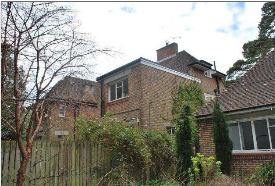
Plate 16 (Shot 372): South-eastern part of Elevation E, looking west
