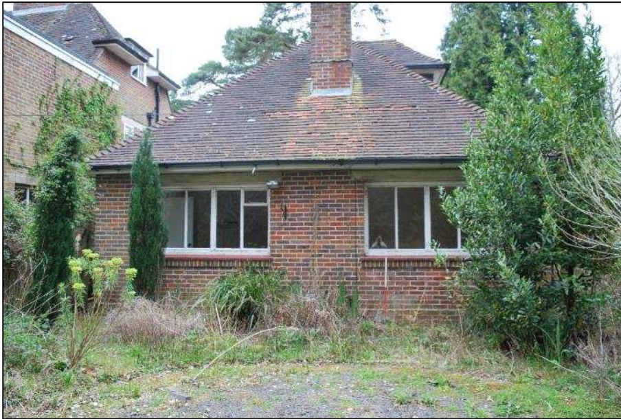
Plate 41 (Shot 370): Southeast facing elevation of the bungalow, looking northwest 1m scale
