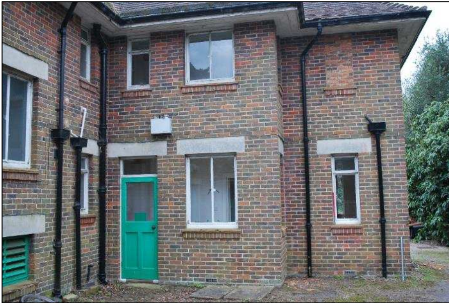
Plate 9 (Shot 5): Elevation C, looking southwest, 1m scale
