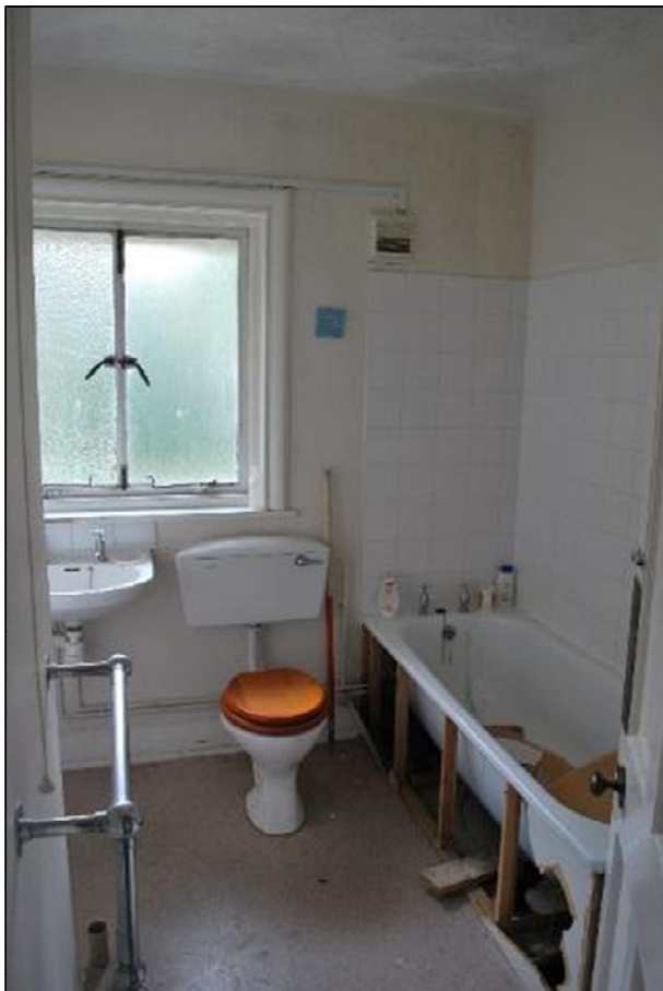
Plate 32 (Shot 230): Example of a bathroom, looking southwest
