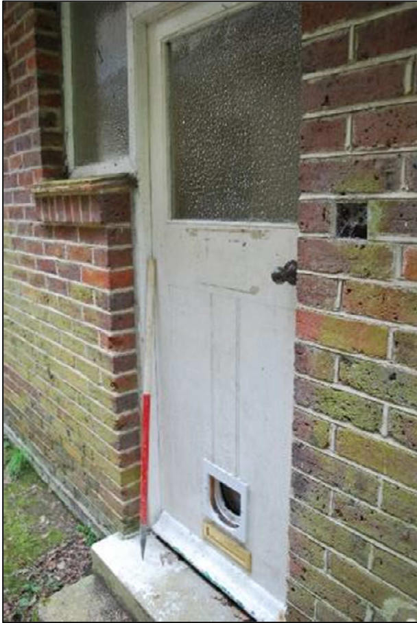
Plate 39 (Shot 365): Entrance to the bungalow, looking north, 1m scale
