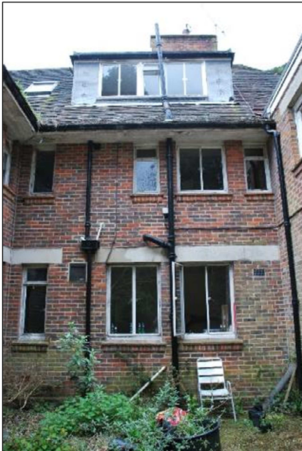
Plate 18 (Shot 54): Central section of Elevation F, looking northwest 1m scale
