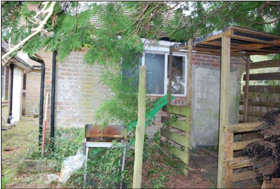
Plate 37 (Shot 342): Northeast facing elevation of the Garage, looking southwest 1m scale
