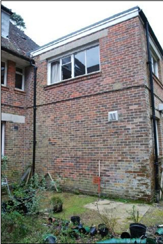
Plate 19 (Shot 51): Elevation G, looking north, 1m scale
