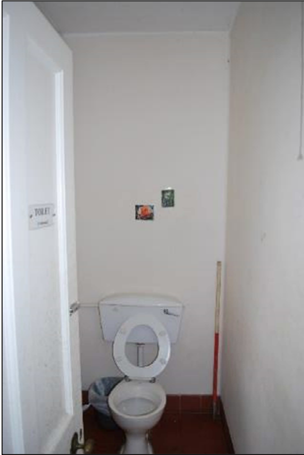
Plate 23 (Shot 134): Ground floor WC, looking northeast, 1m scale
