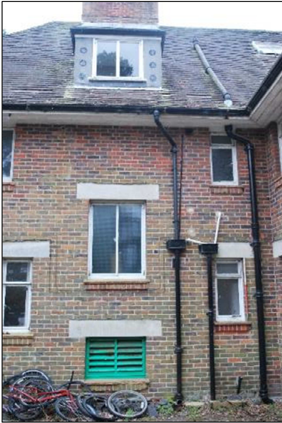
Plate 11 (Shot 20): Southern extent of Elevation D, looking southeast 1m scale
