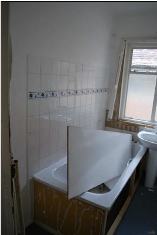
Plate 44 (Shot 385): Bungalow bathroom, looking north, 1m scale
