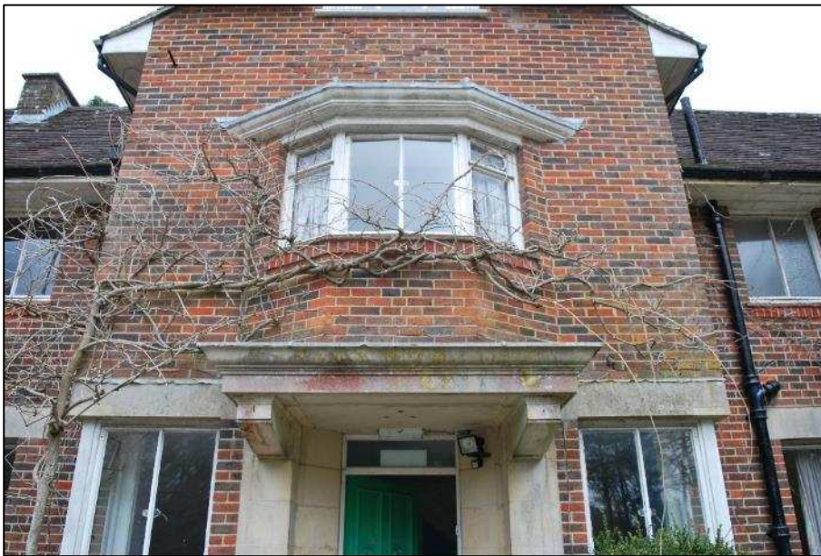
Plate 4 (Shot 80): Bay window above entrance porch, looking northeast
