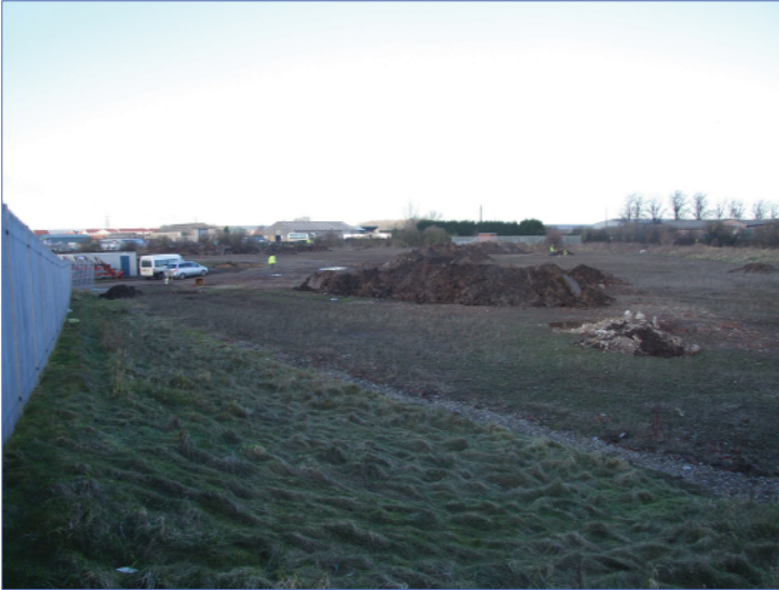
Plate 1: Areas A and B during evaluation. Taken from south-east corner of Area A, looking west
