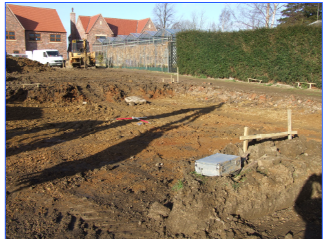
Plate 4: Stripped area at the north-west corner of Plot 11. Looking north-north-west.
