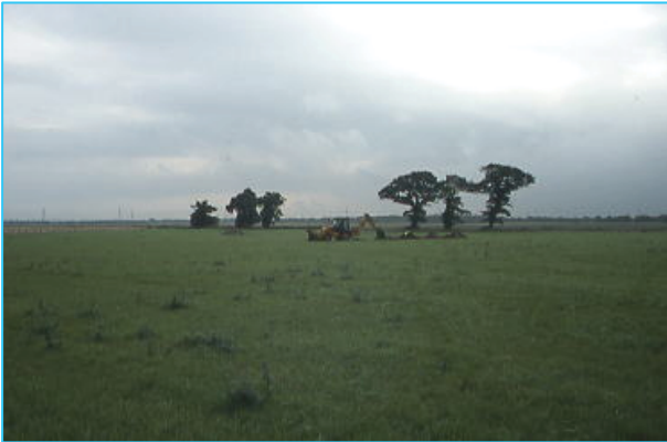
Pl. 1: General view of the development area, looking south-east, during machine excavation of Trench 1.
