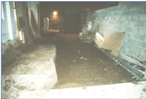
Plate 3: Trench 2, after cleaning, looking south-west.
