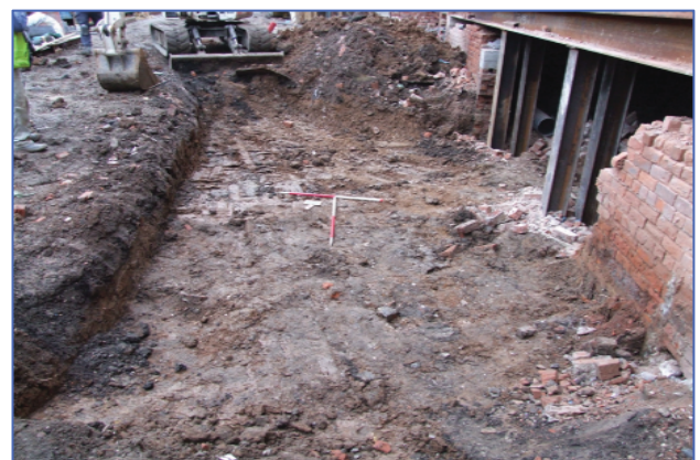
Plate 6: Trench 3, immediately to the east of the Hopper Building. Looking south-east.
