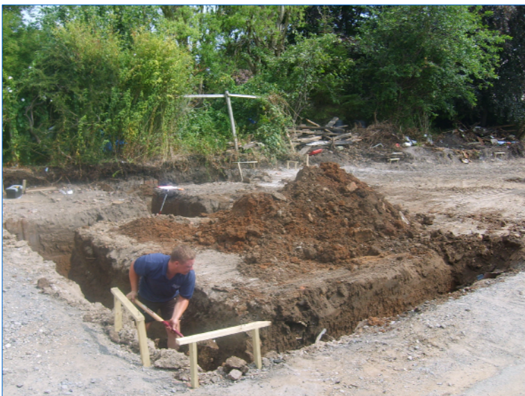
Plate 3: Plot 3 under excavation. Taken from southwest corner of plot, looking northeast.
