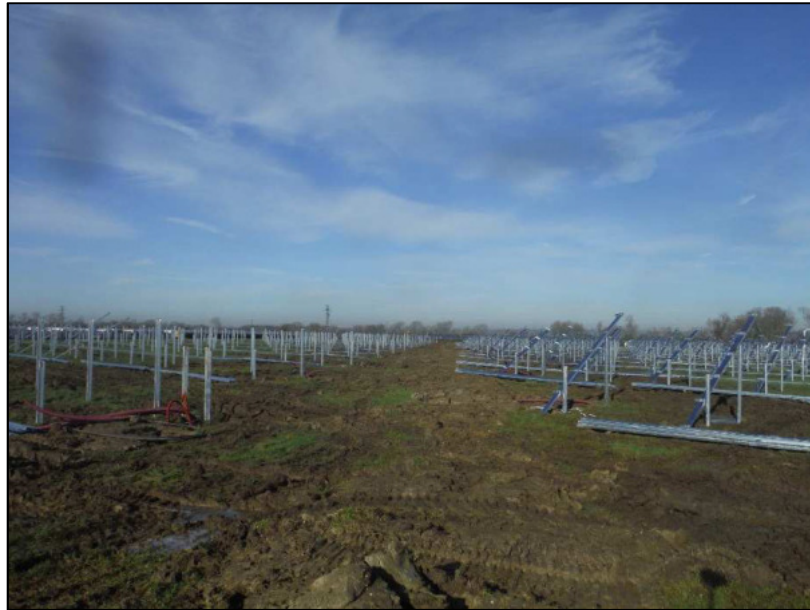
Plate 1: Backfilled Trench 7, looking northwest
