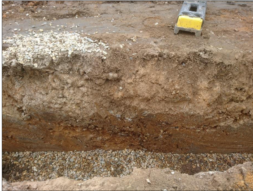
Plate 1: Representative section through service run, looking west
