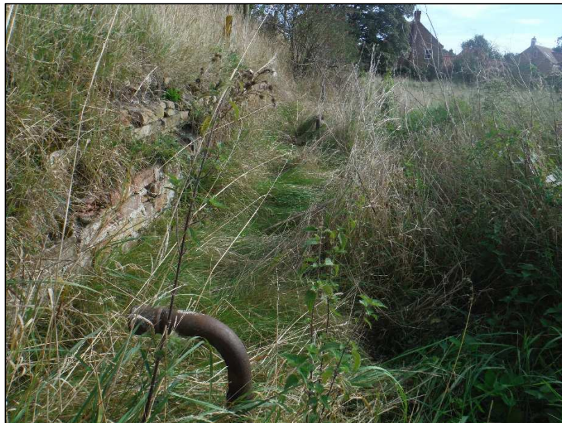
Plate 8: Pipework in-situ between the bank and boundary wall, looking east
