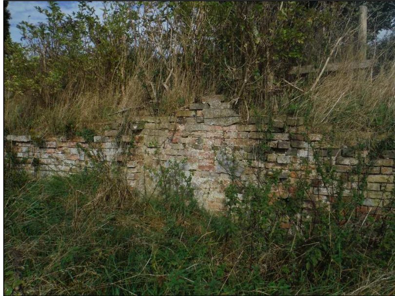
Plate 3: Section of boundary wall showing where internal walls were tied-in, looking northwest
