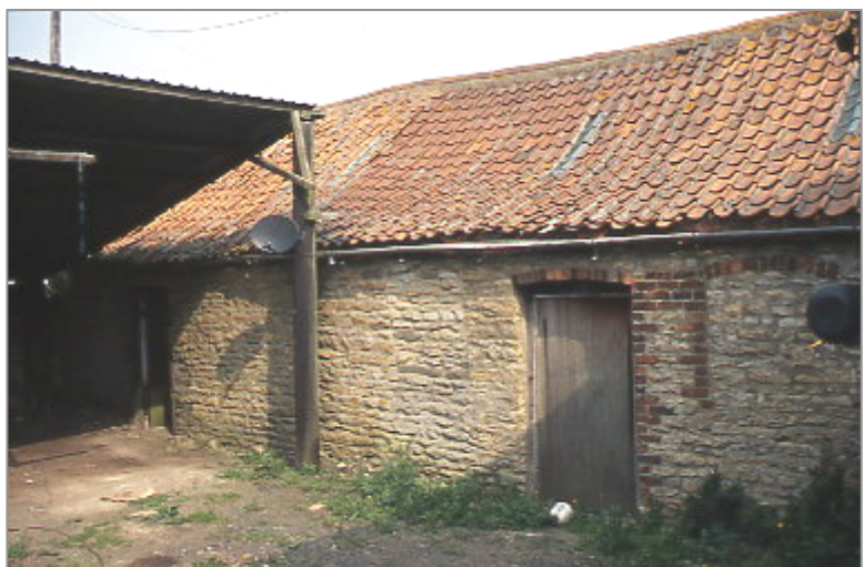
Plate 24: South elevation of Barn 1. Looking north-west, showing the two doors and the blocked windows.
