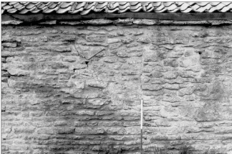
Plate 2: Detail of the north elevation of Barn 1, showing a blocked window and a scar indicating a former X-shaped tie (scale 1m).
