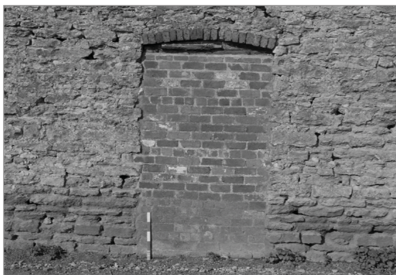
Plate 5: Detail showing blocked doorway in the east elevation of Barn 2. Looking west (scale 0.5m)
