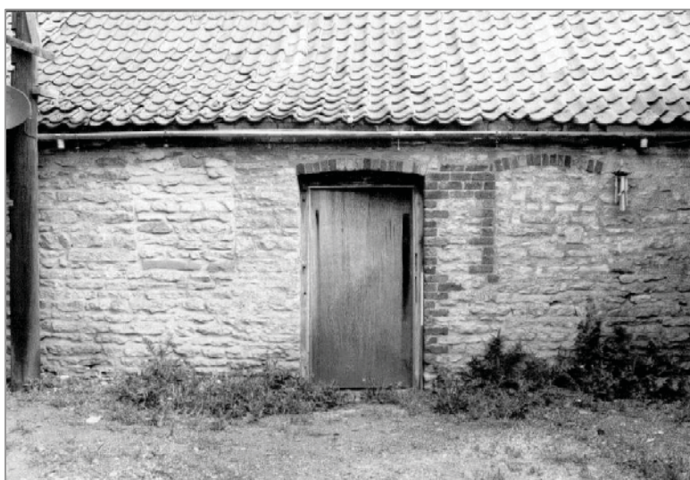
Plate 8: Detail of door and blocked windows in south elevation of Barn 1, looking north (scale 1m).
