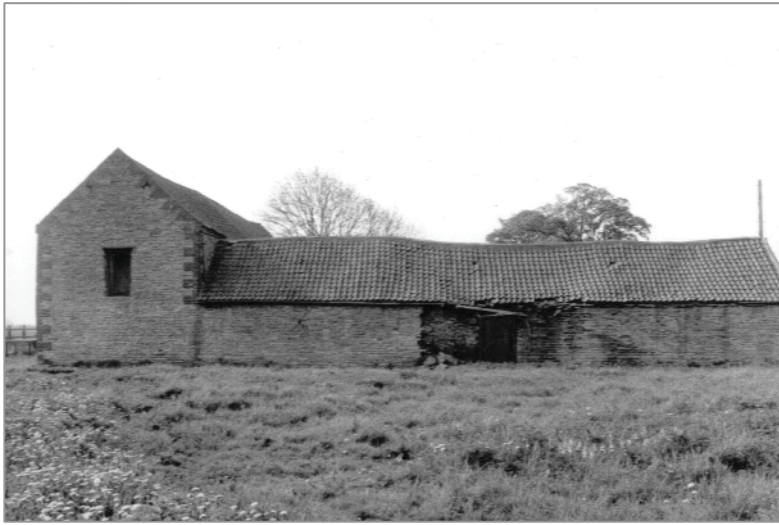
Plate 1: Northern elevation, looking south, showing the area of collapse around the central door of Barn 1, and the northern gable end of Barn 2.
