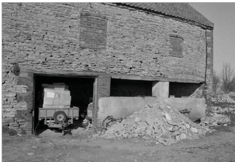
Plate 4: Detail showing the three bay opening (possible former cartshed) at the north end of Barn 2. Looking north-east.
