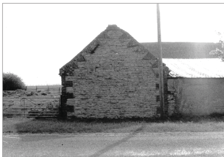
Plate 6: Western gable end of Barn 1 fronting South Cliff Road. Note the brick sawtooth quoins and tumbling. Looking east.
