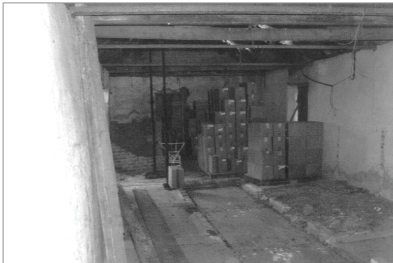
Plate 11: General view of large room at the west end of Barn 1. Looking east-south-east from the north-west corner. The brick foundations of the pig sties are clearly visible as are the wooden and steel tie beams in the roof.
