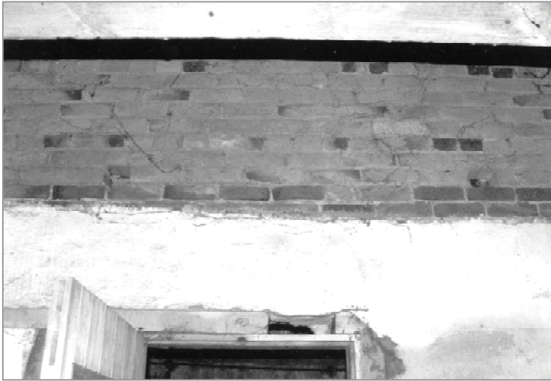
Plate 13: Detail showing the brickwork of the dividing wall between the two rooms at the east end of Barn 1, looking east. A number of 'airholes' are also visible.
