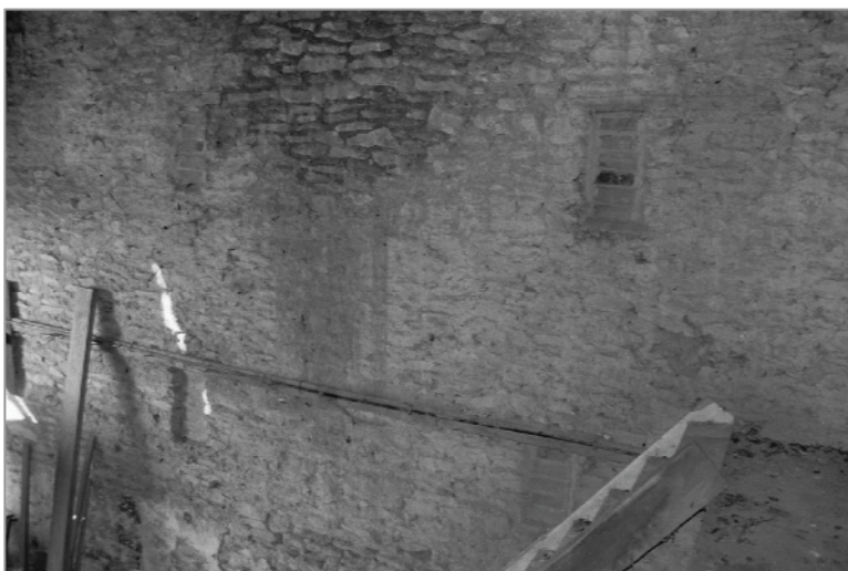
Plate 18: Interior east elevation of Barn 2, showing blocked ventilation holes. Looking south-west.
