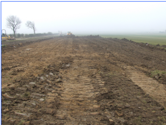
Plate 3: The stripped area of the north-eastern chicken shed, looking west-south-west.
