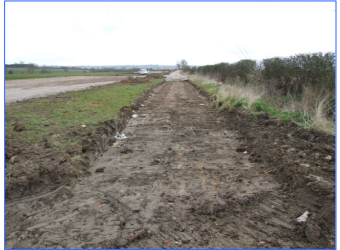
Plate 2: The access road running along the north side of the existing field boundary, looking east-north-east from the eastern end of the development area.
