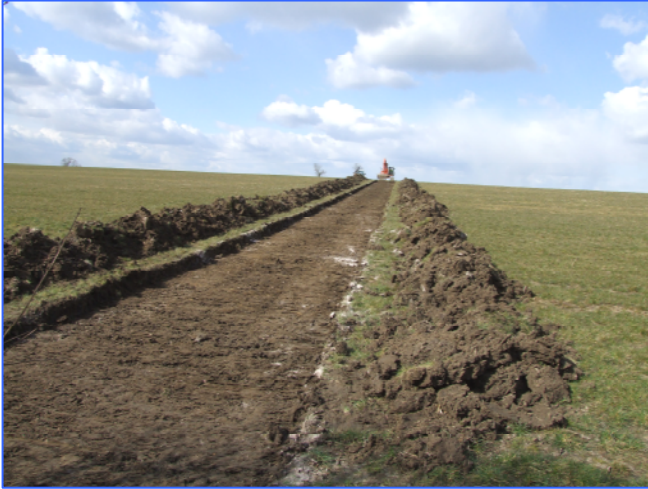
Plate 1: The access road during machine stripping, looking north-north-west from Moor Road.
