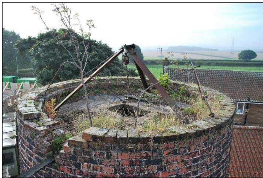
Plate 4 (Shot 1): The top of the windmill, looking southeast
