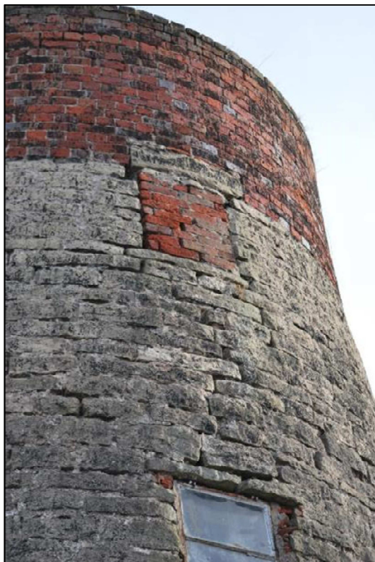
Plate 8 (Shot 24): Blocked second floor window, looking east
