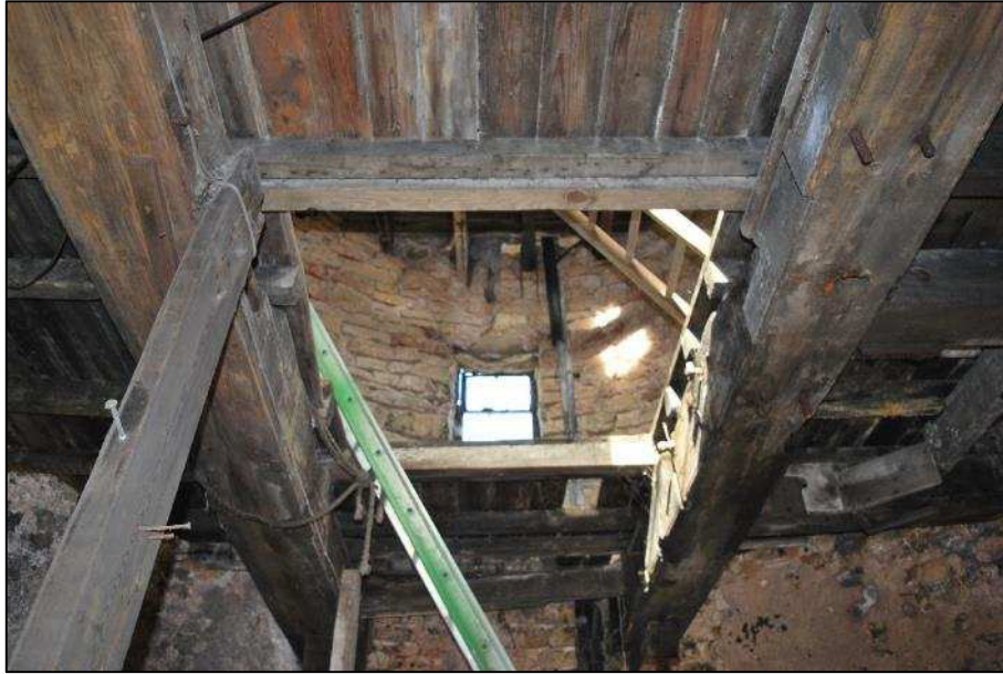
Plate 21 (Shot 71): Various additional supports to the first floor, looking northwest
