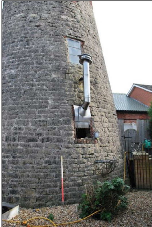
Plate 7 (Shot 23): Southwestern ground and first floor windows, looking east (1m scale)
