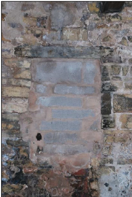
Plate 14 (Shot 64): Ground floor window bricked up from the interior, looking northeast
