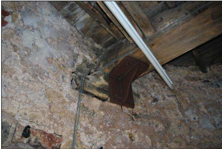
Plate 20 (Shot 72): Principal beam recessed into the wall, looking southeast
