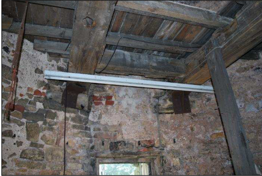
Plate 19 (Shot 68): Ceiling support; beams supporting joists and planks, looking southeast
