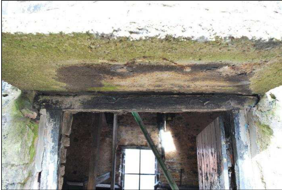
Plate 9 (Shot 37): Detail of the concrete porch and wooden door frame, looking northwest
