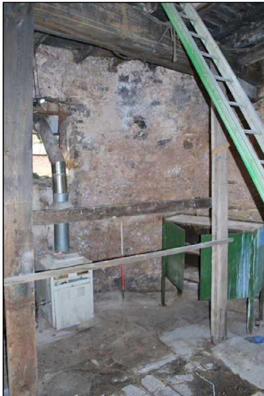
Plate 16 (Shot 76): Supports added to the principal beams, looking west (1m scale)
