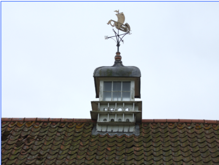
Plate 14: The glazed cupola on the roof of the three storey barn, with the wind vane and flight holes for pigeons. Looking south-south-east.
