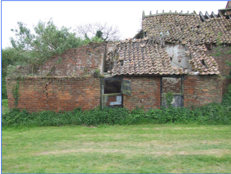
Plate 4: Stable block and cartshed at the east end of the north elevation of the north range. Looking south-south-east.
