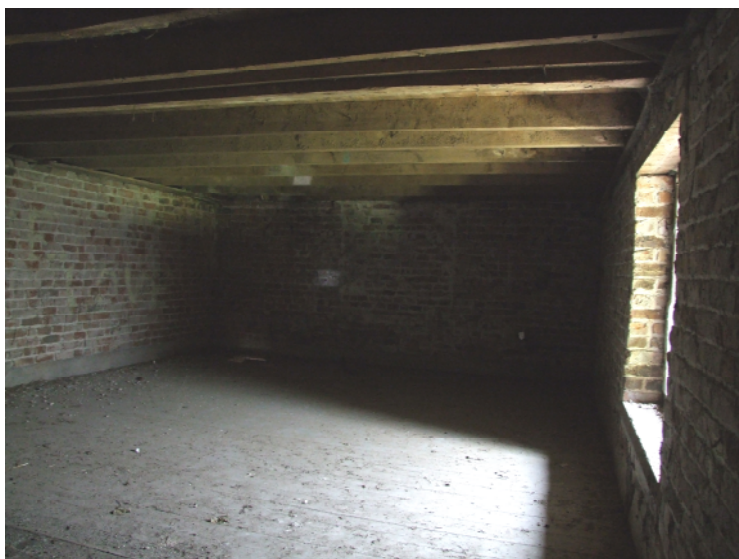
Plate 12: First floor of the threshing barn, looking west.
