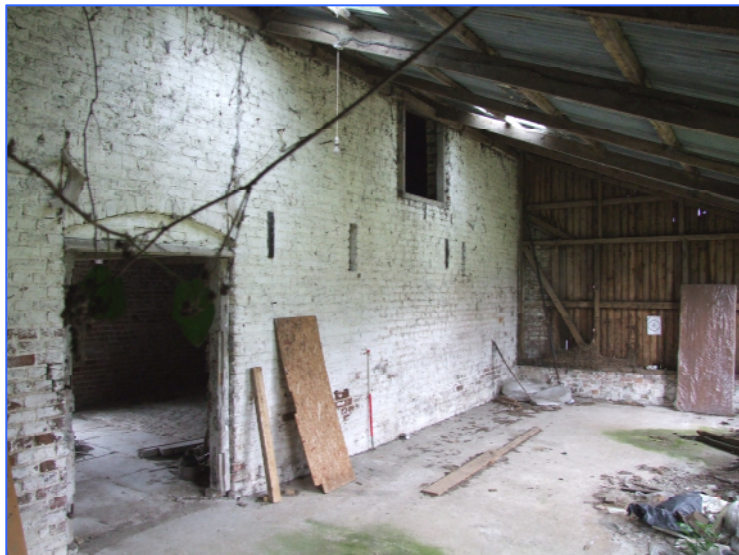
Plate 10: Interior of lean-to on north elevation of north range, showing the door and pitching hole in the north elevation of the barn.
