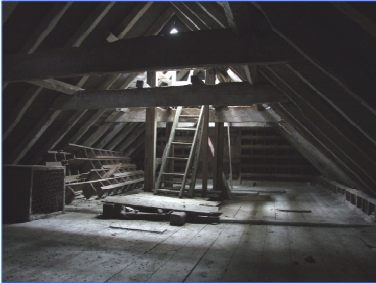
Plate 13: Pigeon cote in the second storey of the threshing barn. Note the pigeon holes at the far end of the room and along the right hand side of the shot, and the ladder allowing access to the cupola above. Looking west.
