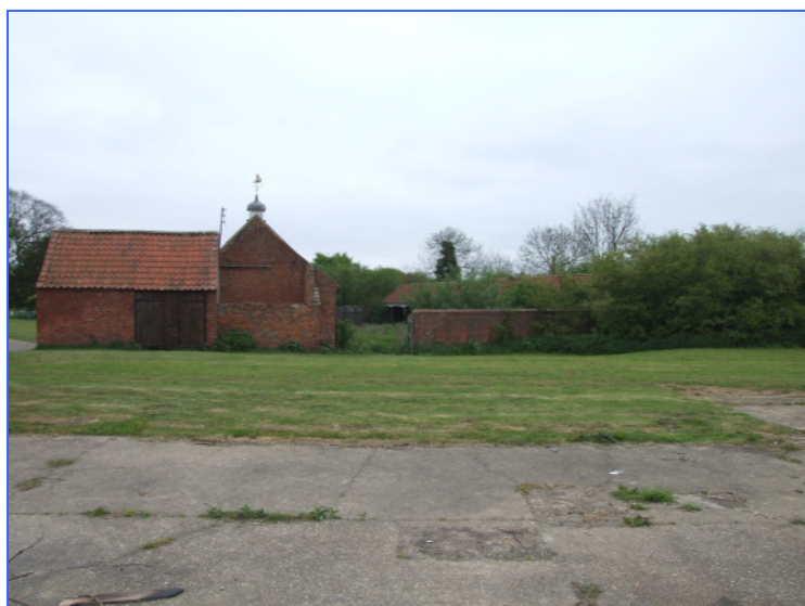
Plate 27: West elevation of the barns, showing the outbuildings at the end of the north range and the boundary wall attached to the south range, with the gates between. Looking east-north-east
