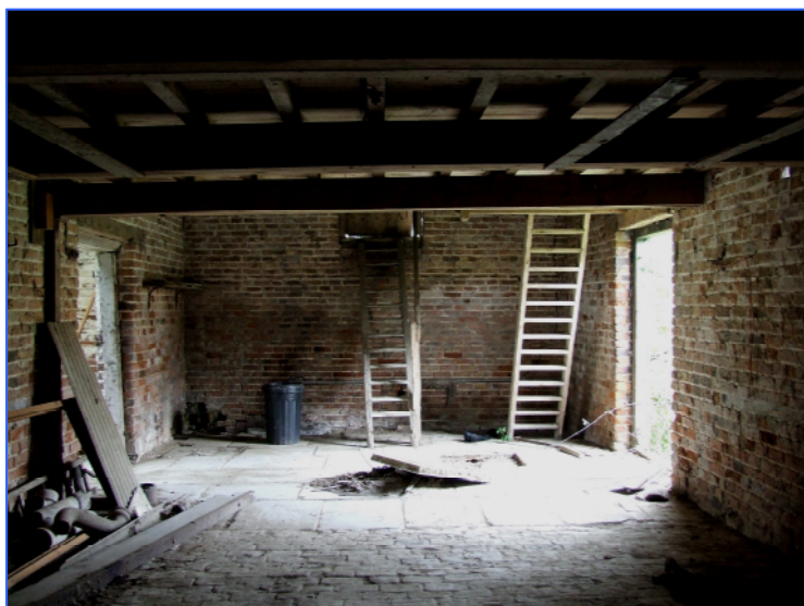
Plate 11: Ground floor of the threshing barn, looking east-north-east towards the flagstone threshing floor, with the large doors at either side allowing the through-flow of air to carry away the chaff.
