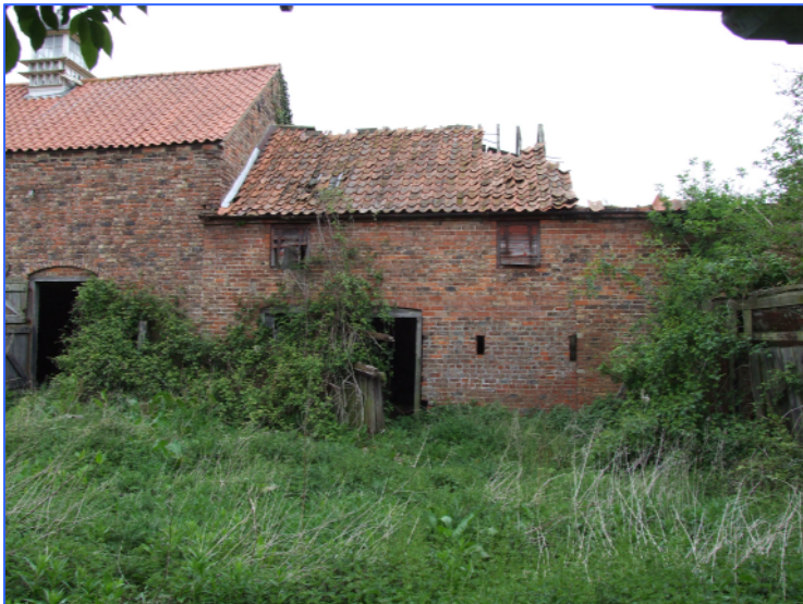
Plate 5: Stable block and hayloft in the south elevation of the north range. Looking north-north-west.
