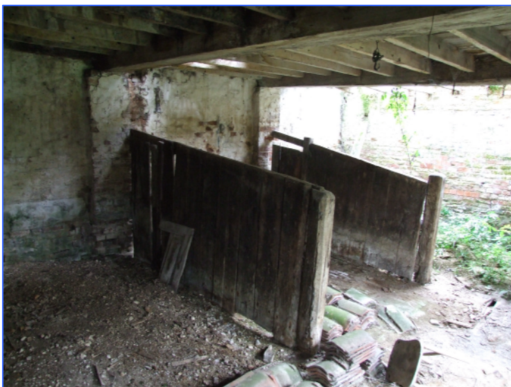
Plate 6: Interior of the stable block, showing the wooden partitions. Looking north-north-east.
