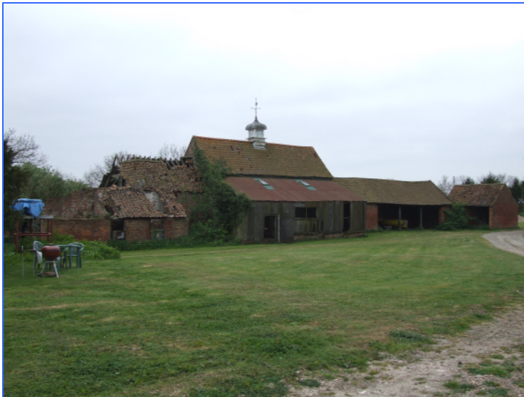
Plate 2: The north elevation of the north range, looking south.
