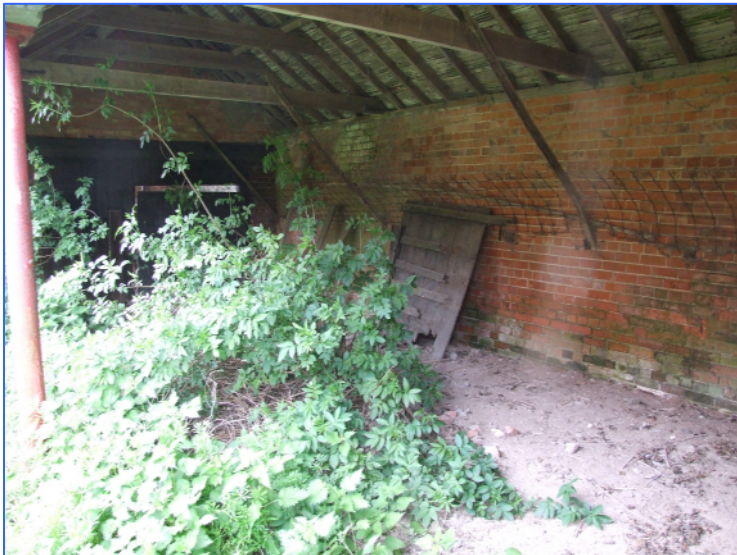
Plate 23: Interior of the eastern bay in the south range, with the feeding rack along the south wall. Looking east
