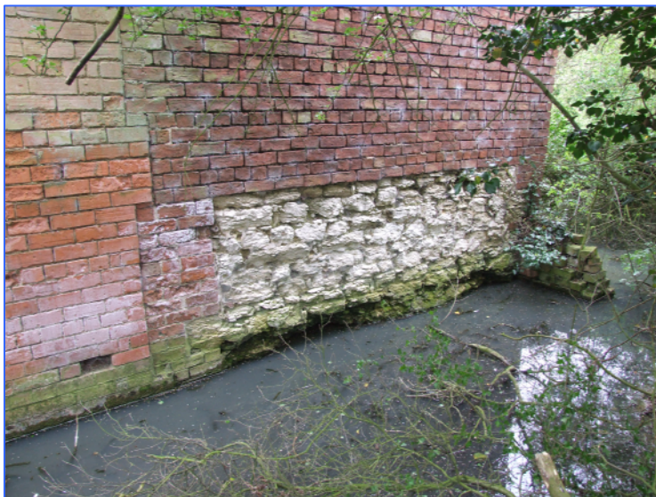
Plate 21: Chalk blocks in the south-east corner of the south range. Looking north. Note also the difference in brickwork at the left of the shot.
