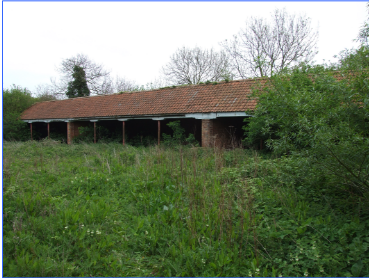
Plate 22: North elevation of the south range, looking east.
