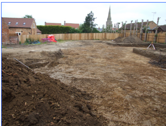
Plate 1: General view of the development area after topsoil stripping, looking east-south-east.
