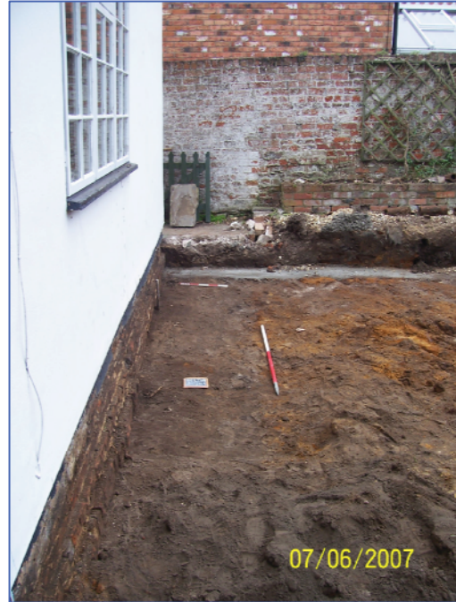
Plate 2: Foundation trench [102] exposed in plan. Looking east-north-east.
