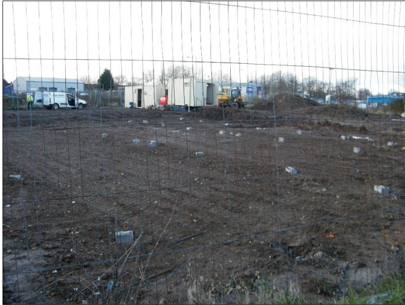
Plate 1: View across site showing pile locations, looking southeast
