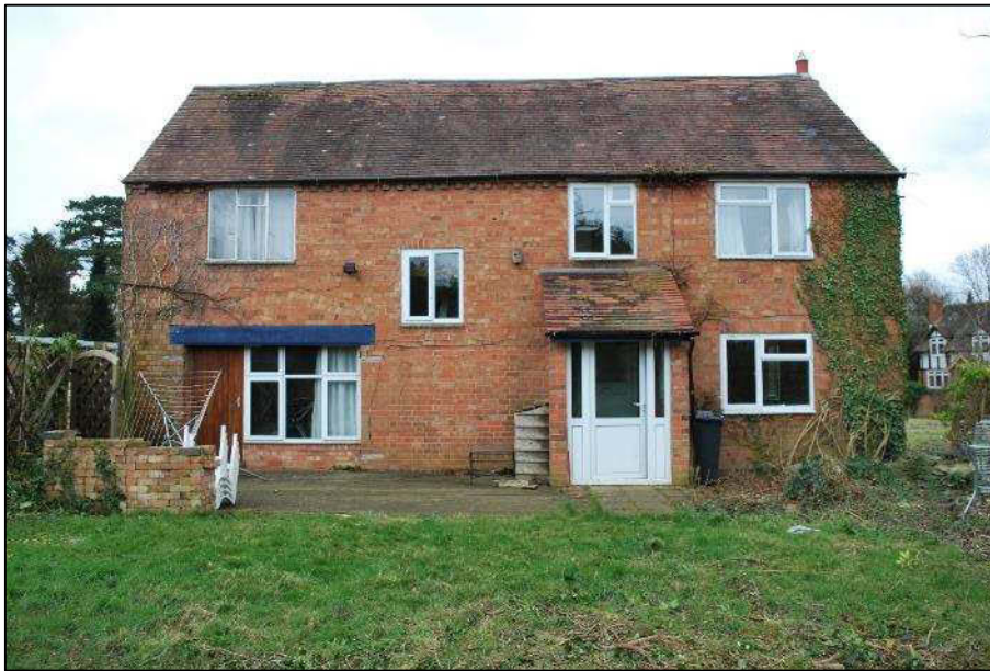
Plate 1 (Shot 57): Southwest elevation, looking east-northeast (1m scale)
