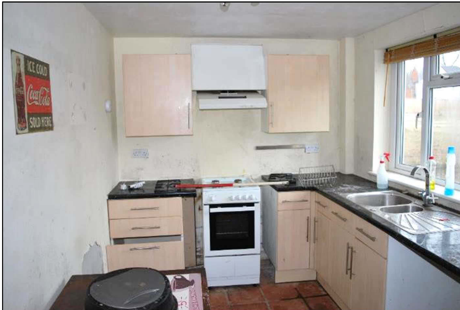
Plate 14 (Shot 41): Kitchen, looking north-northwest (1m scale)
