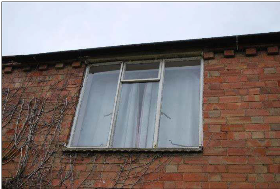
Plate 4 (Shot 63): Window above garage door, looking northeast
