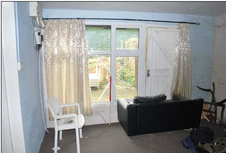
Plate 16 (Shot 36): Bedroom 1, looking west (1m scale)
