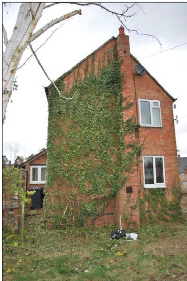
Plate 6 (Shot 69): Southeast elevation, looking north (1m scale)
