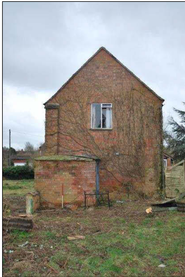
Plate 8 (Shot 76): Northwest elevation, looking south-southeast (1m scale)
