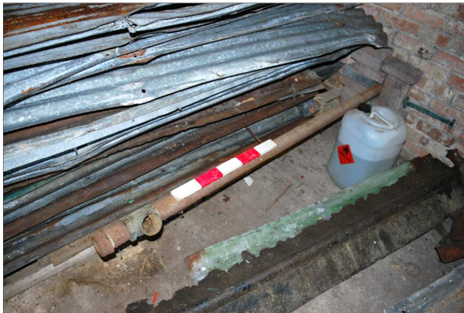
Plate 12 (Shot 17): Pipe extending from eastern elevation, looking northeast (0.5m scale)
