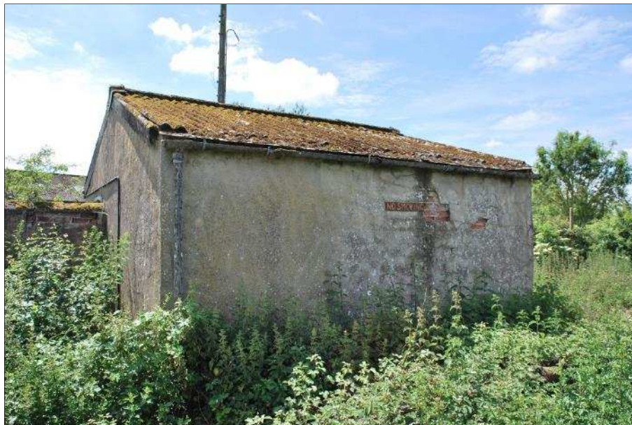
Plate 1 (Shot 27): North elevation of pumping station, looking southwest
