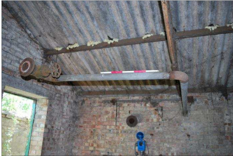
Plate 11 (Shot 18): Pipe extending from southern elevation, looking south (0.5m scale)
