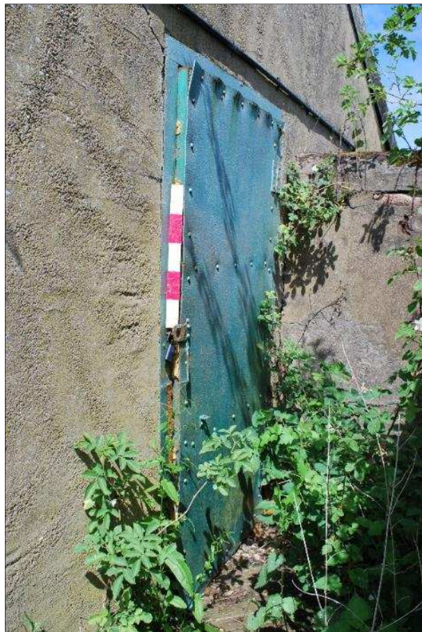
Plate 3 (Shot 5): Steel door on east elevation, looking northwest (0.5m scale)
