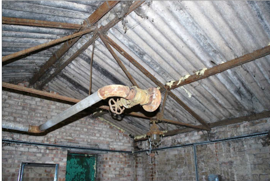
Plate 8 (Shot 13): Metal roof truss and pipework, looking northwest
