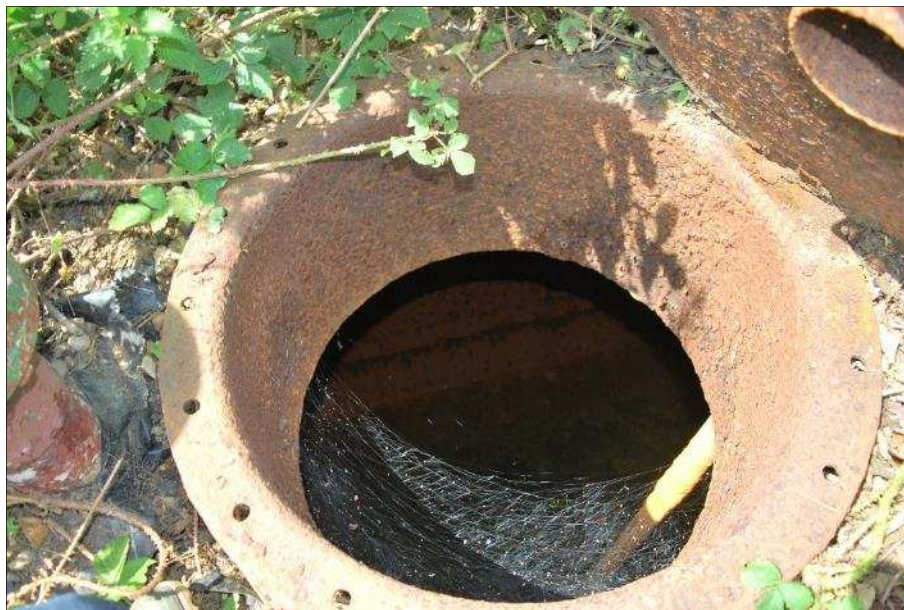
Plate 16: (Shot 47): Circular access shaft into subterranean fuel tank, looking northwest
