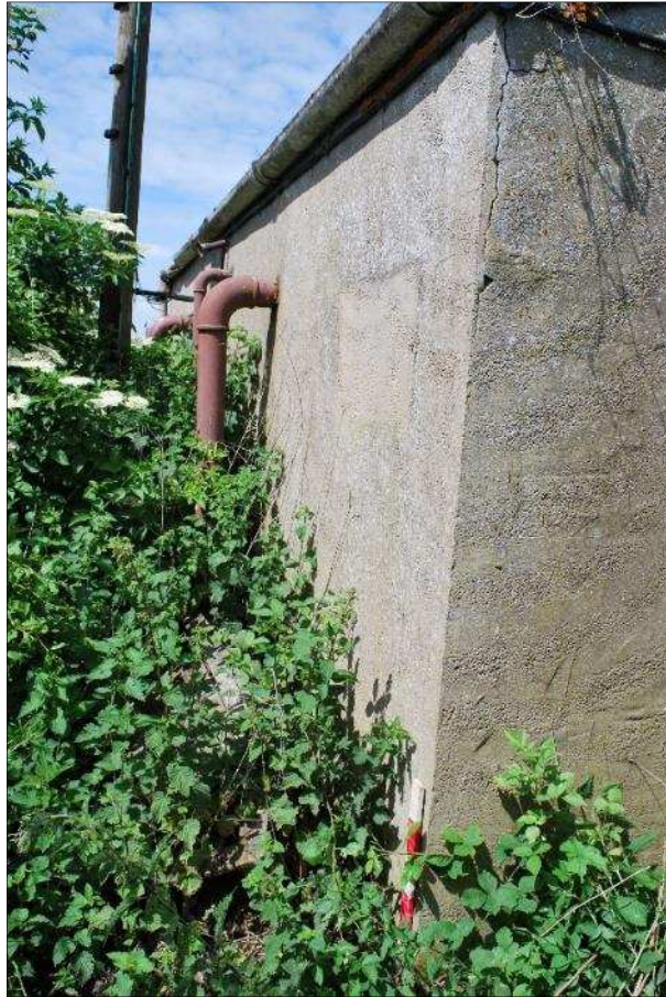
Plate 6 (Shot 3): External pipework on south elevation, looking west (0.5m scale)
