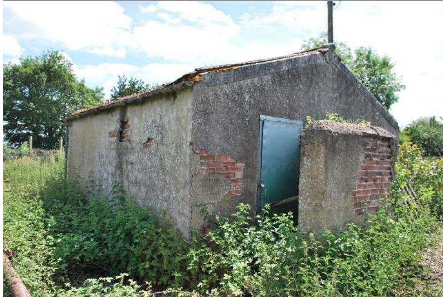
Plate 4 (Shot 28): West and north elevations, looking southeast
