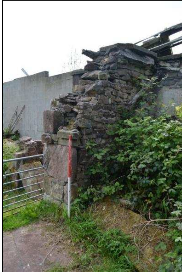
Plate 70 (Shot 112): West part of Building 8, looking southeast (1m scale)
