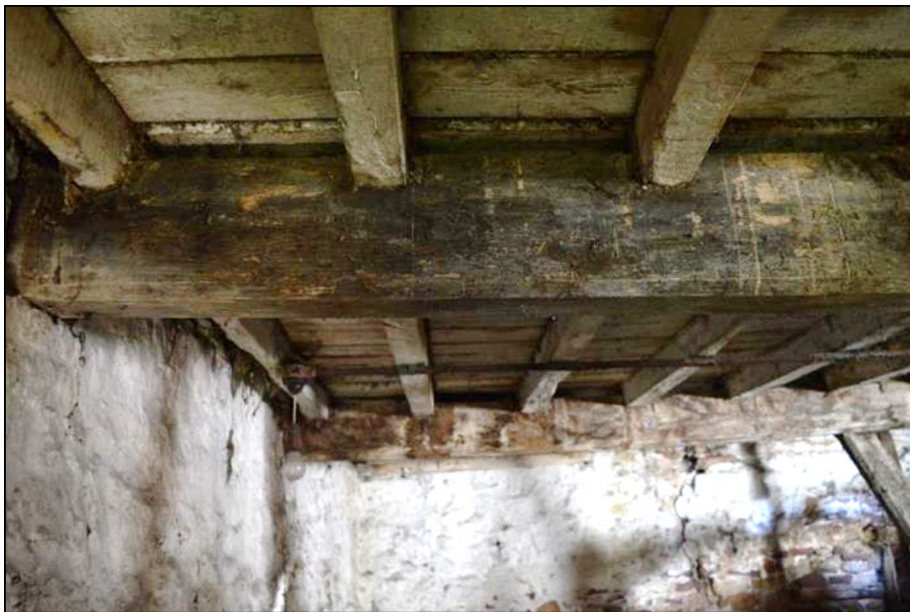
Plate 43 (Shot 65): Interior detail Room 1b (Building 1), ceiling structure, looking north
