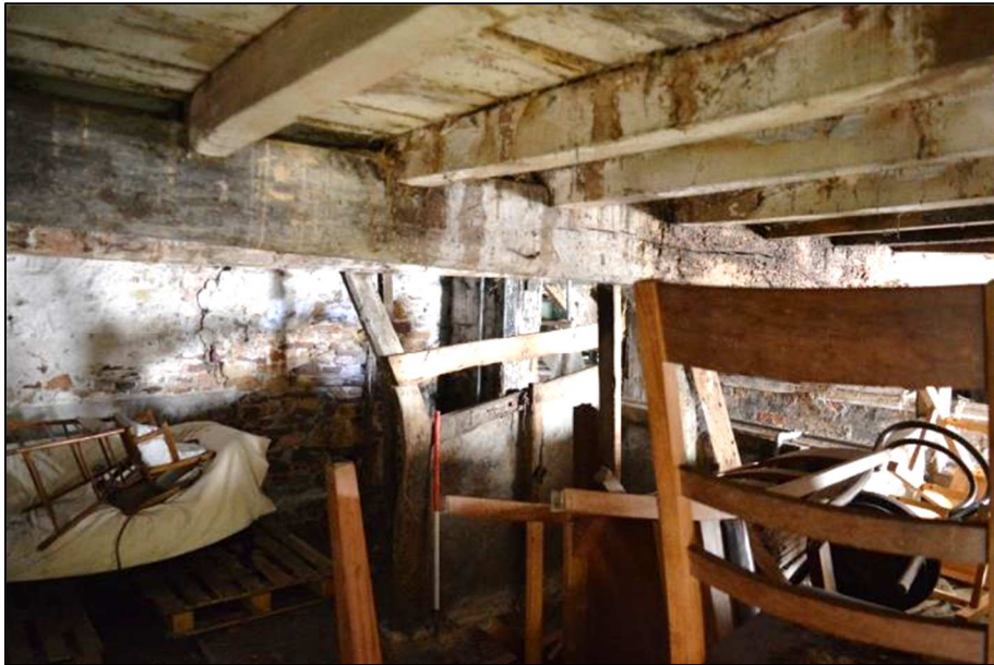
Plate 40 (Shot 64): Interior view of animal accommodation in Room 1b showing wood and stone slab stalls, looking northeast (1m scale)
