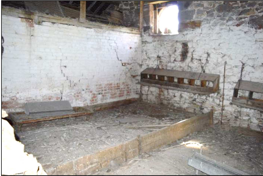
Plate 53 (Shot 72): Interior of Room 1d, showing nest boxes, pitching hole, brick partition wall, wood plank flooring and low wood plank partition, looking southeast
