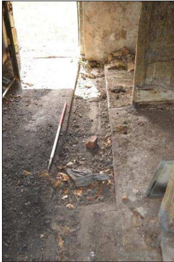
Plate 46 (Shot 130): Interior ground floor animal accommodation (Room 1c) showing manuring gully between manuring and access passage and stalls, looking south (1m scale)
