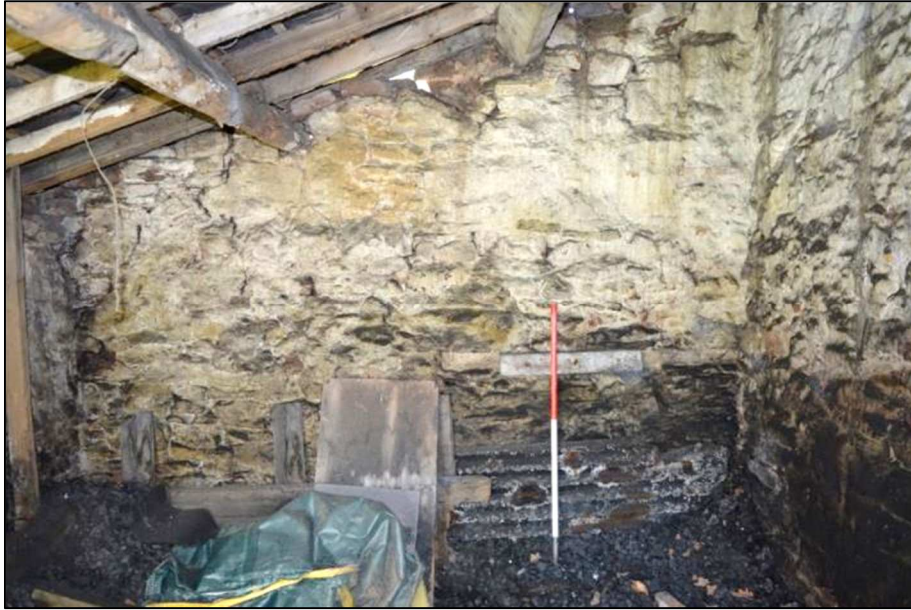
Plate 73 (Shot 117): Interior of lean-to Building 9, looking east (1m scale)
