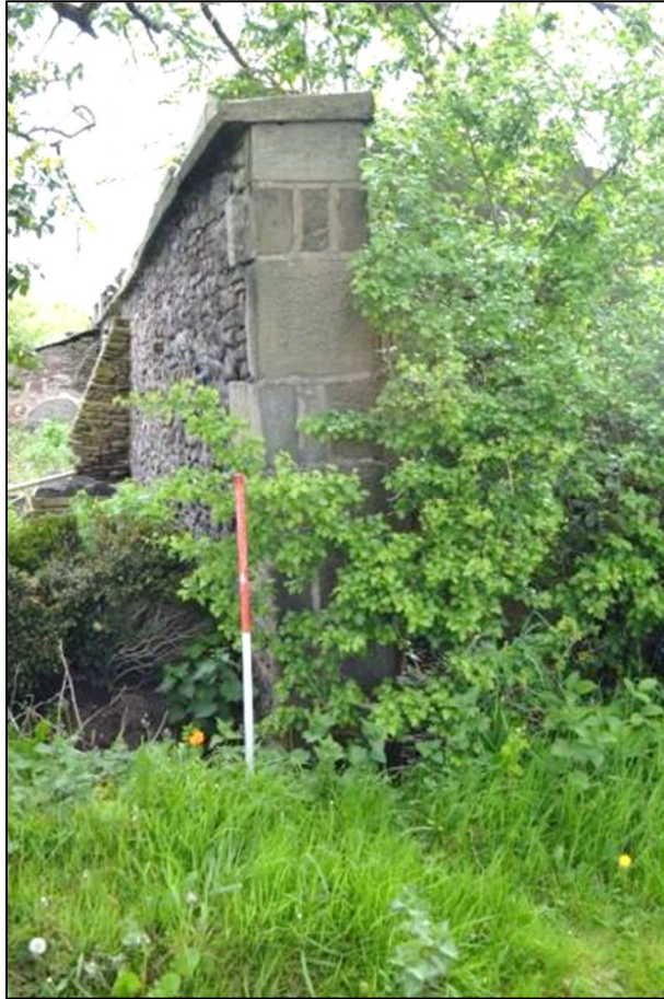
Plate 68 (Shot 120): West end of Wall 7, looking east (1m scale)
