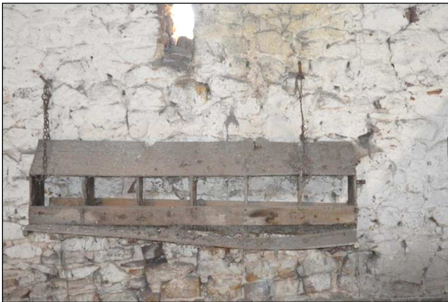
Plate 54 (Shot 74): Interior of Room 1d, detail of nest boxes attached to south wall, looking south
