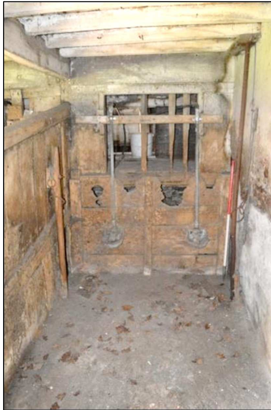
Plate 49 (Shot 126): Interior of animal accommodation at south east corner of barn (Building 1, Room 1c) showing double wooden stall with tethering posts, rings and drinkers and opening through to feeding passage to west, looking west (1m scale)
