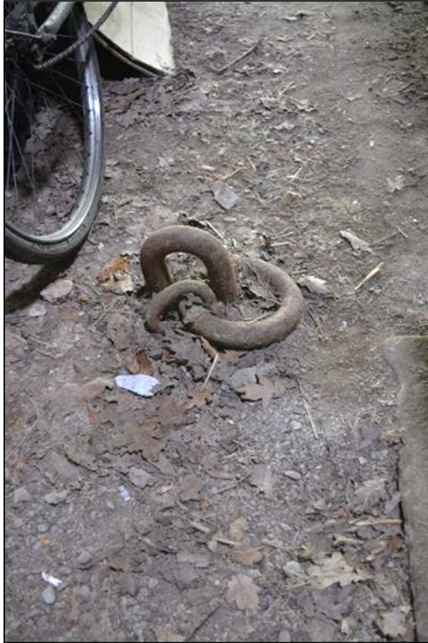
Plate 35 (Shot 56): Barn (Building 1, Room 1a) detail showing iron rings attached to floor near western double doors, looking west
