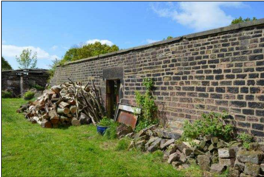
Plate 66 (Shot 104): Wall 6, looking southwest
