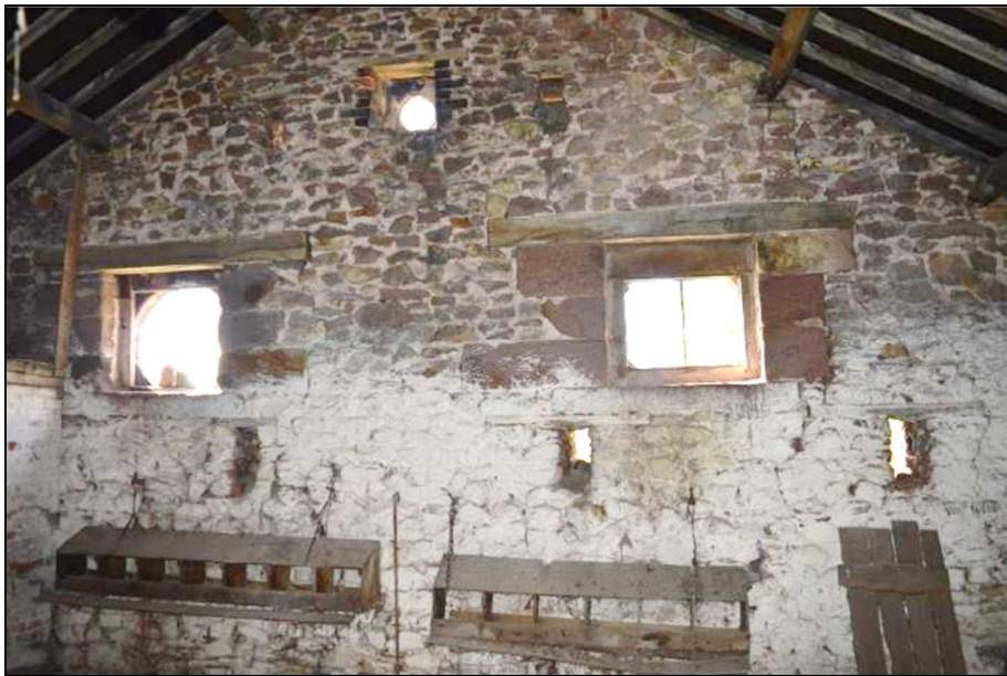
Plate 22 (Shot 70): Interior first floor of barn, south gable end including owl hole, two pitching holes and breather slits. Also, wooden nest boxes attached to wall, looking south
