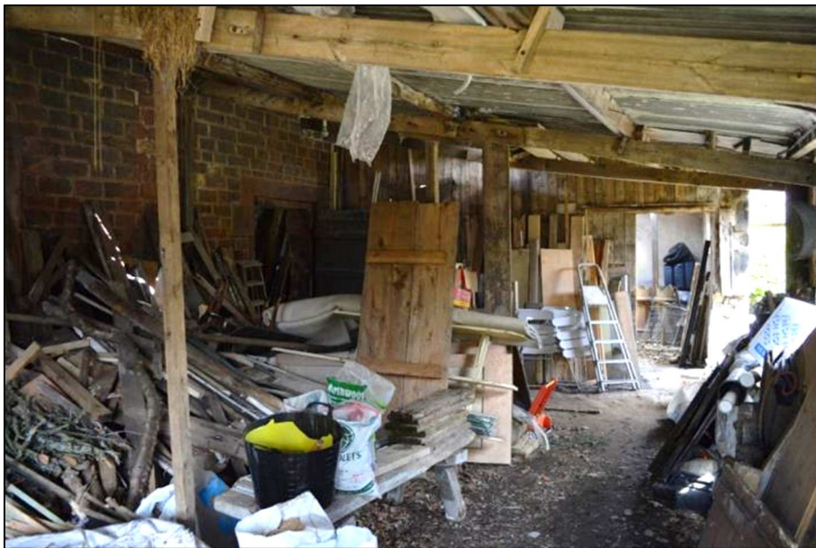
Plate 62 (Shot 93): General view of interior of lean-to Building 4, looking north towards Building 3 (1m scale)
