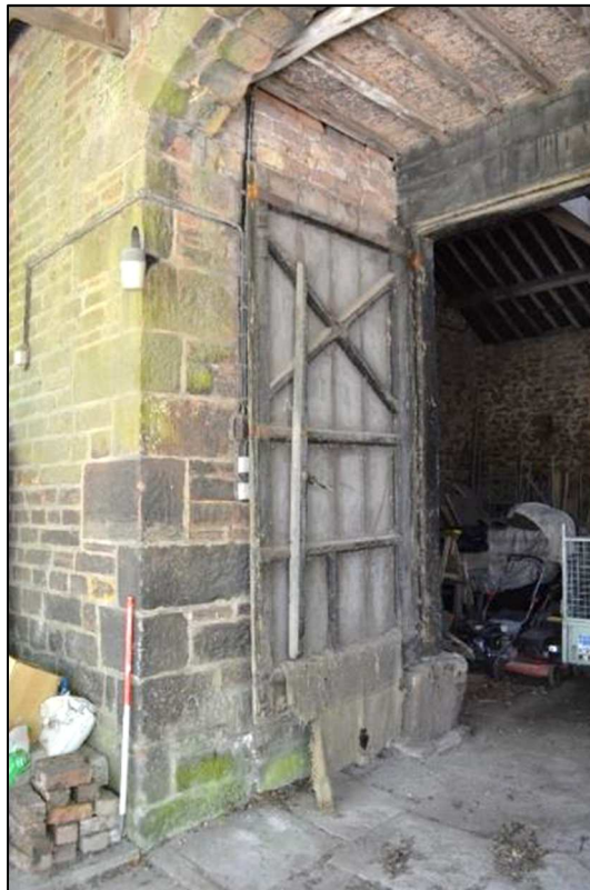
Plate 11 (Shot 37): Detail of entrance at west side of barn (Building 1) including stone and wood internal porch, wooden door and carved stone to accept threshold (1m scale)
