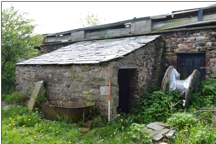
Plate 69 (Shot 113): Lean-to Building 9 and adjoining Wall 7, looking southeast (1m scale)
