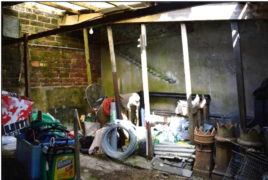
Plate 59 (Shot 94): Interior of lean-to Building 3, including detail of stepped projecting stonework of north wall for former eaves, looking northwest (1m scale)
