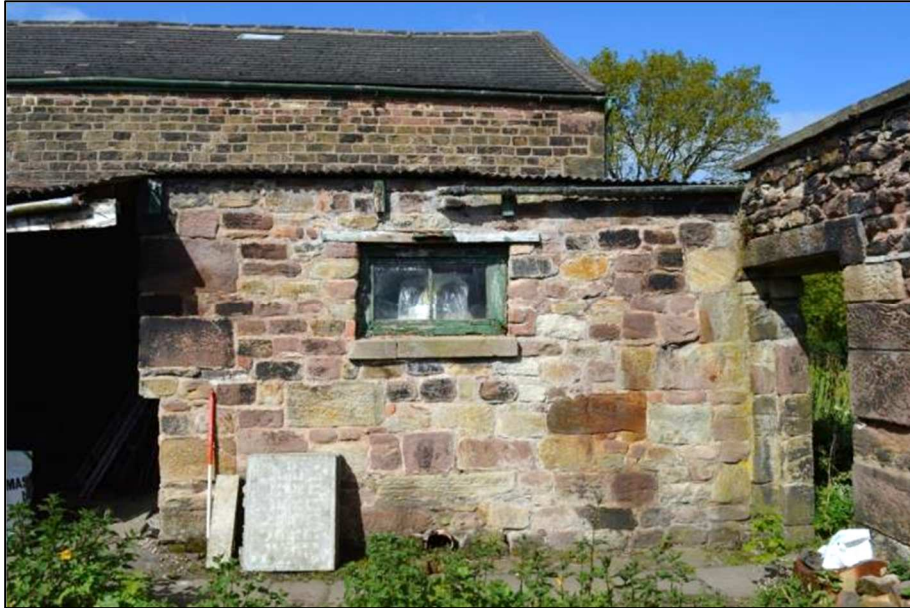
Plate 58 (Shot 15): East elevation of Building 3, looking west (1m scale)
