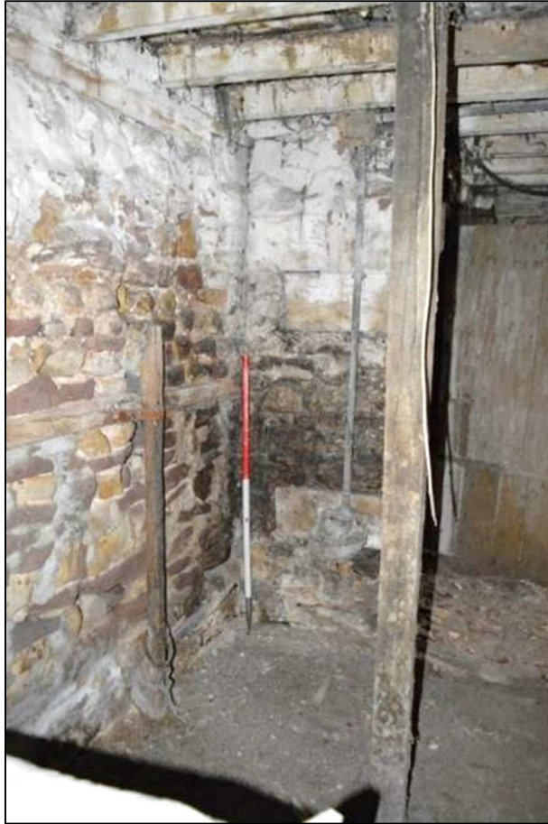
Plate 42 (Shot 69): Interior of barn (Building 1) showing tethering post and ring alongside drinker at northeast corner of Room 1b, looking east (1m scale)
