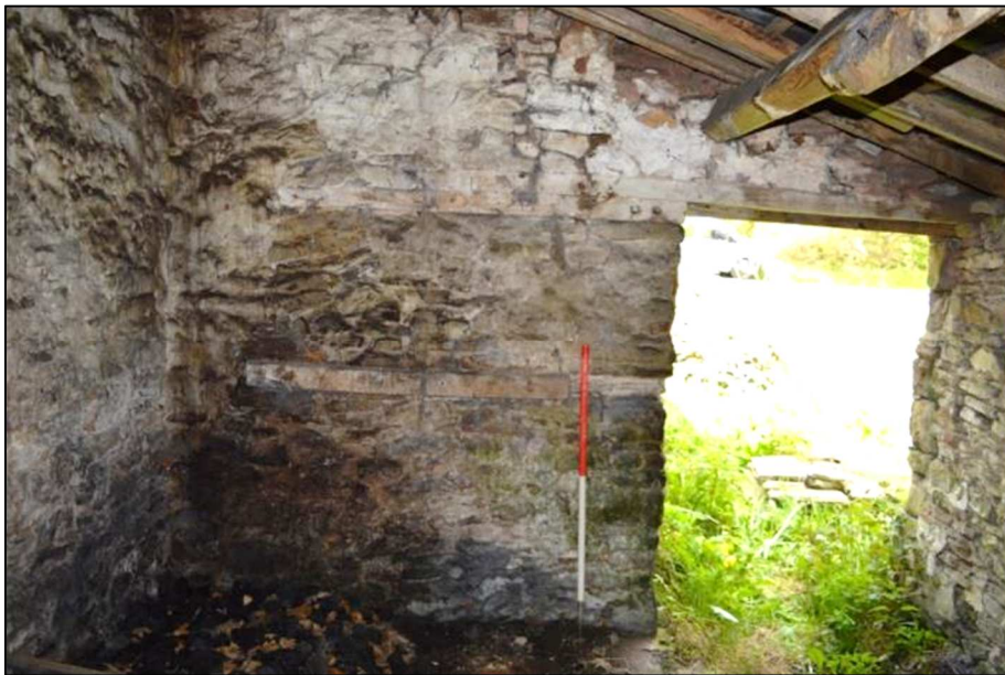
Plate 74 (Shot 118): Interior of Building 9, looking west (1m scale)
