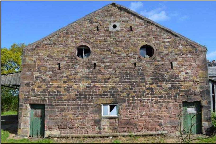
Plate 2 (Shot 3): South elevation of barn (Building 1) looking north (1m scale)
