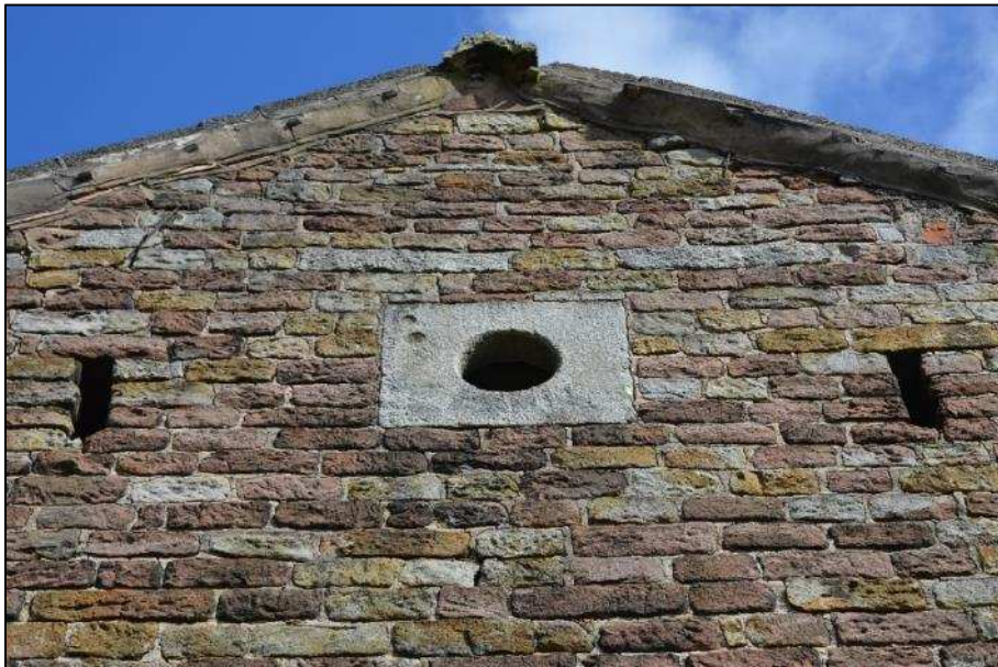
Plate 4 (Shot 8): Detail of south elevation of barn (Building 1), showing owl hole, breather slits and eaves, looking north
