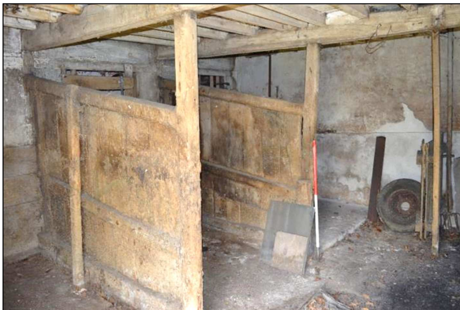
Plate 48 (Shot 125): Interior of ground floor animal accommodation at southeast corner of Room 1c showing wooden stalls and tethering post, looking northwest (1m scale)
