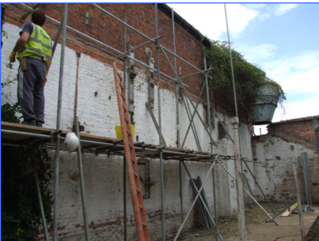
Plate 6: East elevation, looking north-north-west. Note the small chimney and the metal funnel at the north end of the elevation.
