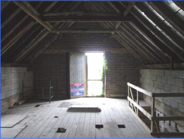
Plate 13: North end of the second floor, looking north to the door and repaired north wall.
