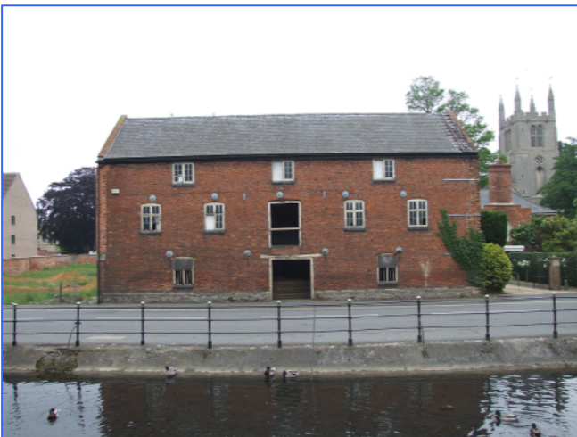
Plate 2: West elevation, looking east.
