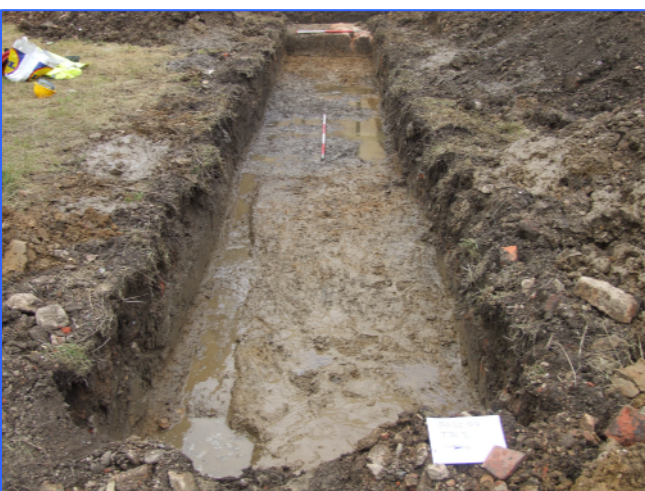
Plate 3: Trench 2, looking west
