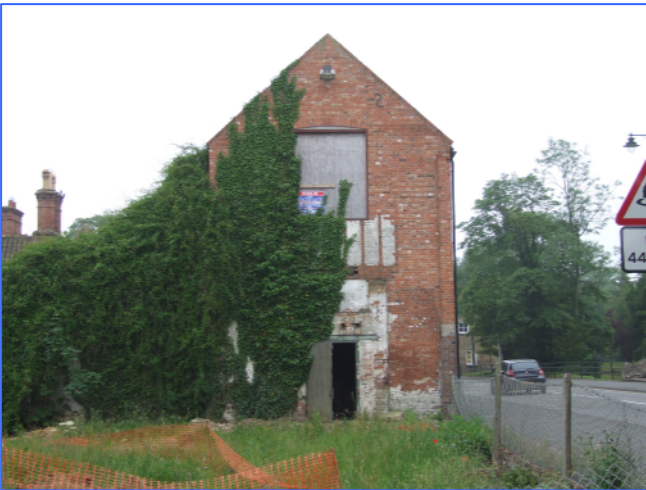
Plate 5: North elevation, looking south
