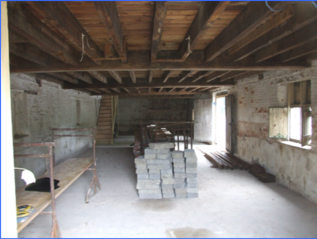
Plate 7: Ground floor of the building, looking south.
