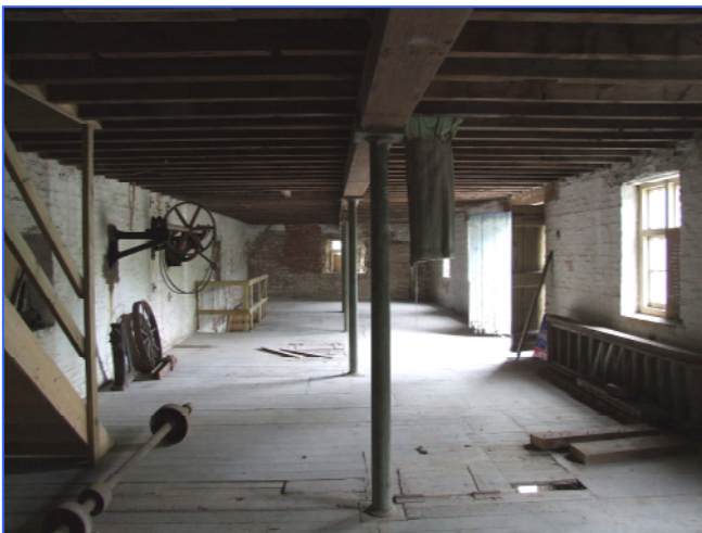
Plate 8: First floor, looking south. The in situ mill machinery is visible to the left of the shot, with the cloth grain chute over a hatch in the foreground.
