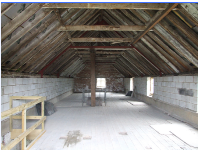
Plate 12: Second floor, looking south
