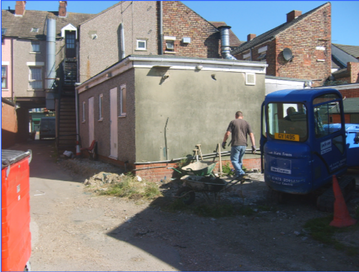
Plate 1: General view of the site, looking north.
