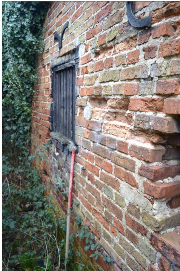
Plate 6 (shot 12): Window on the southwest elevation. Looking northwest, 1m scale
