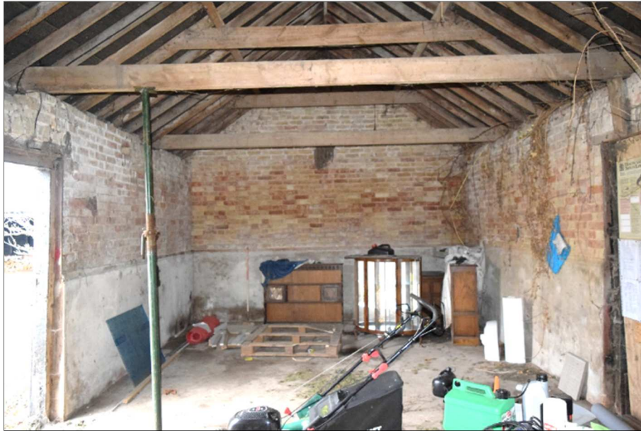
Plate 23 (shot 31): General view of the barn. Looking southeast, 1m scale
