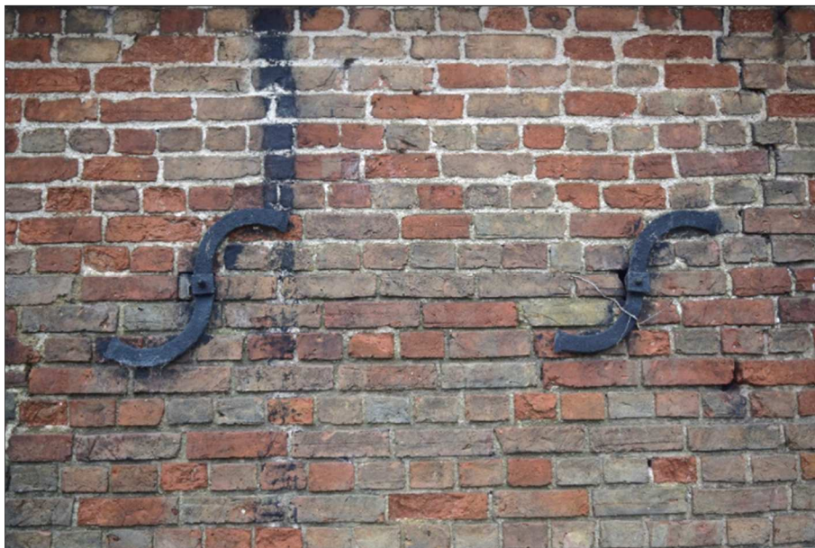
Plate 4 (shot 10): S-shaped tie plates on southwest elevation. Looking south
