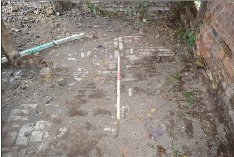
Plate 15 (shot 22): Representative view of brick floor. Looking southeast, 1m scale
