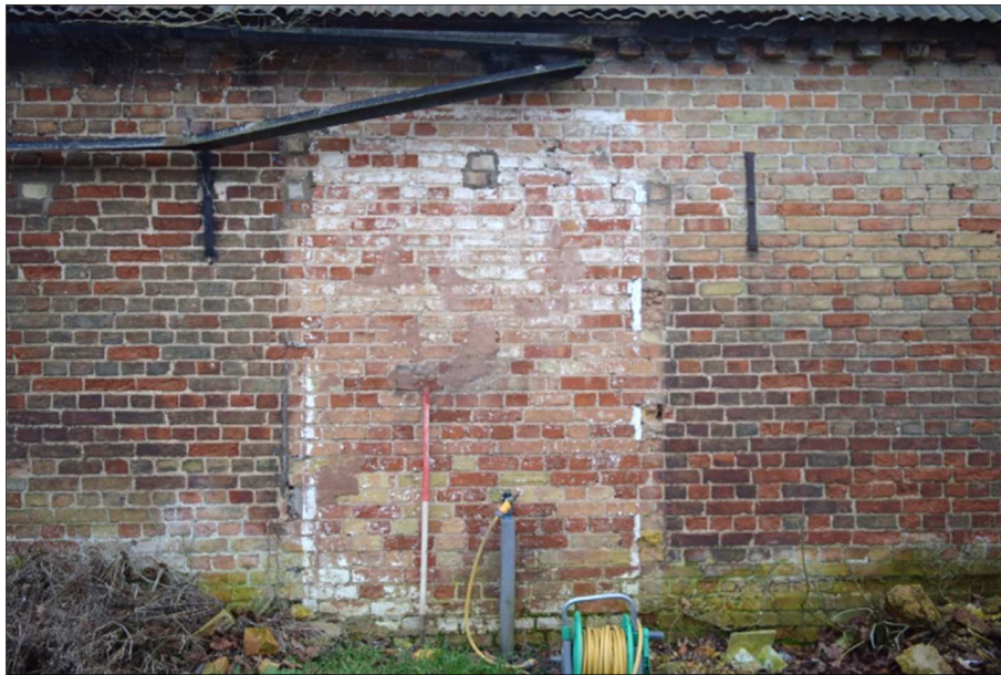
Plate 3 (shot 27): Bricked-up opening on northeast elevation. Looking south, 1m scale
