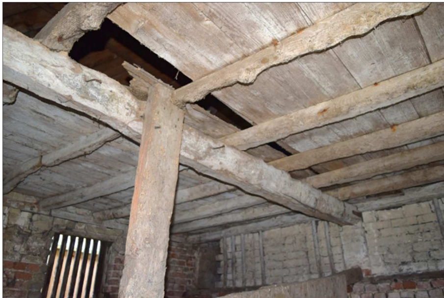
Plate 14 (shot 18): Ceiling and loft floor joists. Looking southwest
