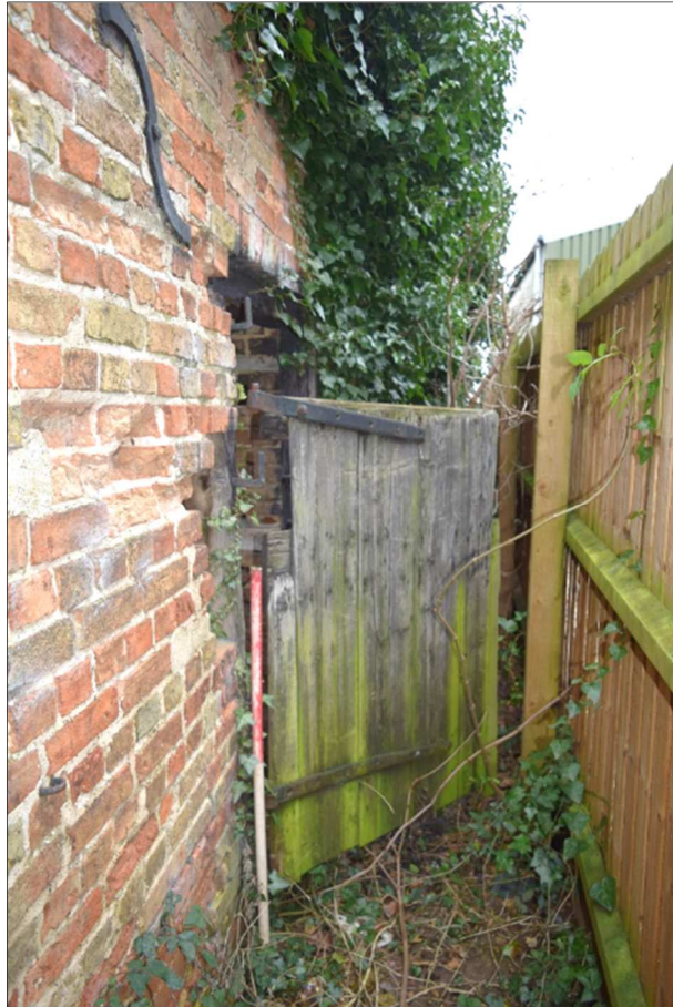
Plate 7 (shot 13): Door on southwest elevation. Looking southeast, 1m scale
