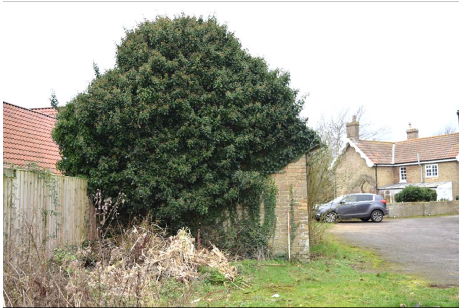
Plate 21 (shot 8): Southeast elevation largely covered by vegetation. Looking northwest, 1m scale
