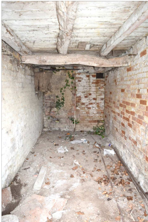
Plate 16 (shot 29): General view of storage space. Looking southwest, 1m scale
