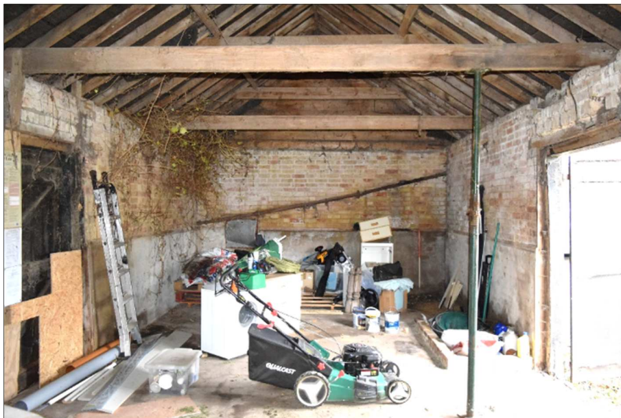
Plate 24 (shot 32): General view of the barn. Looking northwest, 1m scale
