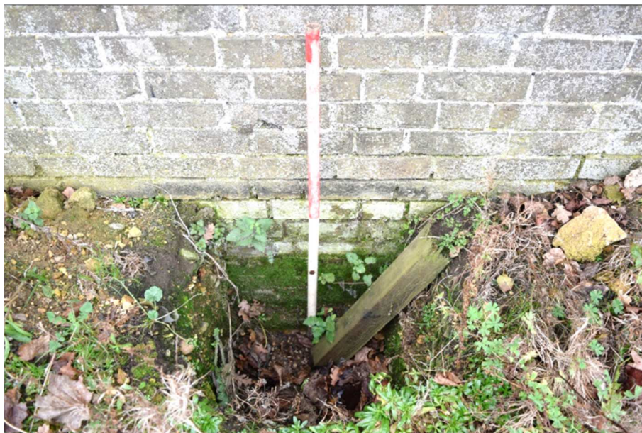
Plate 22 (shot 37): Inspection pit revealing stepped foundation. Looking southwest, 1m scale
