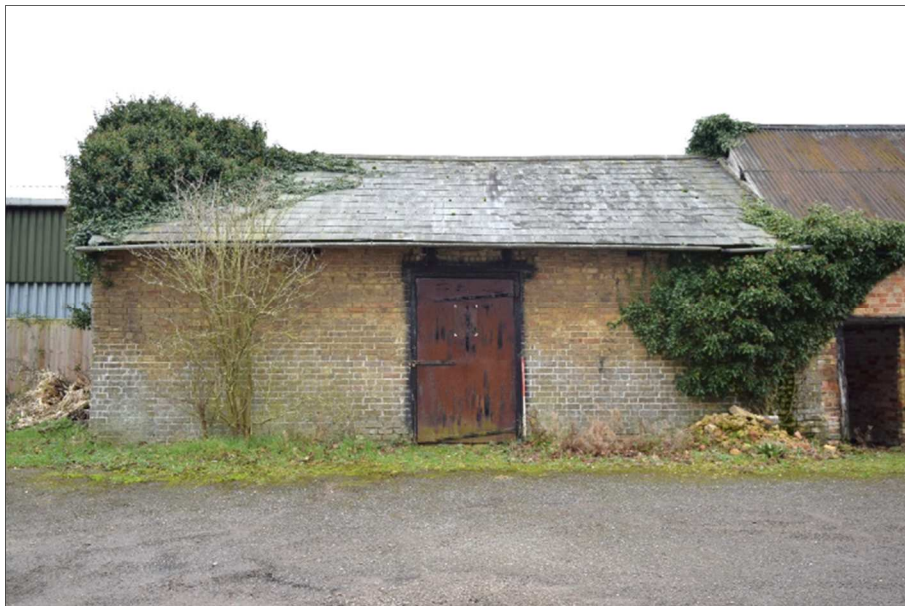
Plate 20 (shot 7): Northeast elevation. Looking southwest, 1m scale
