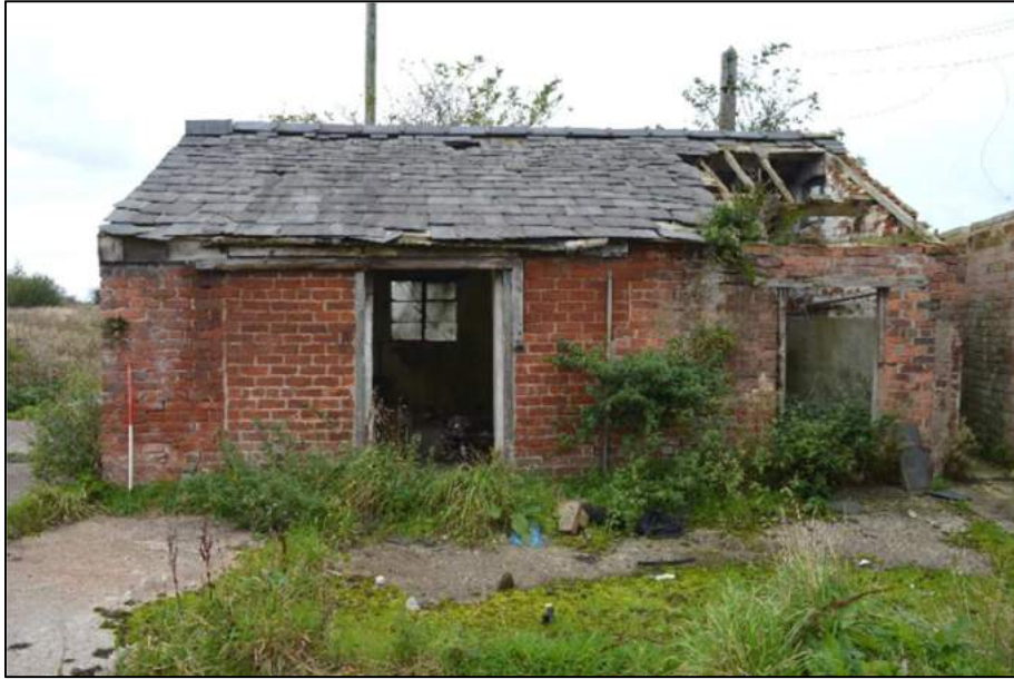
Plate 69: (Shot 214) Southeast elevation of Building G, looking northwest (1m scale)
