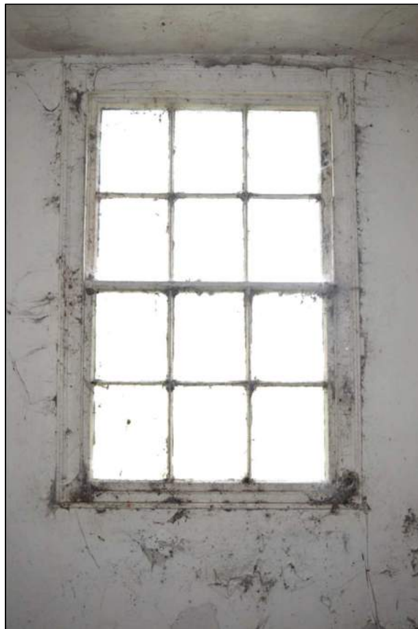
Plate 11: (Shot 134) Window to ground floor Room 2, Farmhouse A, looking north
