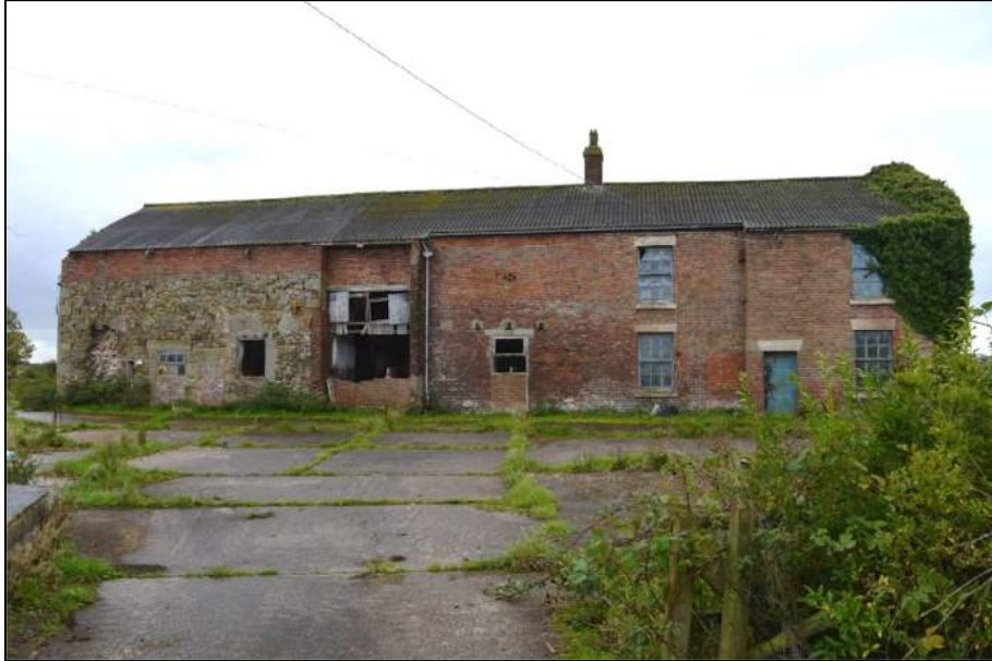
Plate 3: (Shot 2) North elevation of farmhouse A and barn B, looking south
