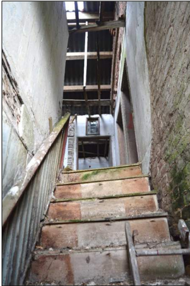
Plate 19: (Shot 165) View up the stairs in Farmhouse A, looking north
