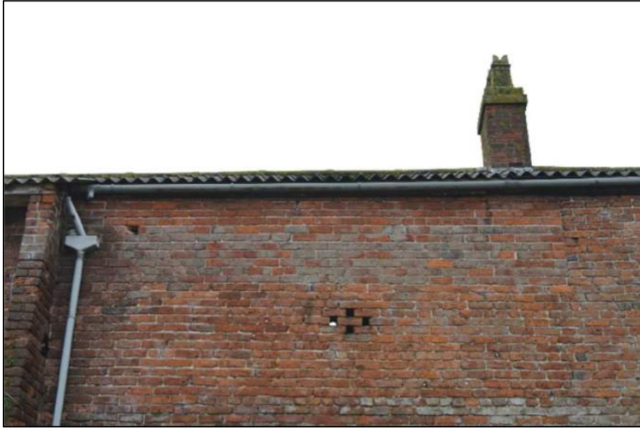
Plate 31: (Shot 20) Detail of north elevation of barn B showing ventilation holes, chimney of Farmhouse A and straight join high in wall between barn and farmhouse, looking south
