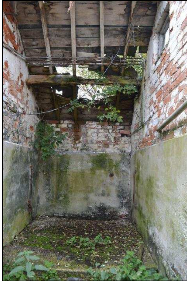
Plate 73: (Shot 228) Interior of Building G, Room 17, looking northwest
