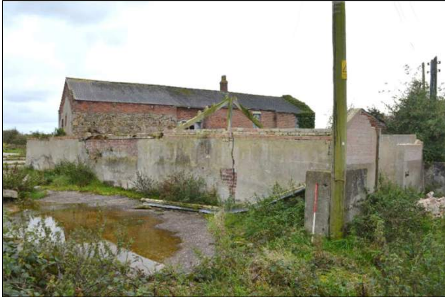
Plate 76: (Shot 238) Building H with Barn B and Farmhouse A in background, looking southwest (1m scale)
