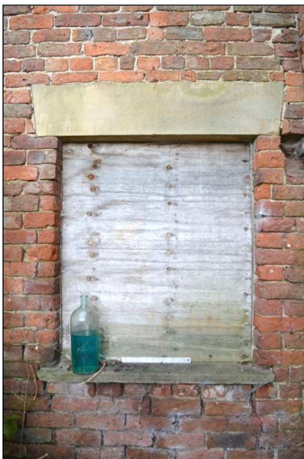
Plate 6: (Shot 91) Ground floor window to Room 13 in south elevation of Farmhouse A, looking north (0.30m scale)
