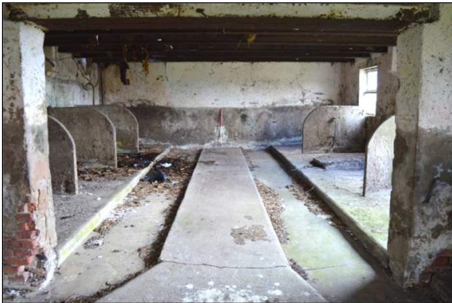
Plate 46: (Shot 114) Room 5, Barn B, looking west (1m scale)
