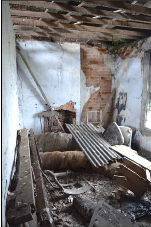
Plate 25: (Shot 181) First floor Room 8 of Farmhouse A, looking west towards chimneybreast
