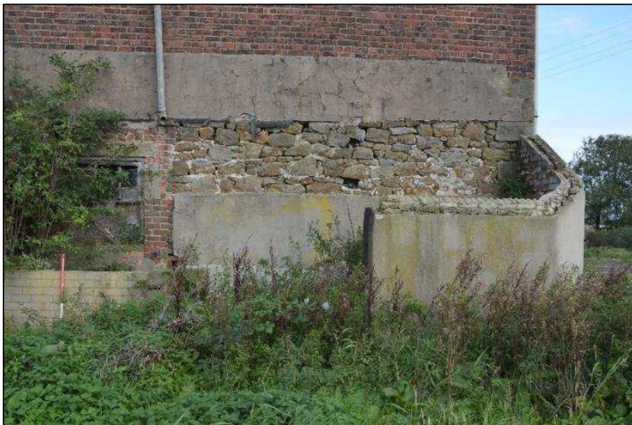
Plate 67: (Shot 56) Lean-to Building F, looking north (1m scale)
