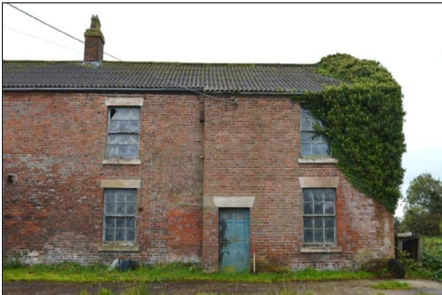
Plate 4: (Shot 4) North elevation of Farmhouse A, looking south (1m scale)
