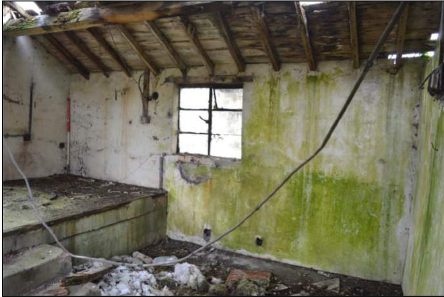
Plate 71: (Shot 219) Interior of Building G, Room 16, looking northwest (1m scale)
