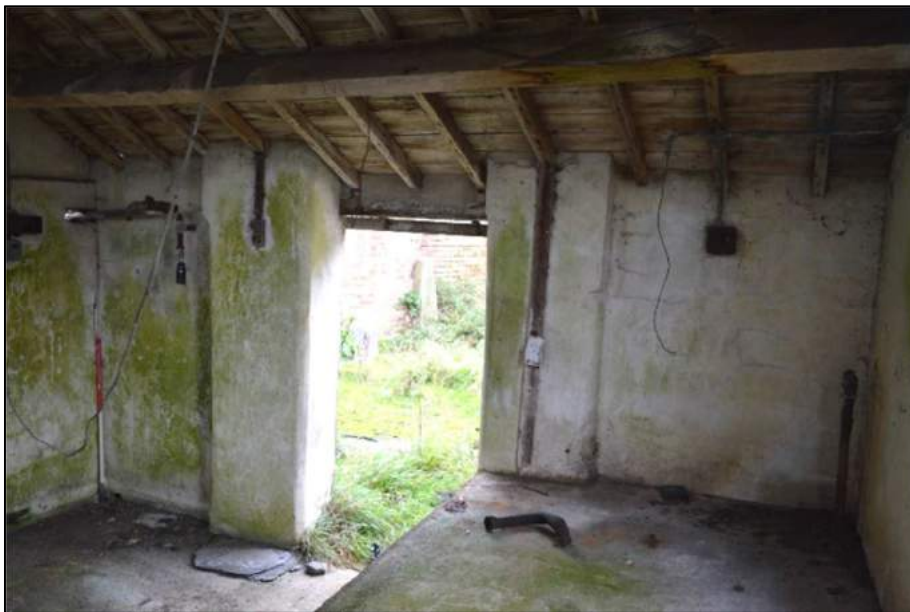
Plate 72: (Shot 217) Interior of Building G, Room 16, looking southeast (1m scale)
