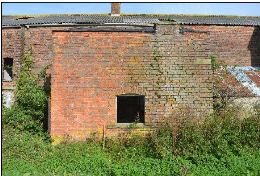
Plate 57: (Shot 71) South elevation of Building C, looking north (1m scale)
