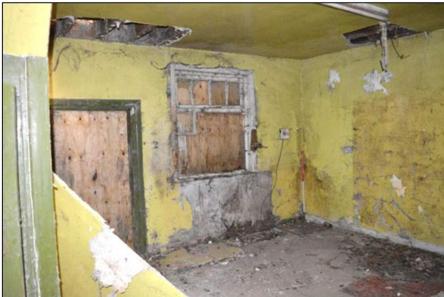
Plate 15: (Shot 158) Interior of Room 3 of Farmhouse A, looking southwest (1m scale)
