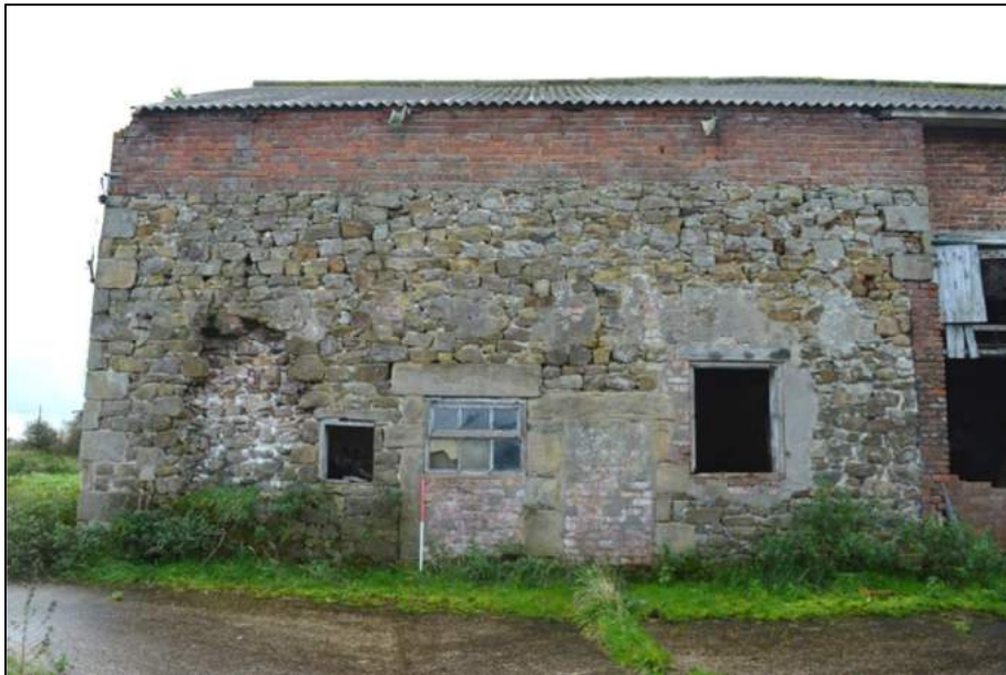
Plate 35: (Shot 26) North elevation of stone-built section of Barn B, looking south (1m scale)
