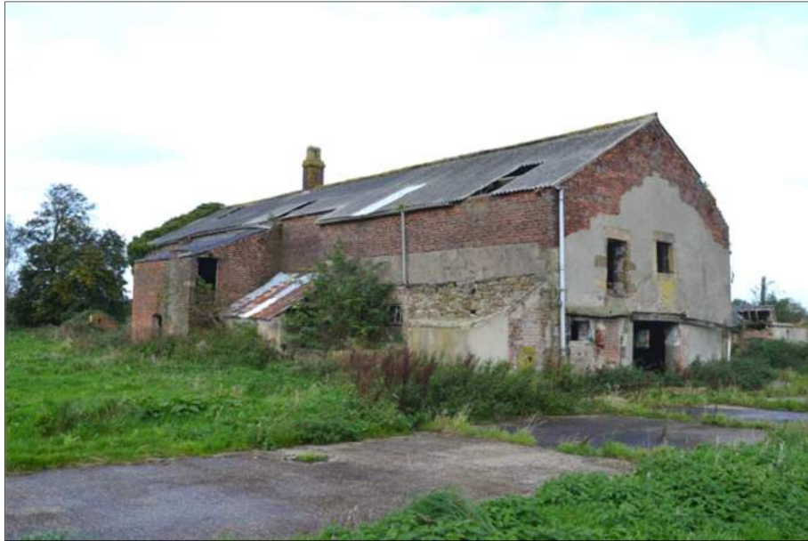
Plate 29: (Shot 46) General view of east and south elevations of Barn B with attached buildings A, C, D, E and F, looking northwest
