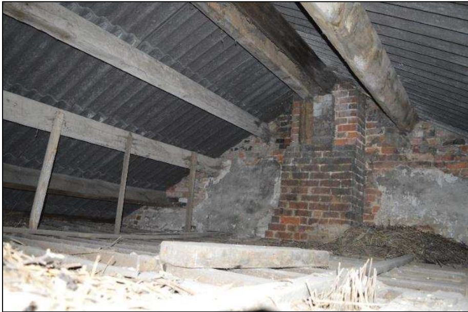
Plate 22: (Shot 174) View into roof space above Room 13, looking east
