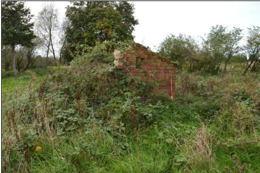
Plate 77: (Shot 244) Building I, looking northwest (1m scale)
