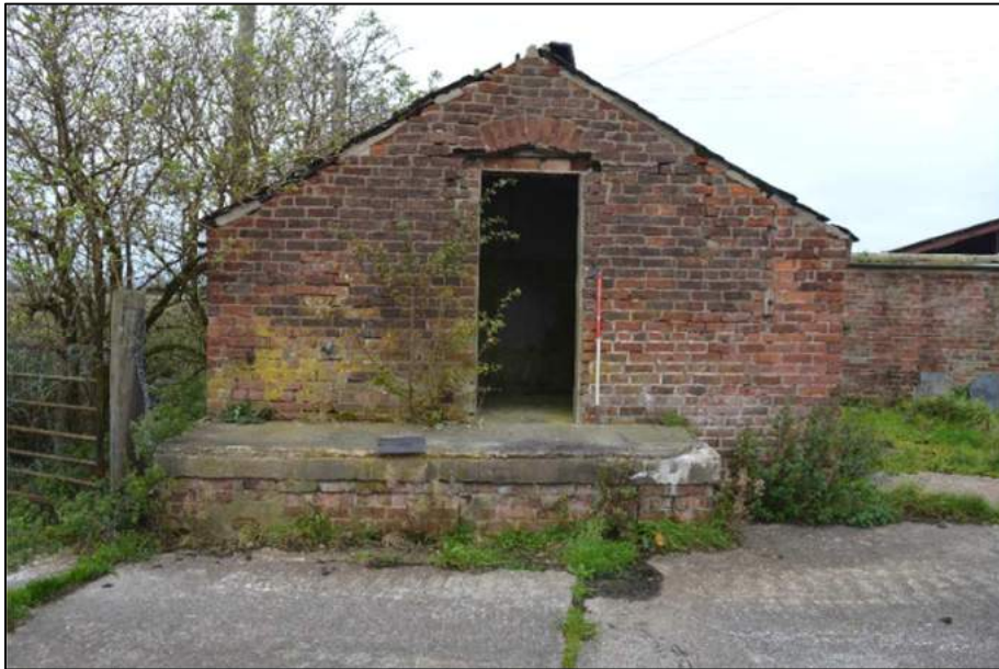
Plate 70: (Shot 226) Southwest gable of Building G, looking northeast (1m scale)
