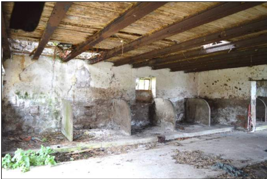
Plate 44: (Shot 105) Stalls in Room 6, Barn B, looking southwest (1m scale)
