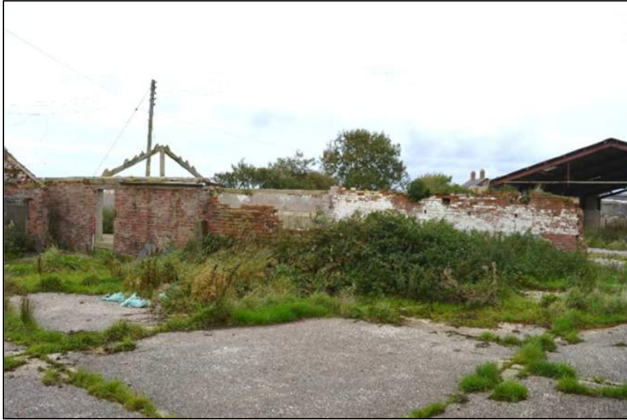
Plate 74: (Shot 231) Building H, looking northeast (1m scale)
