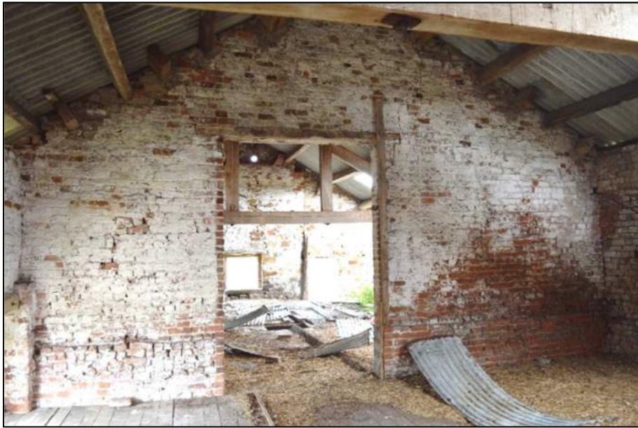
Plate 51: (Shot 203) Room 14 looking east to Room 15, first floor of Barn B
