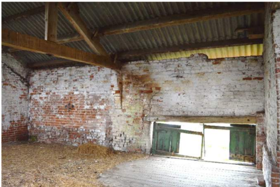
Plate 50: (Shot 198) Opening in north wall of Room 14, Barn B
