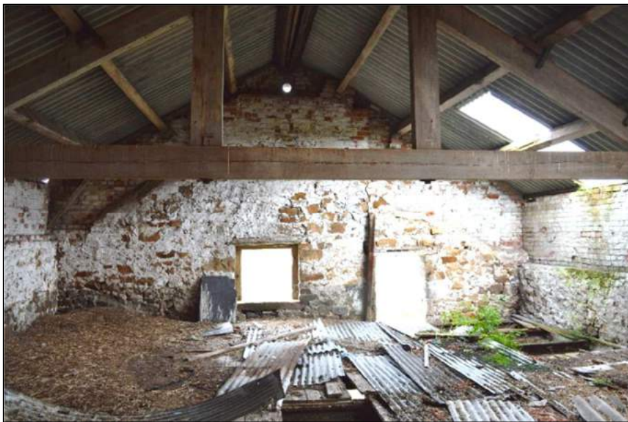
Plate 52: (Shot 204) Room 15, first floor of Barn B, looking east
